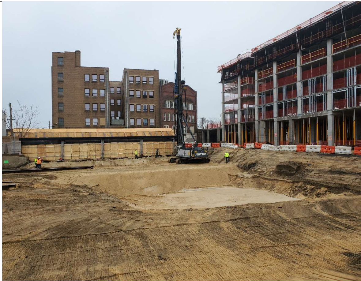
Photo 1- View of SOE drilling at building H1/H2.
