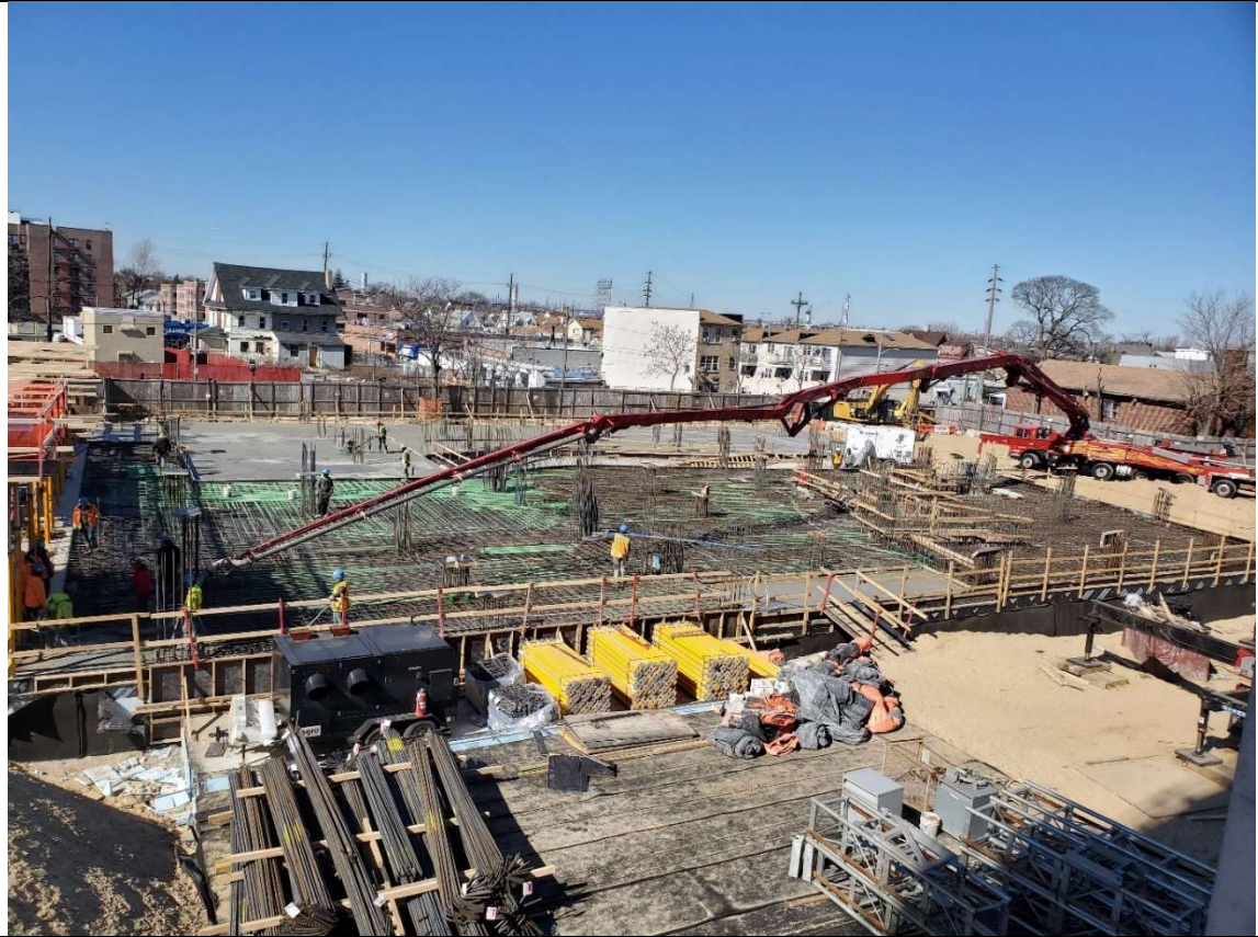
Photo 3- View of pouring concrete at building C grids A3, A4, B3, and B4.
