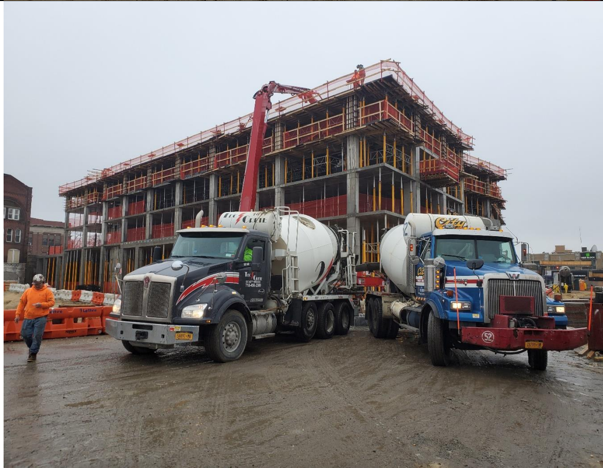
Photo 2- View of formwork rebar, and installation of concrete in grids C3, C4, D3, D4, and E4.
