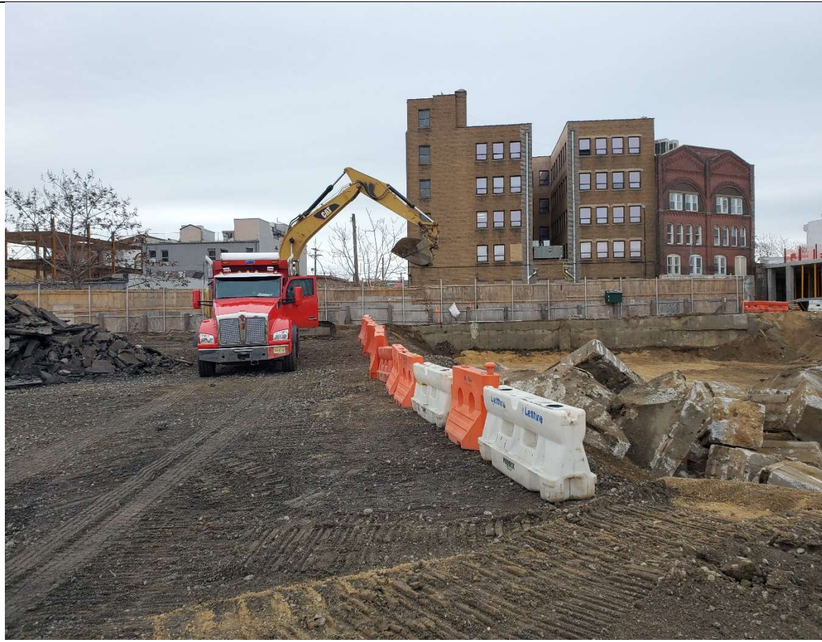
Photo 3- View of loading out soil in D6/E6 for export offsite.
