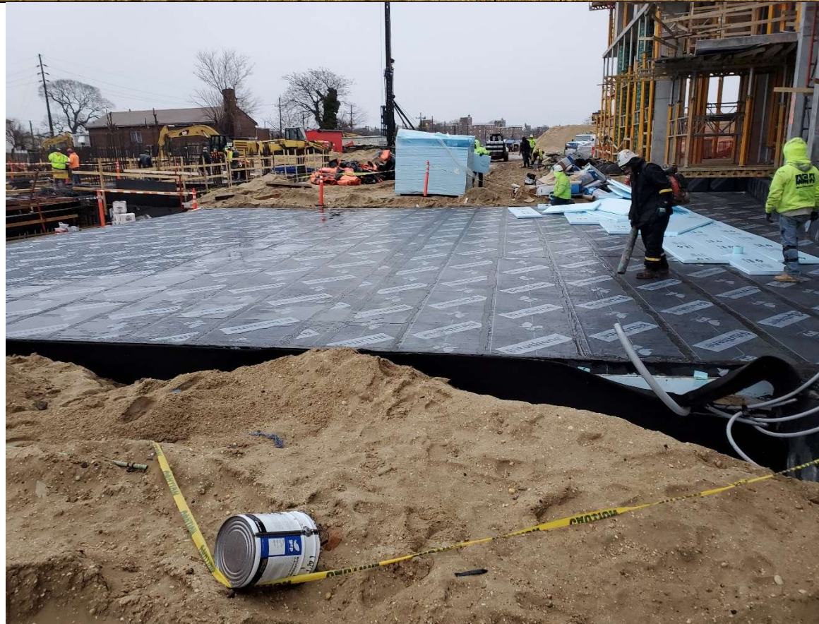
View of waterproofing installation in grids B3 and C3.
