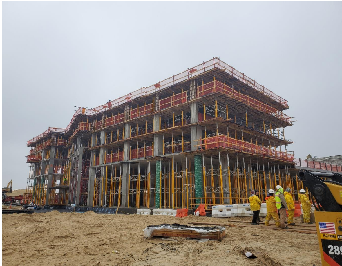
Photo 1- View of formwork and rebar installation in C2, C3, C4, D2, and D3.
