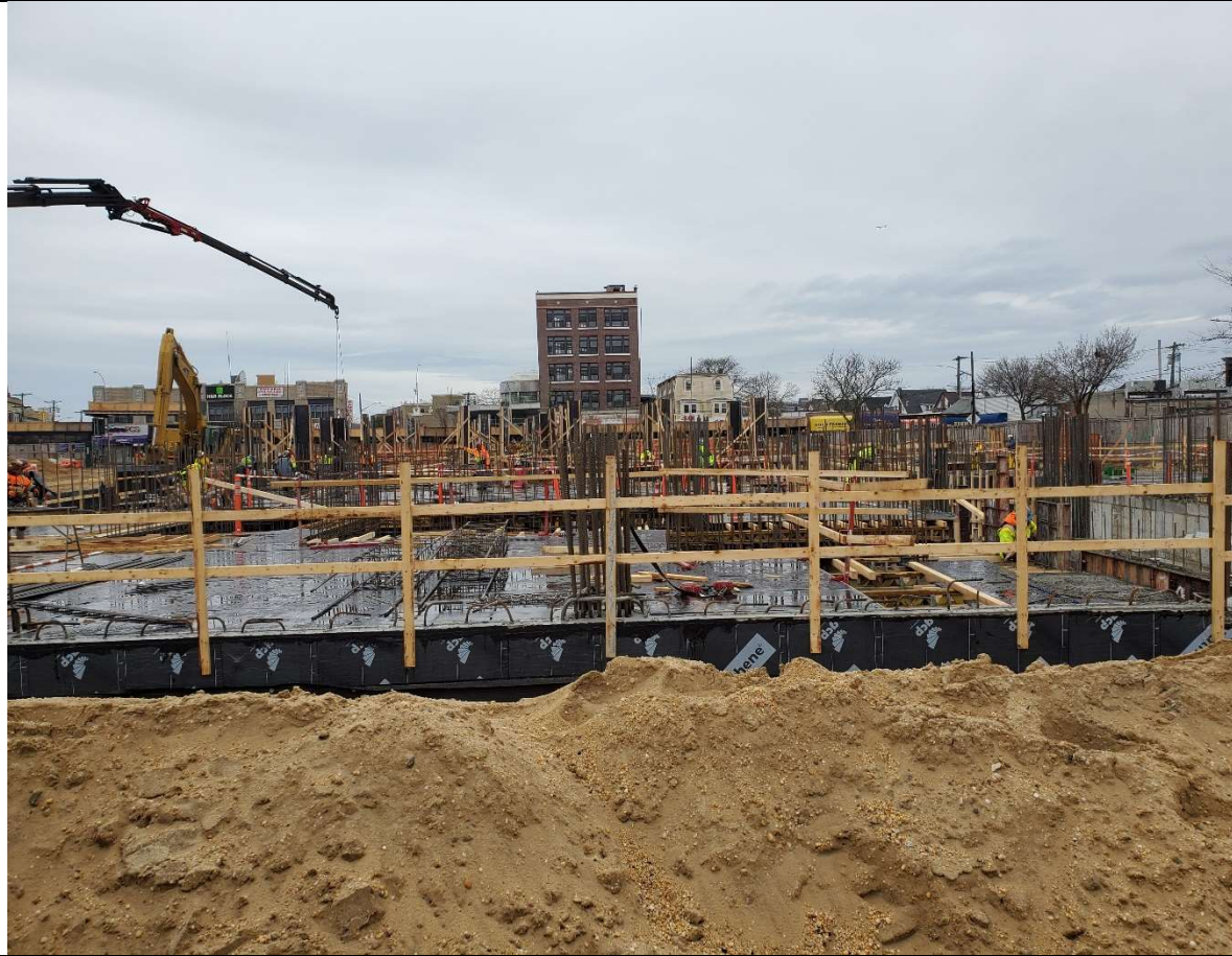
Photo 2- View of formwork and rebar installation in A3, A4, B3, and B4.
