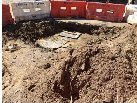
Photo 3- View of backfilling with clean fill in A5.
