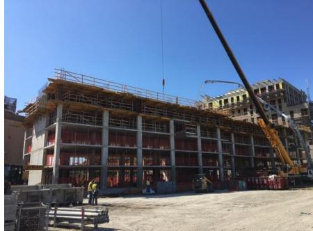
Photo 2- View of pouring concrete, rebar, utility, and formwork installation in A3, A4, B3, and B4.
