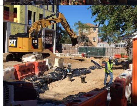
Photo 3- View of tamping down clean fill in A5.
