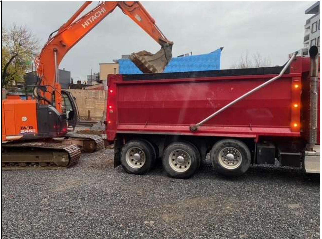
Photo 2 – View of the trucking of three loads of soil to Palmerton PA facility.
