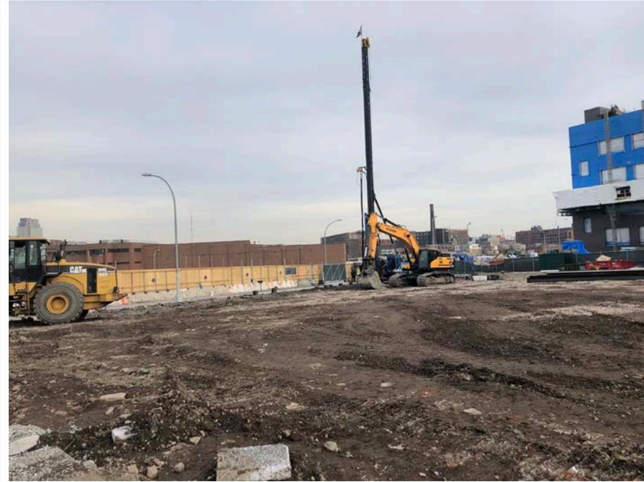
**Photo 3:** Looking southeast, American Pile and Foundation LLC driving piles in WCF-A1.
