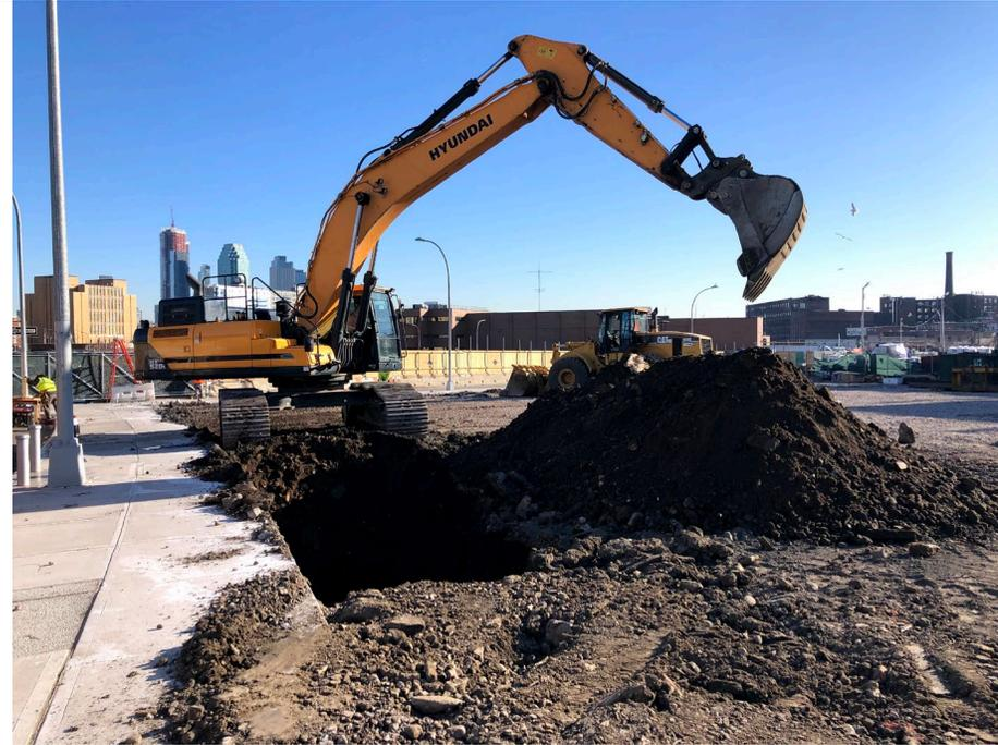
**Photo 3:** Looking northeast, New Leaf using excavator for pre-trenching activities in WCF-C3.
