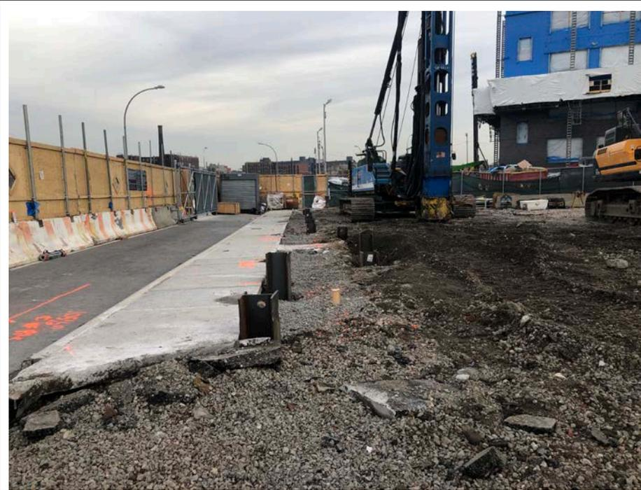
**Photo 4:** Looking southeast, site status of southeast portion of site including SOE piles in WCF-A2.
