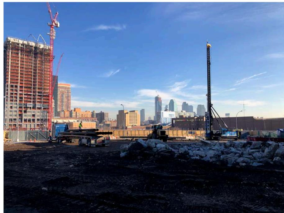
**Photo 2:** Looking north, site status of north portion of site including delivery of SOE piles.
