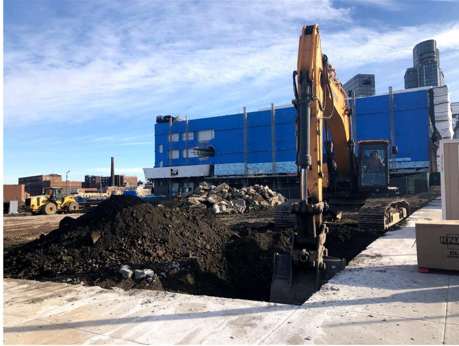
**Photo 1:** Looking southeast, New Leaf using excavator for pre-trenching activities in WCF-C3.
