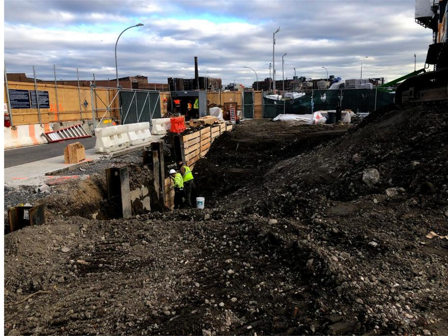
**Photo 3:** Looking east, New Leaf installing wood lagging between SOE piles.
