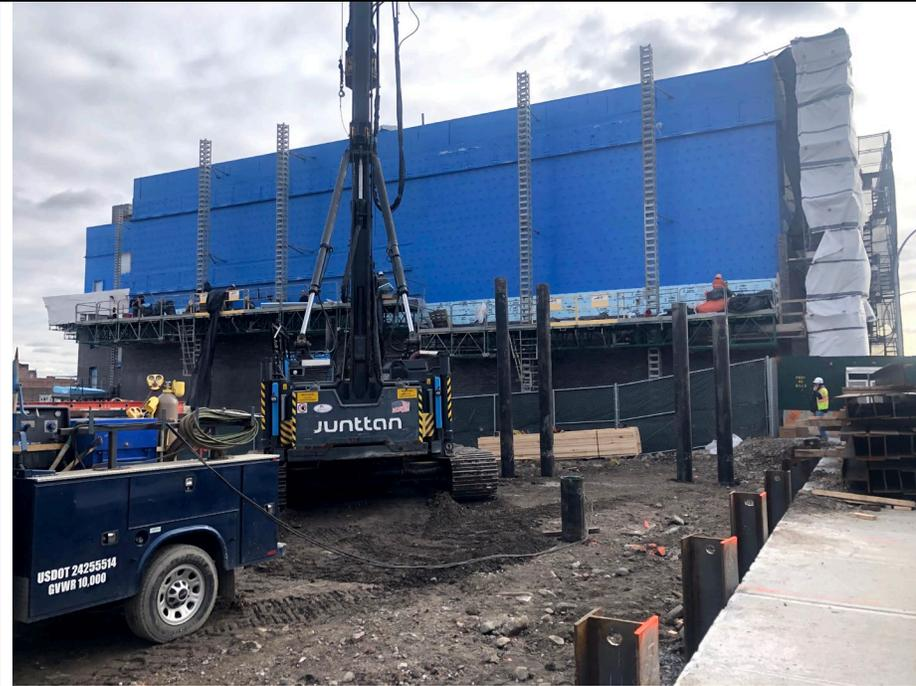
**Photo 1:** Looking southeast, American Pile and Foundation LLC driving index piles in WCF-C1.
