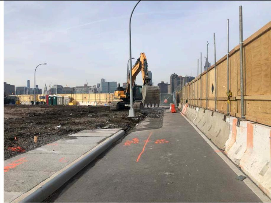
**Photo 1:** Looking southeast, New Leaf removing curb and trenching for SOE preclearing purposes in WCF-A2.
