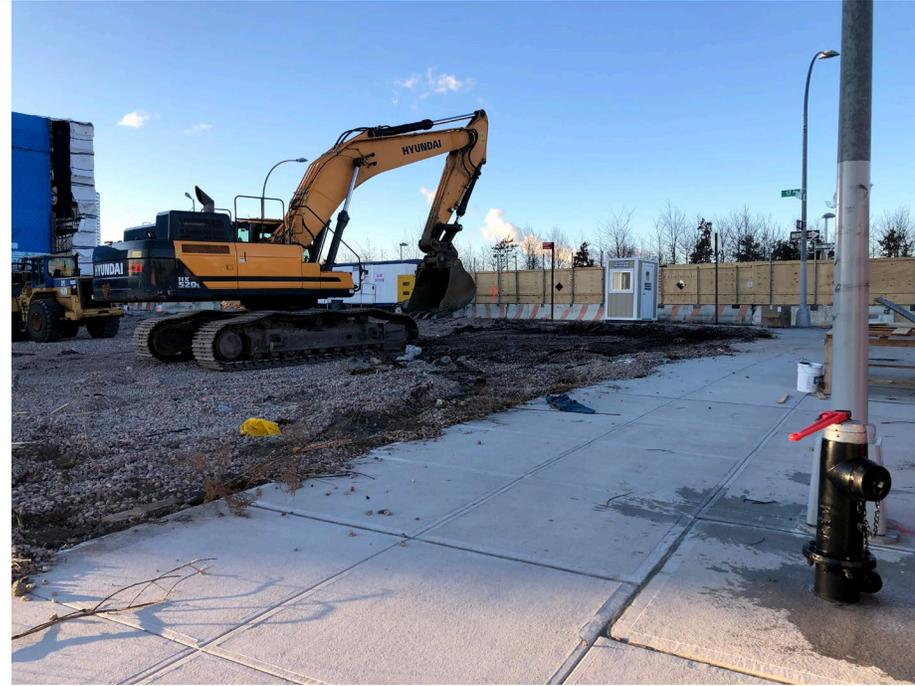
**Photo 1:** Looking south, New Leaf using excavator to grade RCA northeast in WCF-C3 in preparation for curb removal and trenching.
