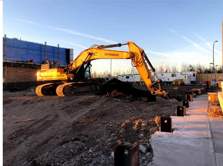
**Photo 3:** Looking south, New Leaf excavating in WCF-B3 prior to installing wood lagging.
