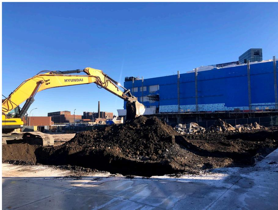
**Photo 2:** Looking southeast, New Leaf using excavator to trench in WCF-C3, identify any potential obstructions, and backfill in place.
