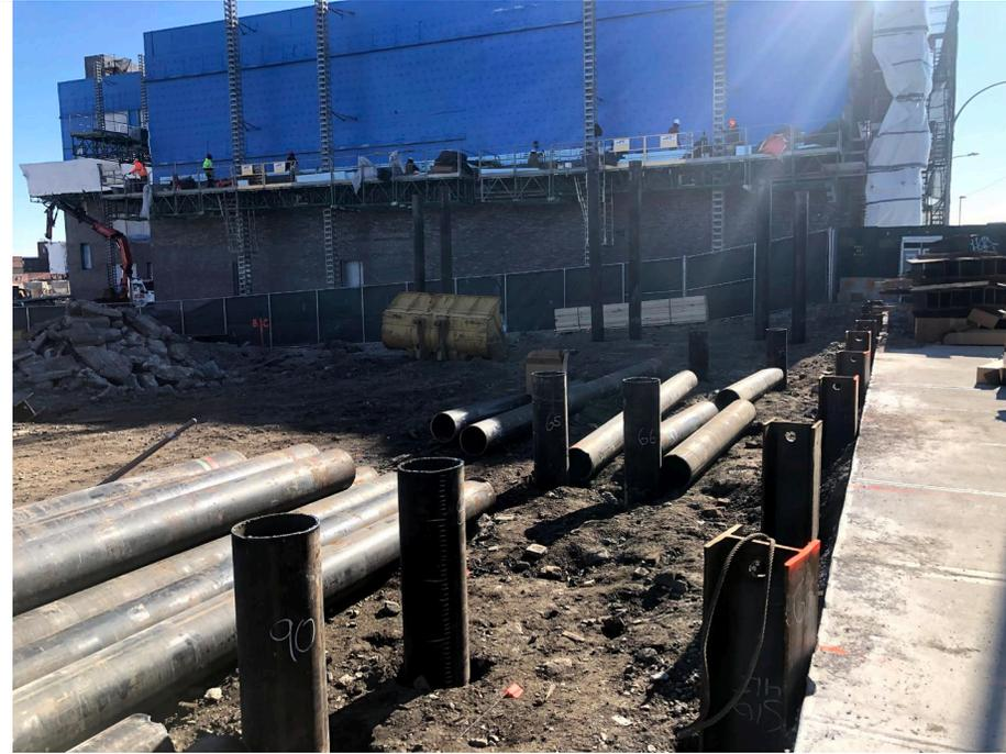
**Photo 1:** Looking southeast, grids WCF-C2 and WCF-C3 pile driving progress.
