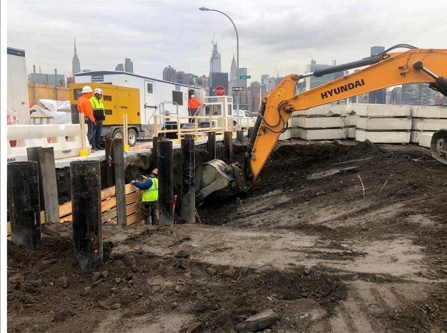
**Photo 1:** New Leaf installing wood lagging between SOE piles in WCF-C2.
