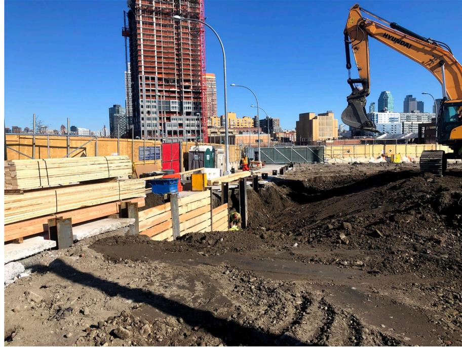
**Photo 3:** Looking east, New Leaf installing wood lagging between SOE piles in WCF-C3.
