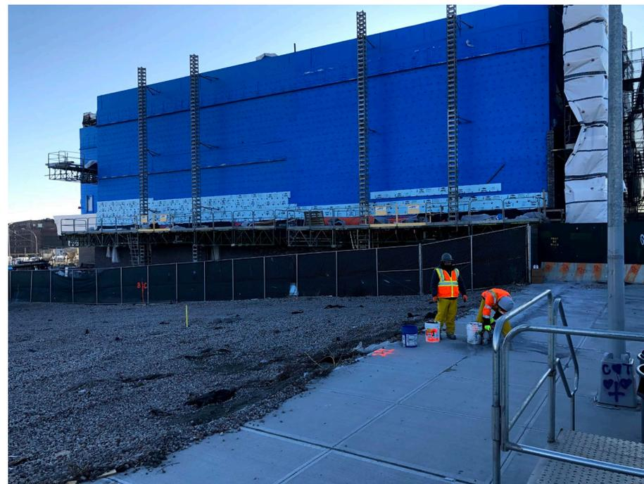
**Photo 2:** Looking southeast, New Leaf laborers using circular saw (with water for dust suppression) in preparation for curb removal.
