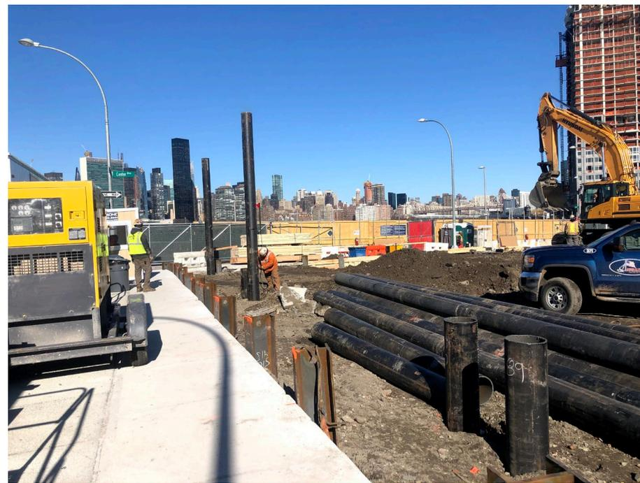
**Photo 2:** Looking north, American Pile and Foundation LLC cutting index piles in WCF-C3.
