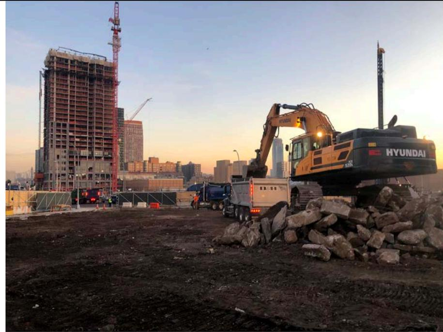
**Photo 1:** Looking north, New Leaf loading C&D from WCF-C2 into a dump truck for export.
