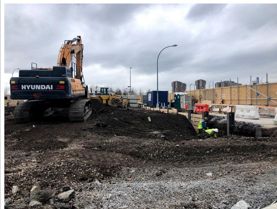
**Photo 2:** New Leaf installing wood lagging between SOE piles in WCF-B3.
