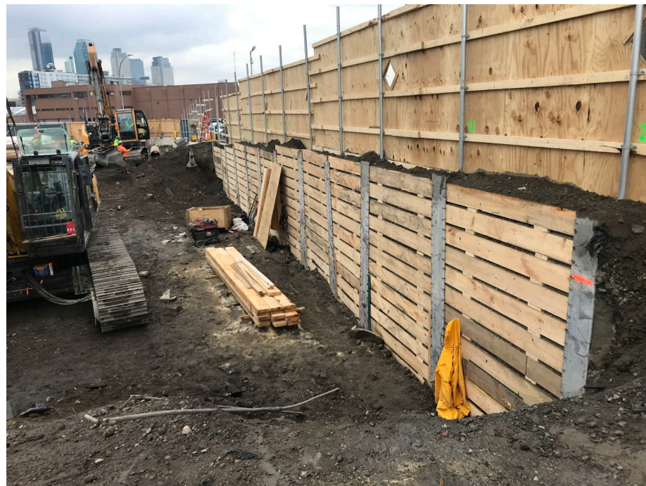
Photo 4: Looking east, New Leaf installing lagging in WCF-B1.
