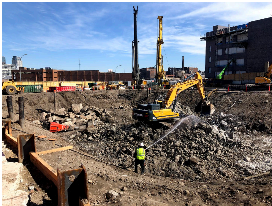
Photo 2: Looking southeast, New Leaf breaking up concrete with water used as dust suppression.
