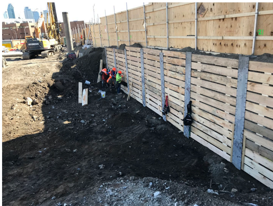
Photo 4: Looking east, New Leaf installing lagging in WCF-C1.
