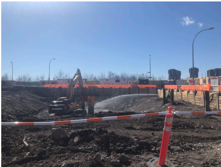
Photo 4: Looking southwest, New Leaf breaking up concrete in WCF-B2 with water used as dust suppression.
