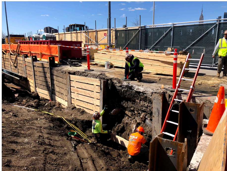
Photo 2: Looking northwest, New Leaf lagging in WCF-B3.
