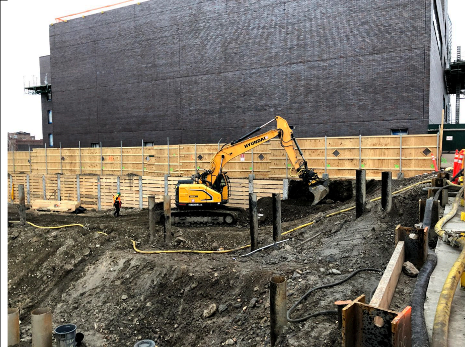
Photo 3: Looking southeast, New Leaf excavating in WCF-C1 for shoring purposes.
