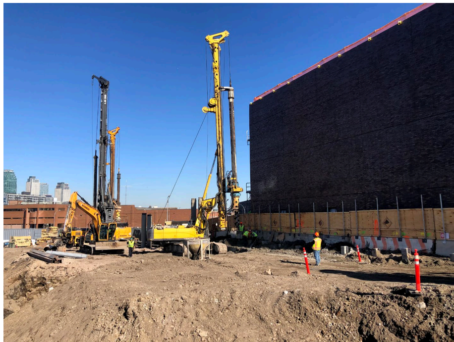
Photo 4: Looking east, New Leaf preapring to drill soldier piles in WCF-B1 towards the end of the work-day.
