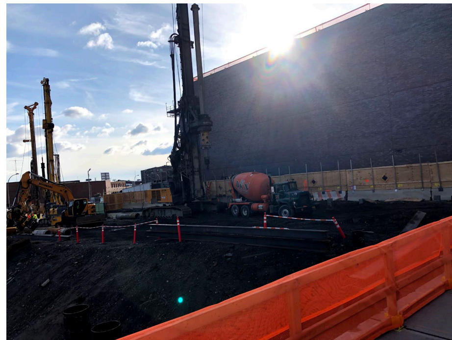
Photo 2: Looking southeast, New Leaf preapring to drill soldier piles and pour concrete in WCF-C1.
