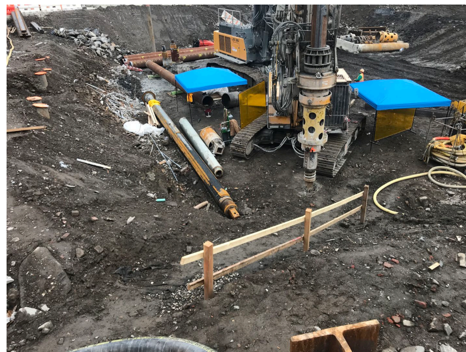
Photo 2: New Leaf continues drilling rat holes in WCF-B3 for future cassion piles.
