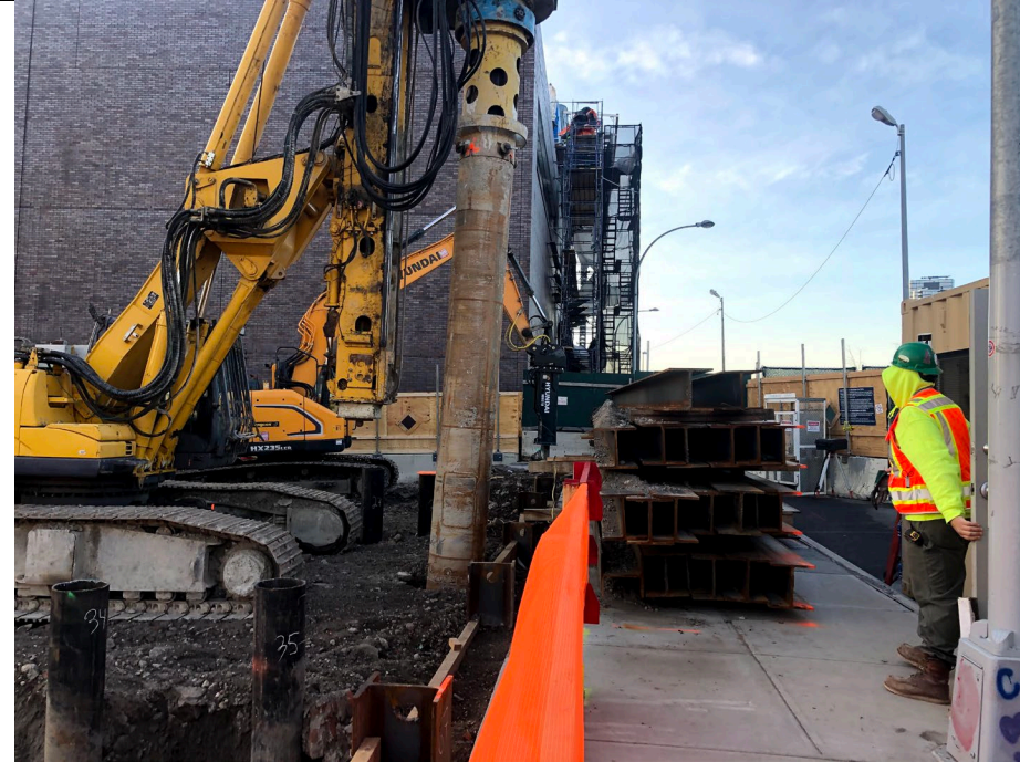
Photo 3: Looking southeast, New Leaf soldier pile drilling in WCF-C1.
