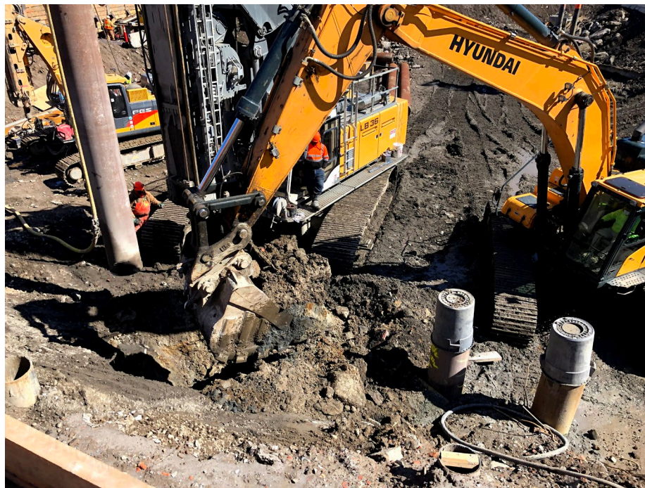
Photo 4: Looking east, New Leaf excavating for drilling preclearing purposes in WCF-C2 .
