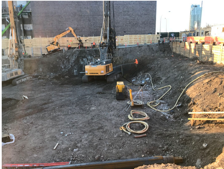
Photo 2: Looking southeast, overview of western portion of site during drilling activities – water is being used for dust suppression.
