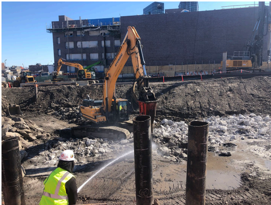
Photo 2: Looking southeast, New Leaf breaking up concrete in WCF-B2 with water used as dust suppression.
