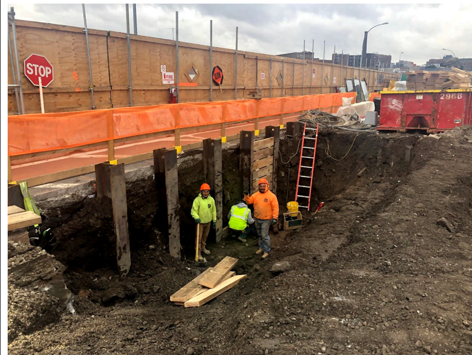
Photo 2: Looking east, New Leaf lagging in WCF-A2.
