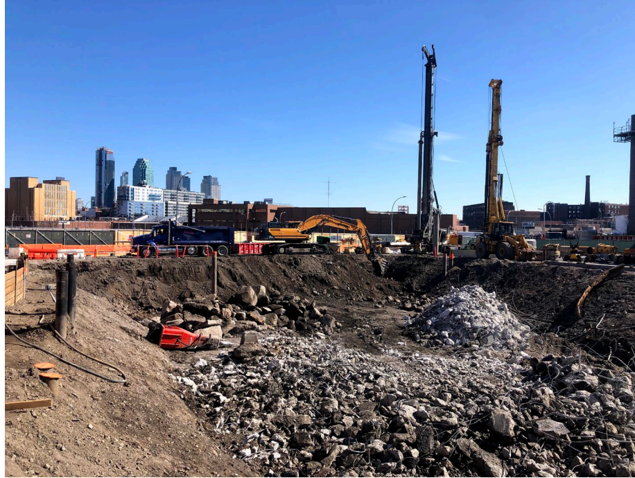
Photo 1: Looking northeast, New Leaf excavating and loading dump truck with soil from WCF-A2 (0-6).
