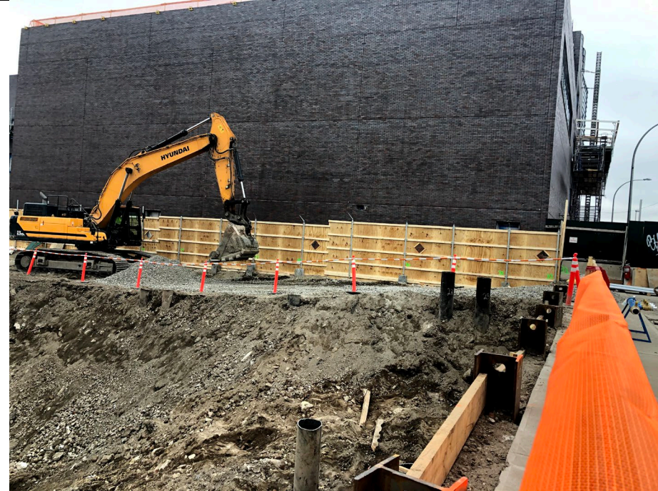
Photo 3: Looking southeast, New Leaf spreading gravel along temporary roadway in WCF-C1.
