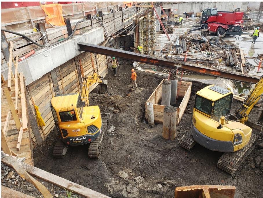
**Photo 4:** View of the southwest portion of the Site including foundation wall and soil excavation/exportation progress.
