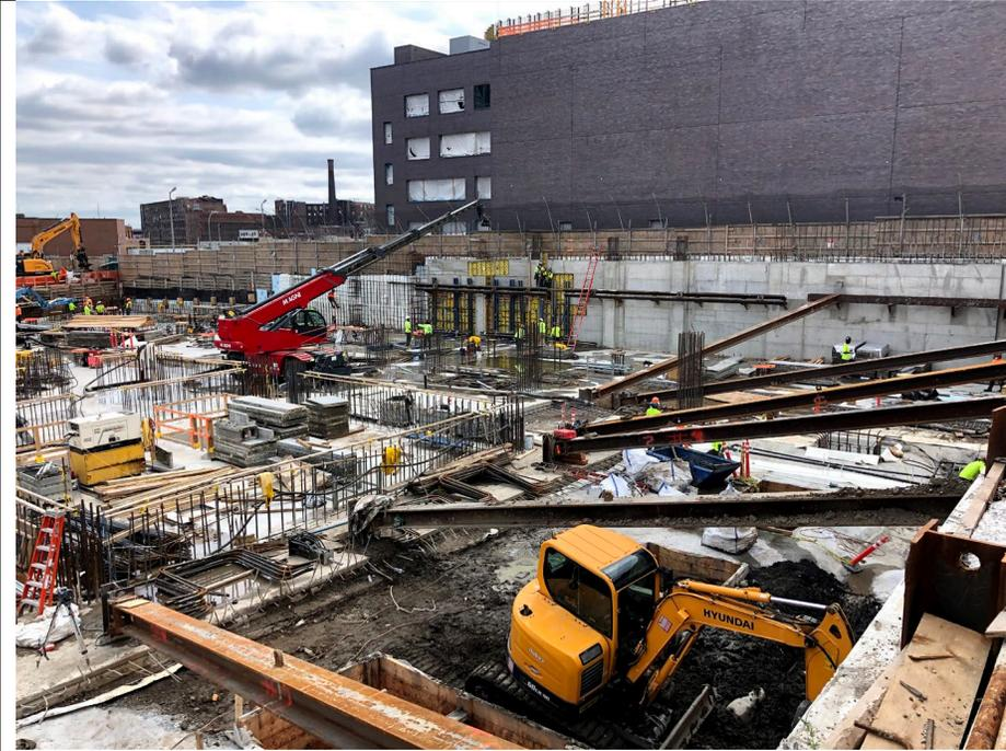
**Photo 3:** Looking southeast, New Leaf removing foundation wall forms in WCF-B1.
