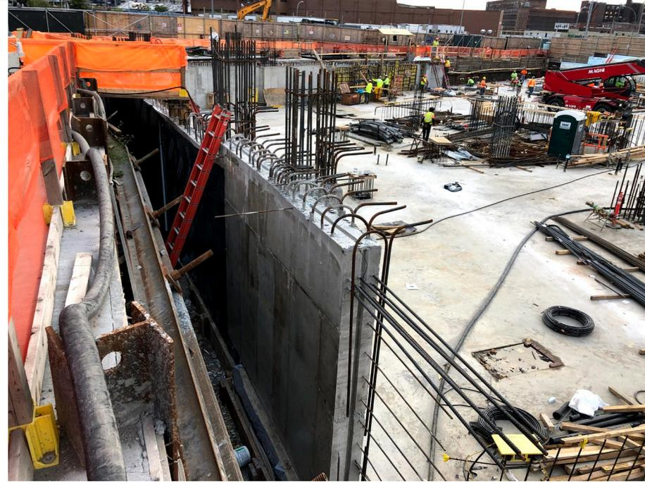
**Photo 3:** View of waterproofing progress on the foundation wall along the northwest perimeter of the Site.
