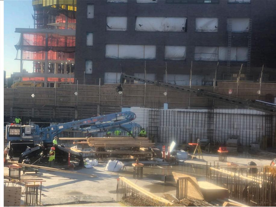
**Photo 3:** Looking South, view of New Leaf bending/latching rebar, laying/removing formwork, and installing waterproofing/insulation for cellar foundation walls.
