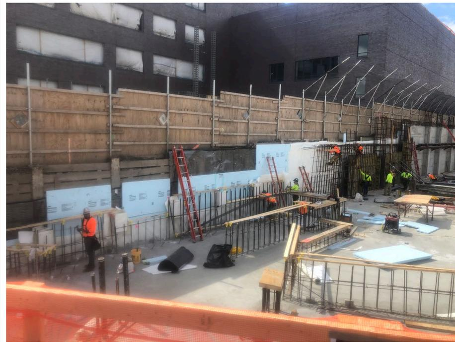
**Photo 4:** Looking south, additional view of New Leaf bending/latching rebar, laying/removing formwork, and installing waterproofing/insulation for cellar foundation walls.
