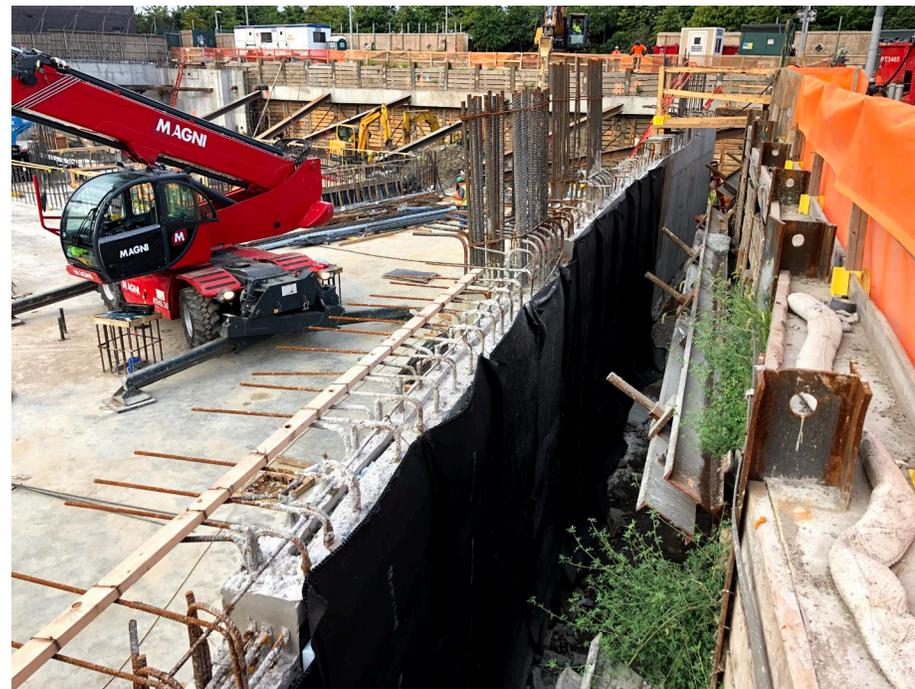
**Photo 4:** View of waterproofing progress along the outer side of the foundation wall in WCF-C3/B3.
