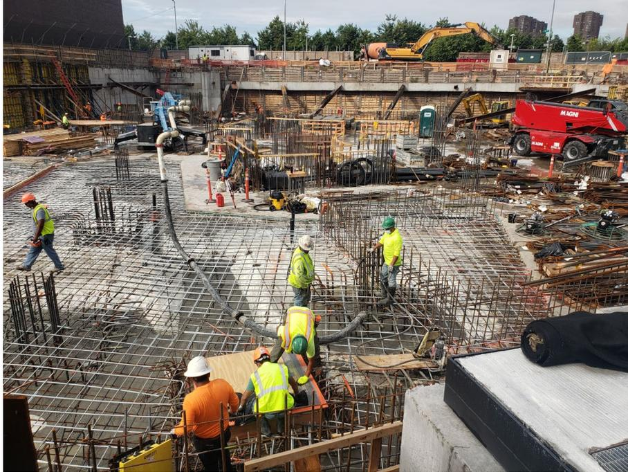
**Photo 3:** Looking southeast, view of New Leaf pouring concrete in WCF-A2 portion of rebar and waterproofing layout.
