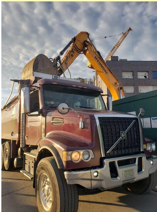
**Photo 2:** Looking southeast, a view of New Leaf loading soils from WCF-A1 for export to Clean Earth waste facility.
