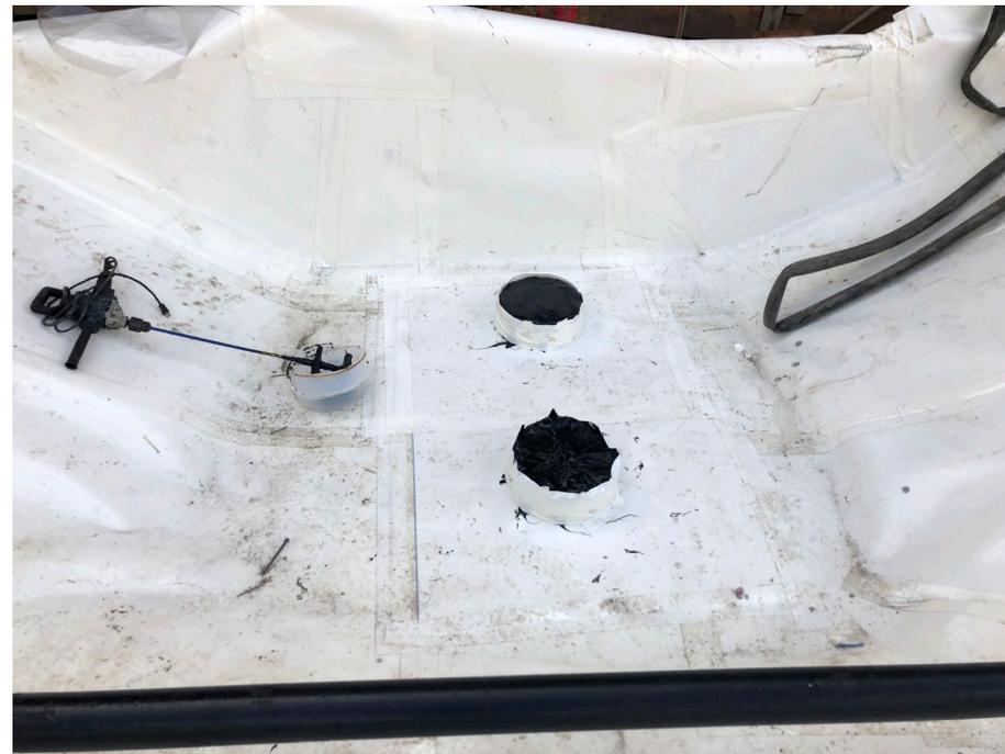
**Photo 2:** View of waterproofing and liquid membrane around protrusions.
