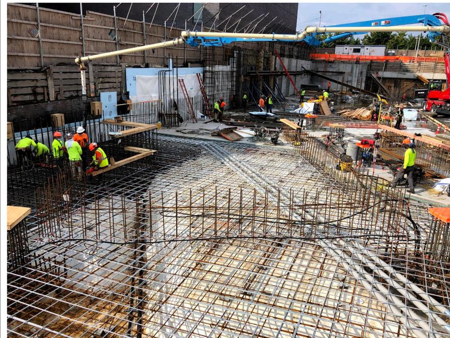
**Photo 4:** Looking south, New Leaf pumping concrete into WCF-A1 for foundation slab.
