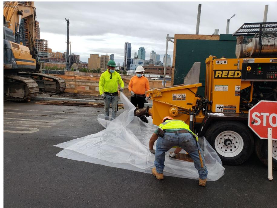
**Photo 2:** Looking northwest, view of New Leaf placing poly-sheeting in preparation for concrete mixing activities.
