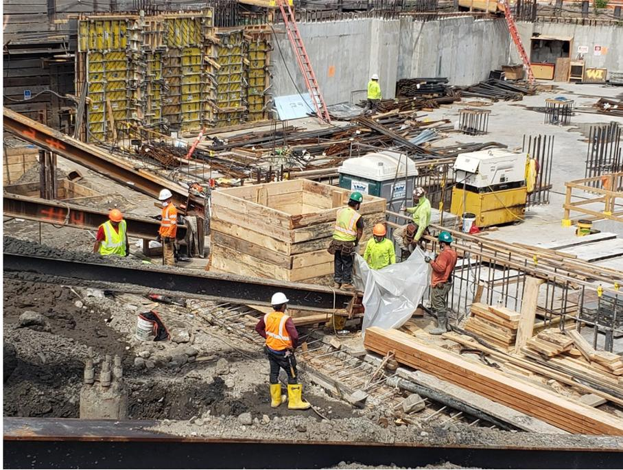
**Photo 1:** Looking north, view of New Leaf prefabricating wooden shoring structures to be installed during pile cap construction.
