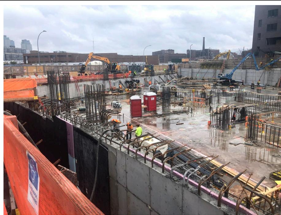
**Photo 4:** Looking east, view of Site status and waterproofing progress along the northwest foundation wall.
