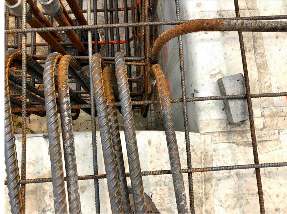
**Photo 3:** View of waterproofing and rebar around the edges of a pile cap.
