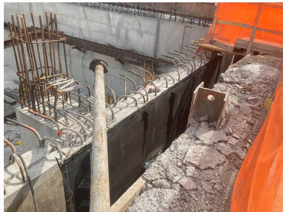
**Photo 4:** Looking east, New Leaf continues waterproofing installation on foundation wall in grid WCF-C1.
