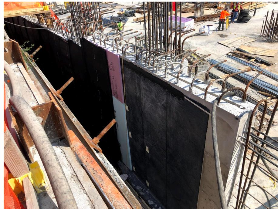
**Photo 4:** View of vapor barrier along the northwest foundation wall.
