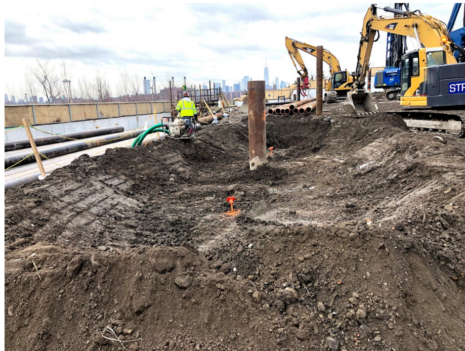
Photo 4: Looking west, site status of southwest portion of site.
