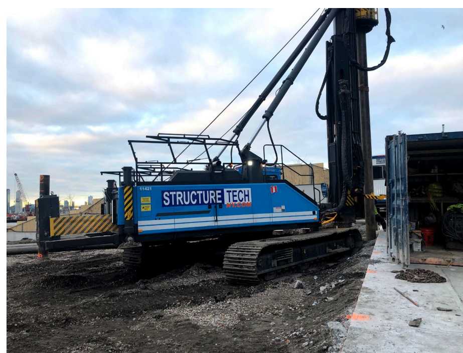
Photo 1: Looking southwest, StructureTech drilling index piles in WCG-3.
