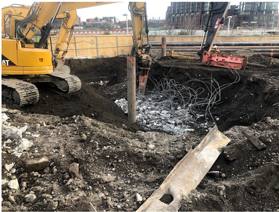
Photo 4: Looking east, StructureTech breaking up concrete slab below grade in WCG-4.
