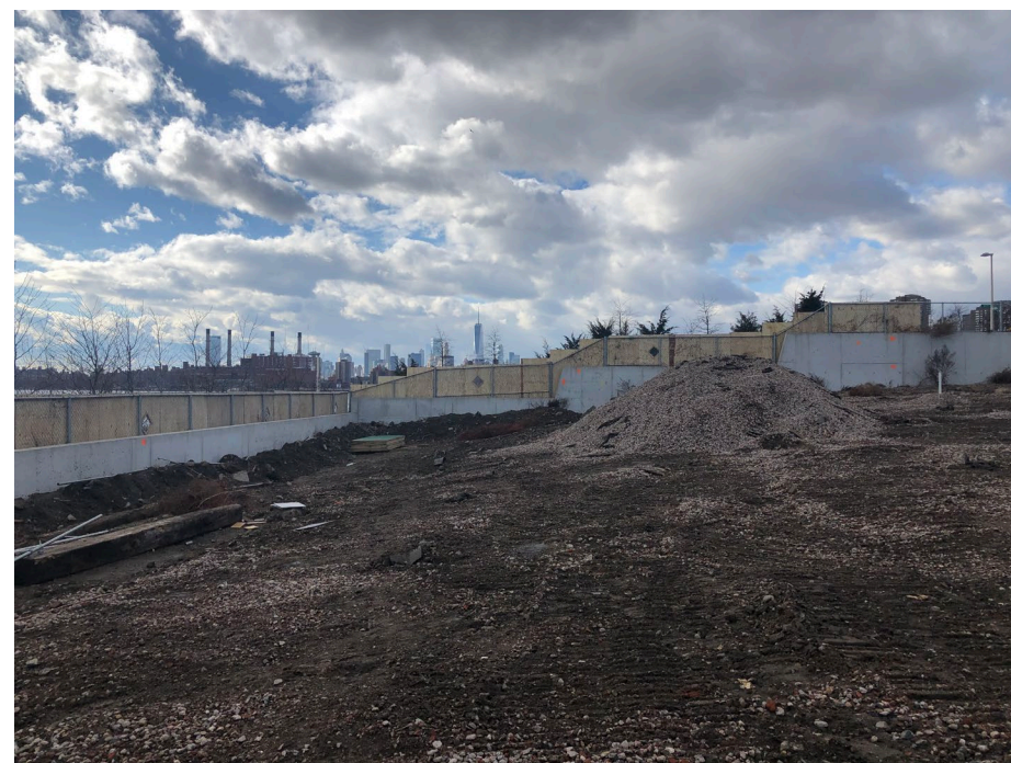
Photo 2: Looking west, site status of the southwest area of the site.
