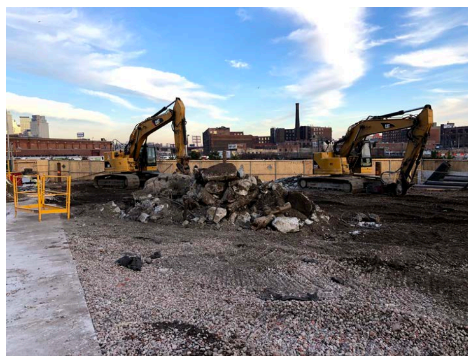
Photo 1: Looking east, StructureTech preclearing for index pile driving in WCG-4.
