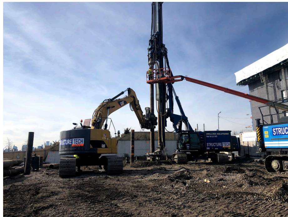
Photo 1: Looking southwest, StructureTech drilling index piles in WCG-3.
