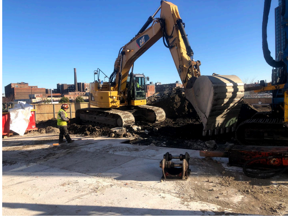
Photo 3: Looking southeast, StructureTech removing curb in WCG-1.
