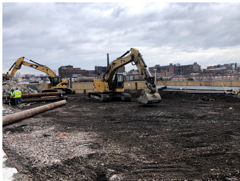
Photo 2: Looking east, StructureTech grading in WCG-4.
