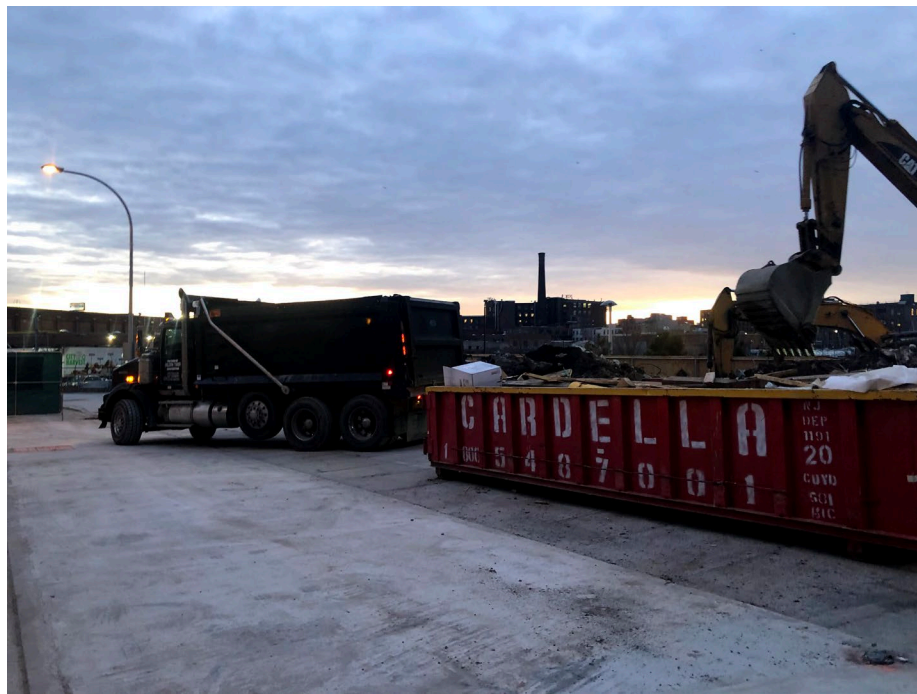
Photo 1: Looking northeast, StructureTech loading C&D into dump truck for export.
