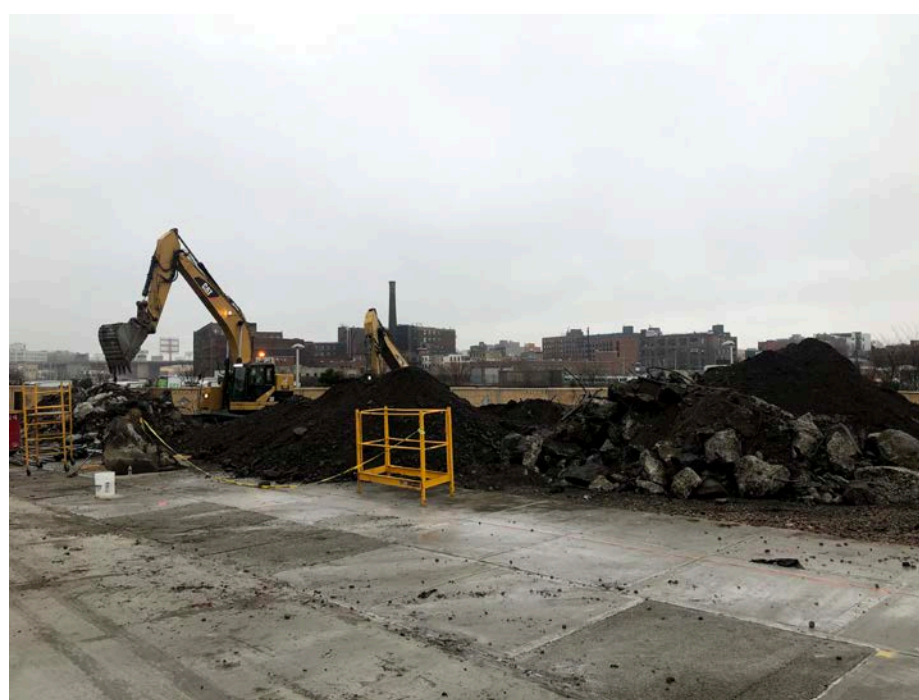
Photo 2: Looking southeast, site status of the southeast portion of site.
