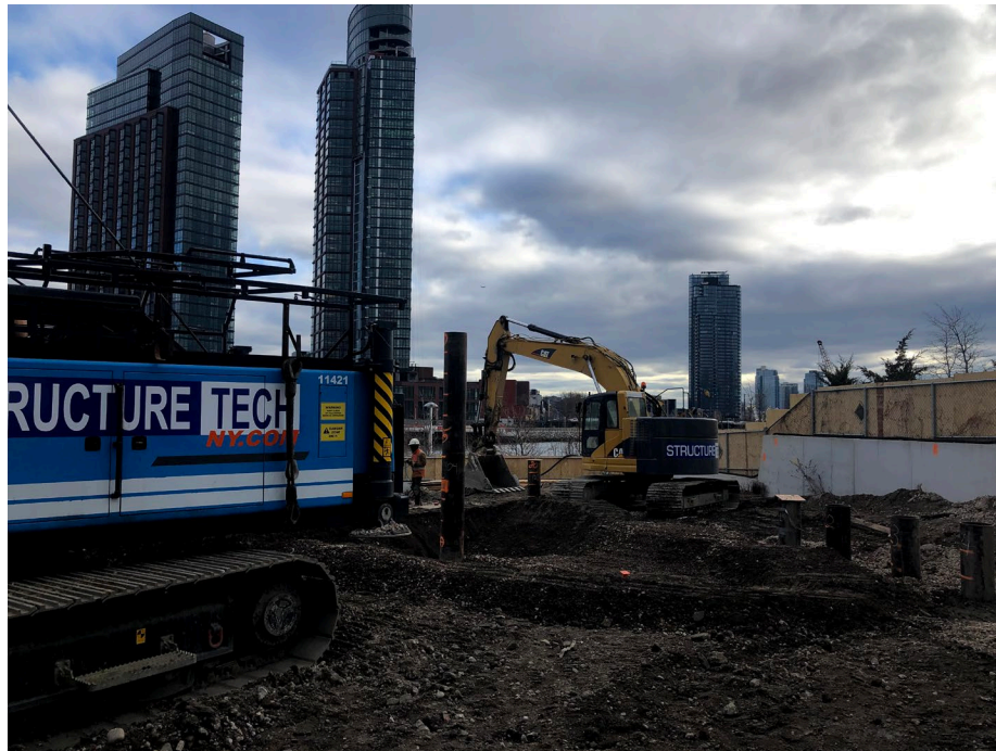
Photo 4: Site grading and pile driving continues in WCG-3.
