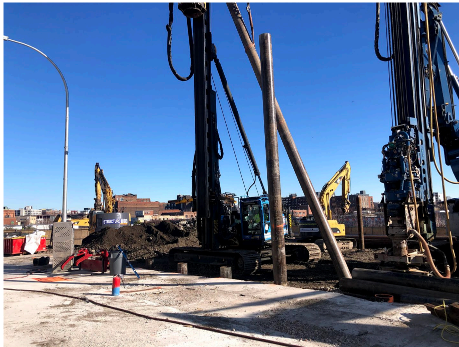
Photo 2: Looking east, StructureTech drilling index piles in WCG-2.
