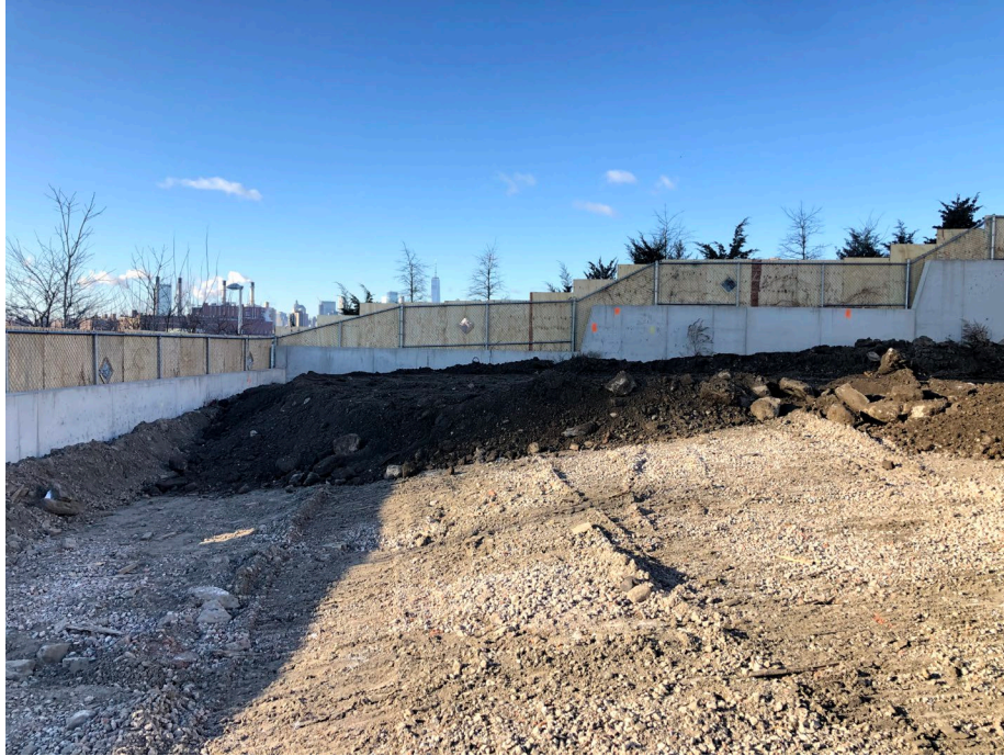
Photo 3: Looking west, site status of the southwest area of the site.
