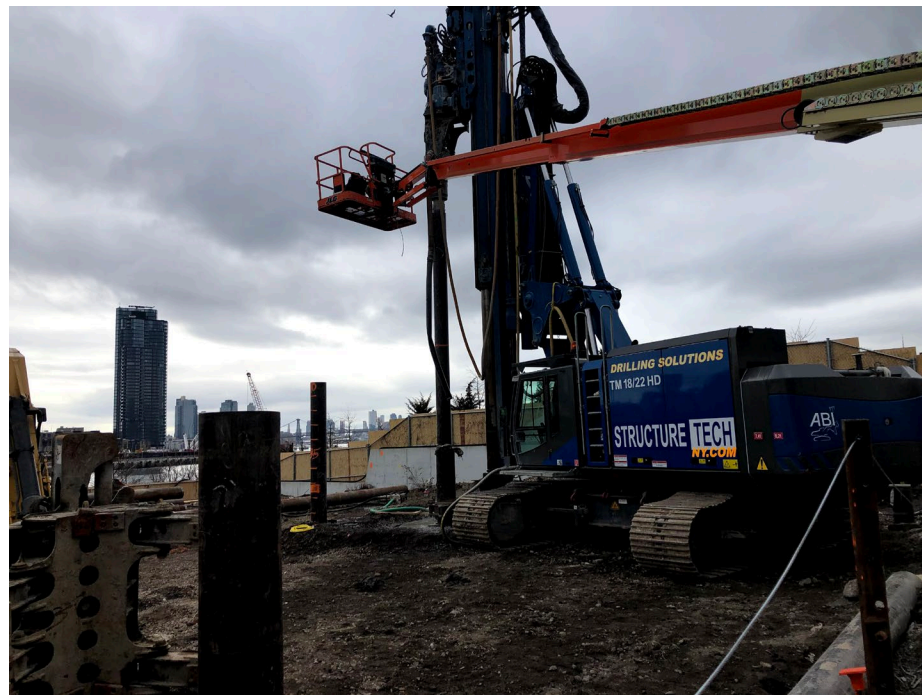
Photo 4: Looking south, StructureTech drilling in WCG-3.
