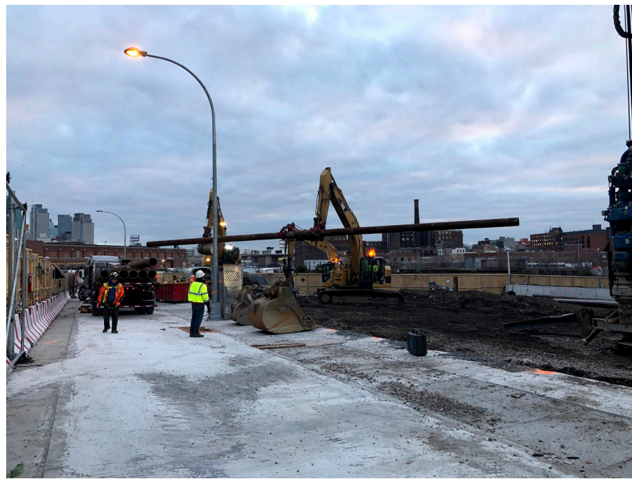
Photo 3: Looking east, StructureTech unloading delivery of index piles.
