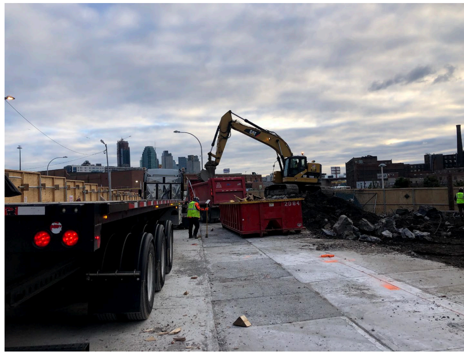
Photo 4: Looking northeast, StructureTech loading C&D into truck for export.
