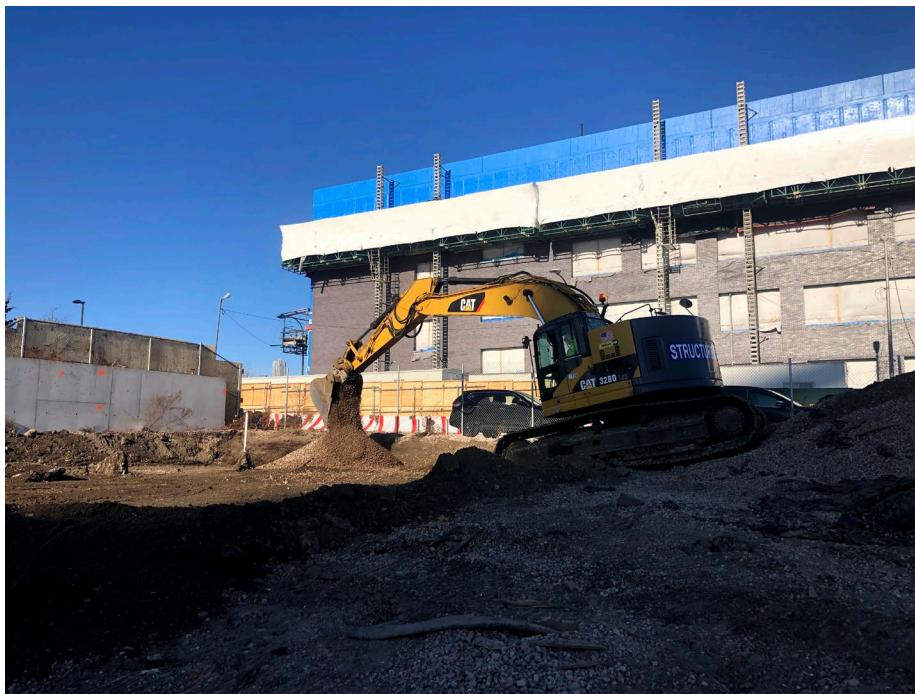
Photo 4: StructureTech moving RCA stockpile from WCG-2 to WCG-3.
