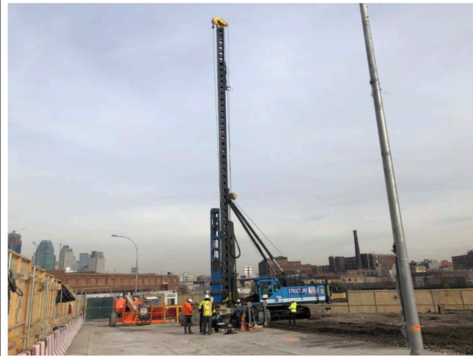
Photo 4: Looking northeast, StructureTech index pilling in WCG-4.
