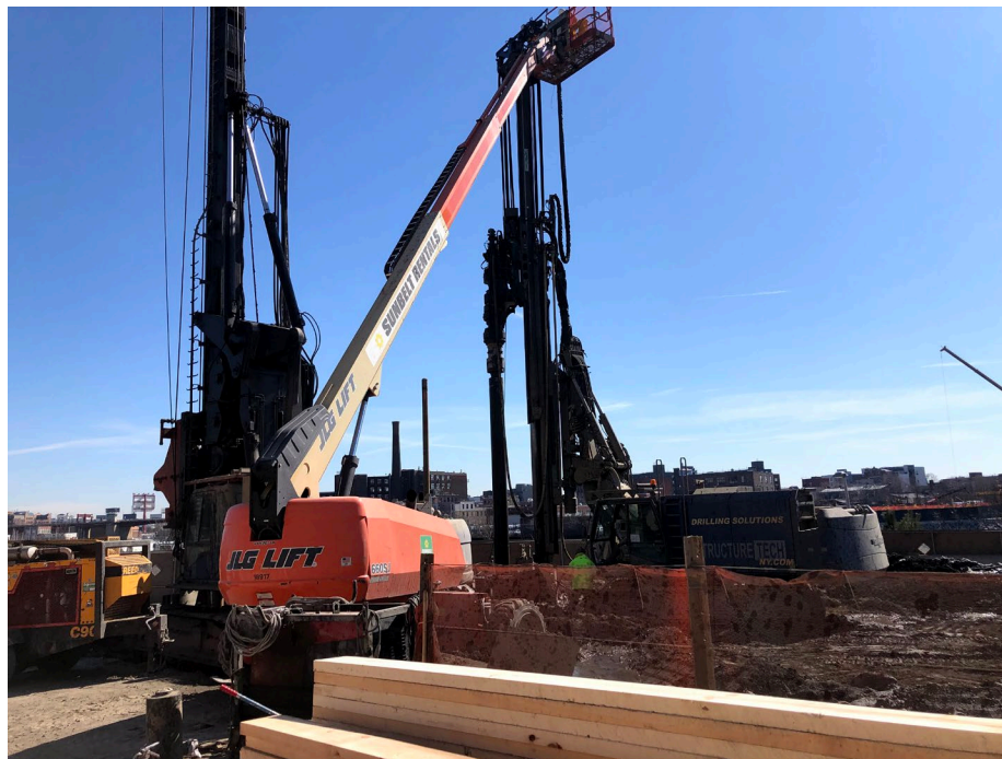
Photo 4: Progress of StructureTech installing piles in WCG-1/WCG-4.
