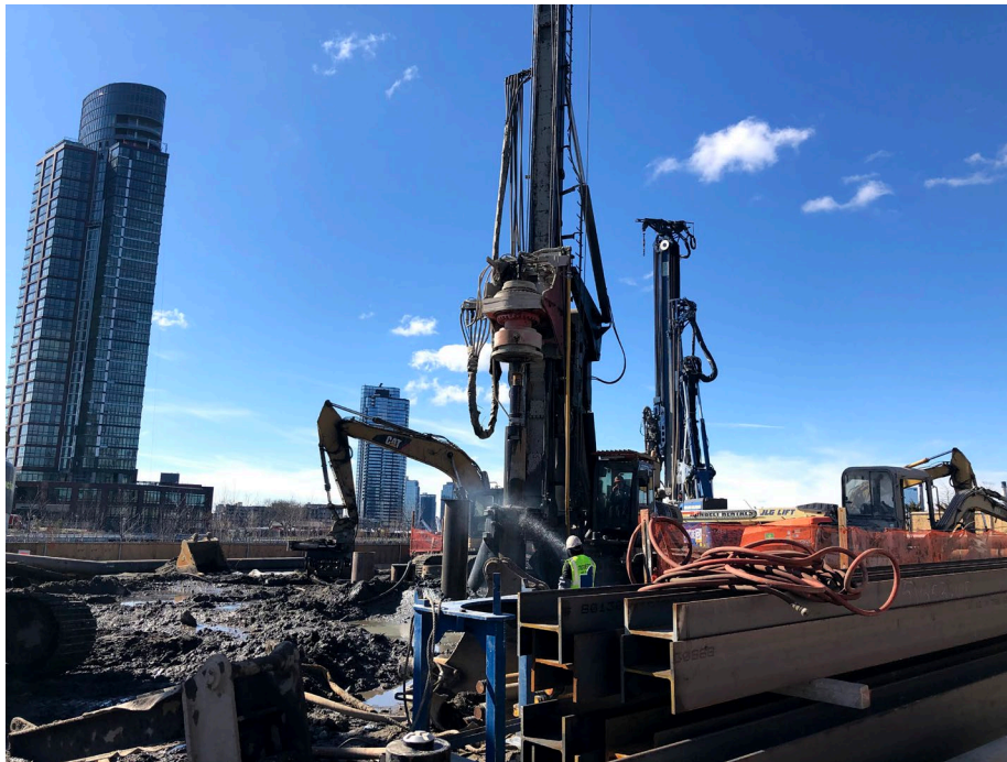
Photo 4: Looking southeast, StructureTech rock socket drilling in WCG-1.
