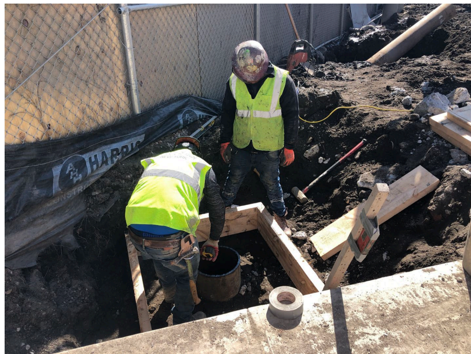
Photo 2: Looking southeast, StructureTech installing pile cap in WCG-4.
