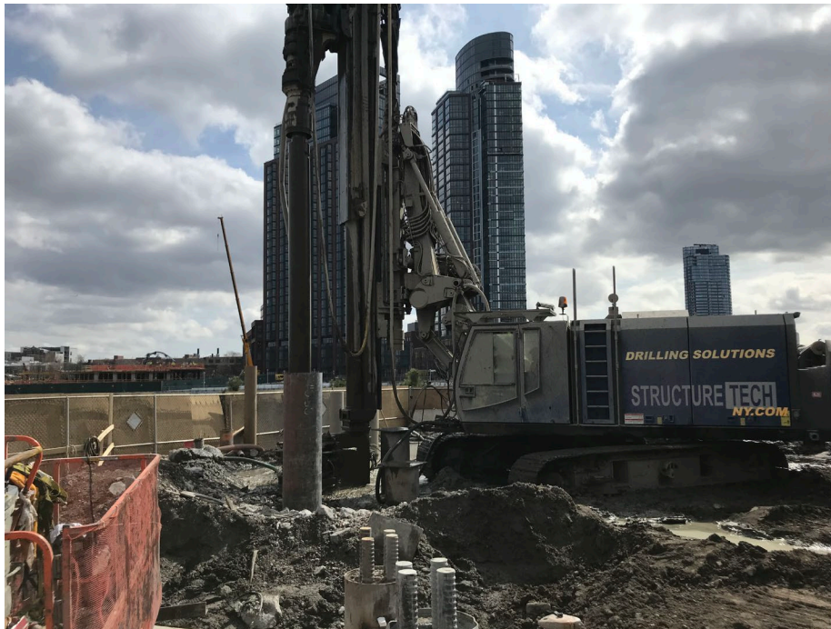
Photo 4: Looking south, StructureTech caisson drilling in WCG-2.
