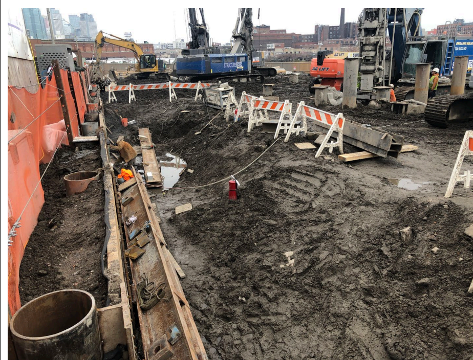
Photo 1: StructureTech installing and welding whalers in WCG-2 and WCG-3.
