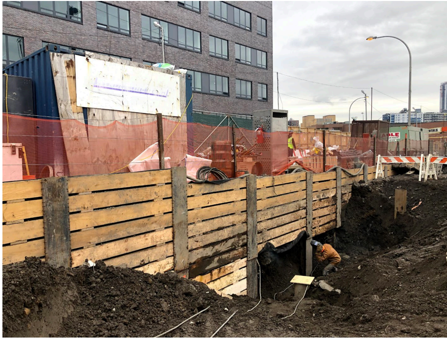
Photo 3: Looking northwest, StructureTech welding piles in WCG-3 at approx. 7 ft bls.
