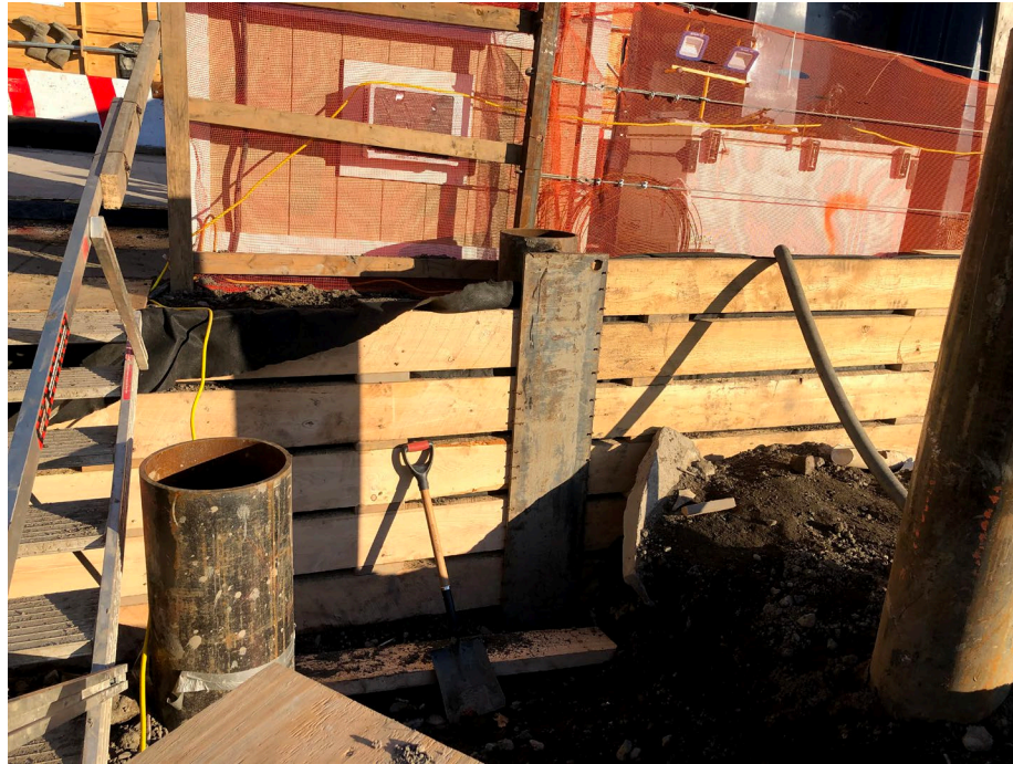
Photo 3: Looking northwest, view of shoring along perimeter in WCG-3.
