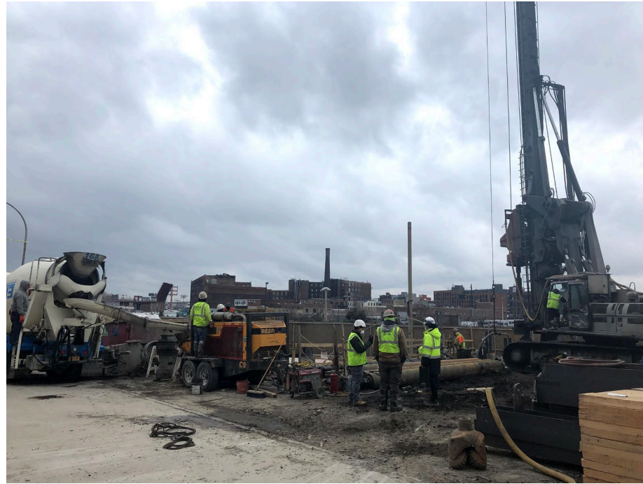
Photo 3: Looking east, StructureTech pumping grout into piles in WCG-4.
