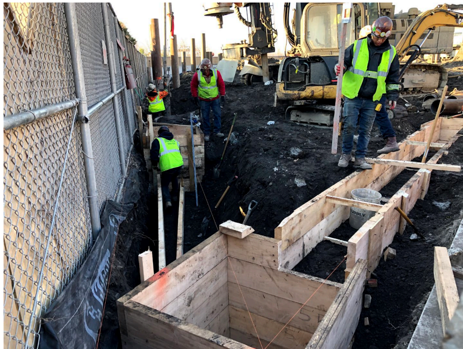
Photo 2: Looking southeast, StructureTech installing pile caps in WCG-4 toward the beginning of the workday.
