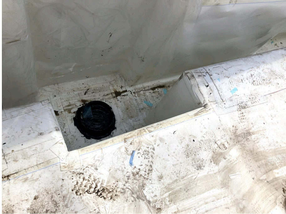
Photo 3: Photo showing taping at endlaps and corners as well as liquid mastic used to seal around penetration in WCG-4.
