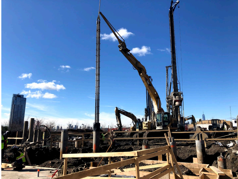
Photo 3: Looking south, StructureTech installing rebar in pile in WCG-4.
