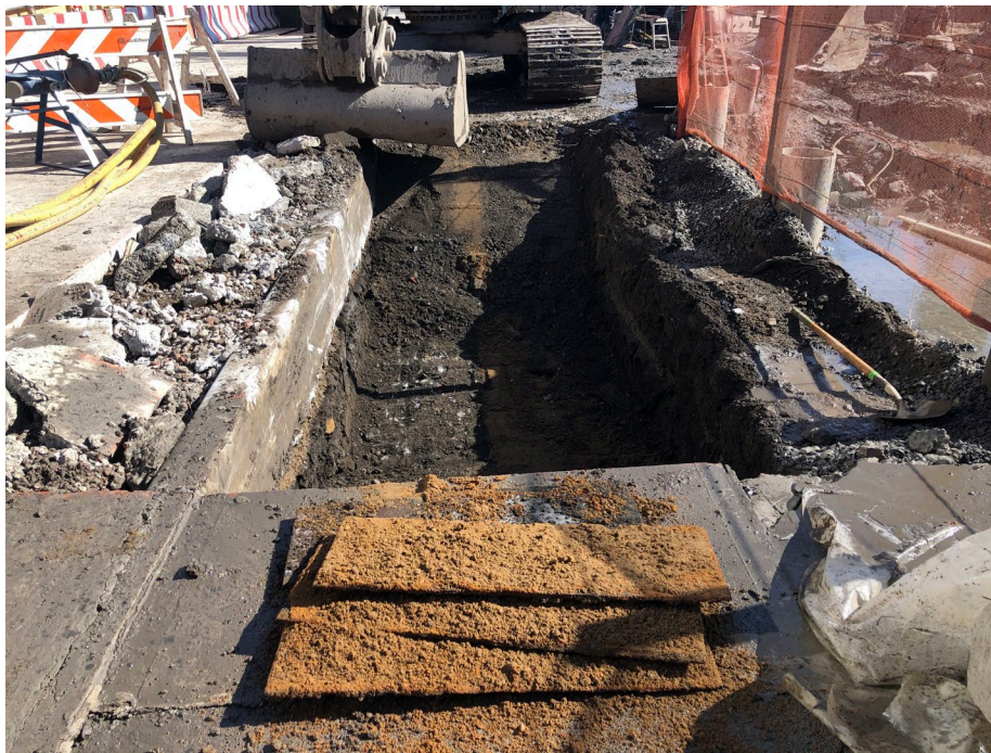
Photo 3: Looking northeast, StructureTech excavating crane pad test pit adjacent to WCG-1.
