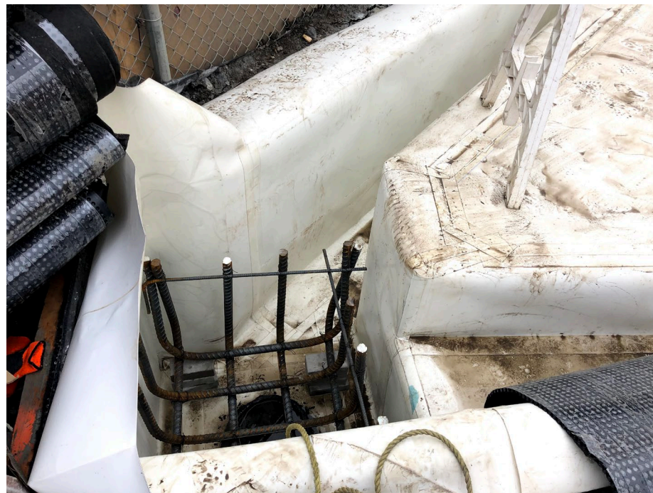
Photo 4: View of waterproofing and rebar installed in corner of rat slab in WCG-4.
