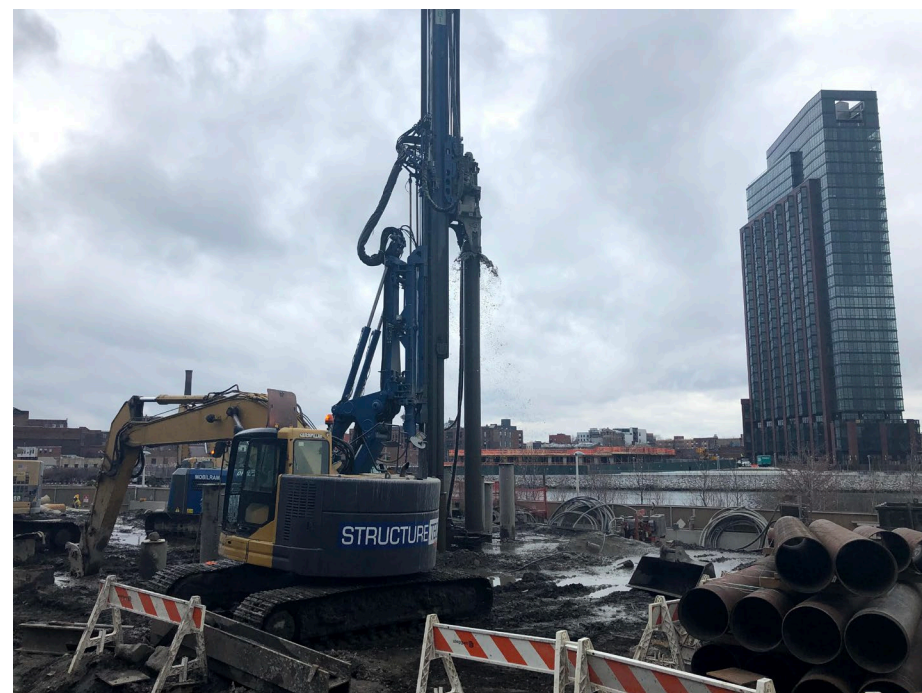
Photo 2: Looking east, StructureTech caisson drilling in WCG-2.
