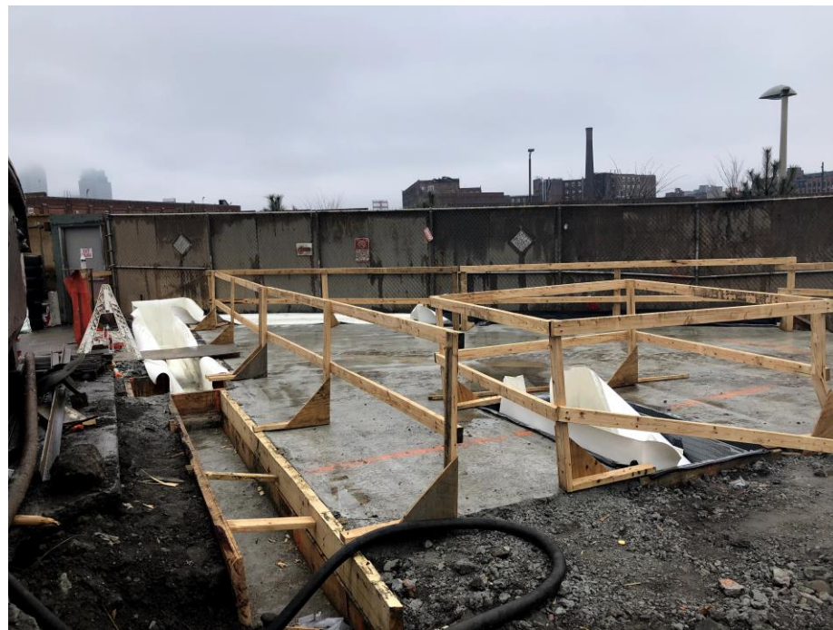
Photo 4: Looking northeast, status of north corner of site including rat slab in WCG-4.
