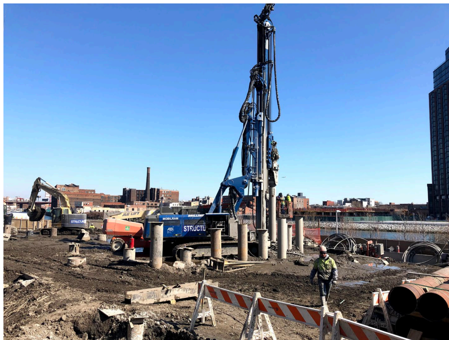
Photo 2: Looking east, StructureTech caisson drilling in WCG-2.
