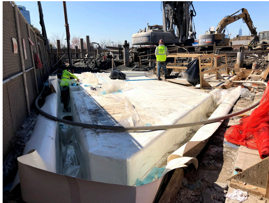
Photo 4: Looking south, StructureTech installing waterproofing in WCG-4.
