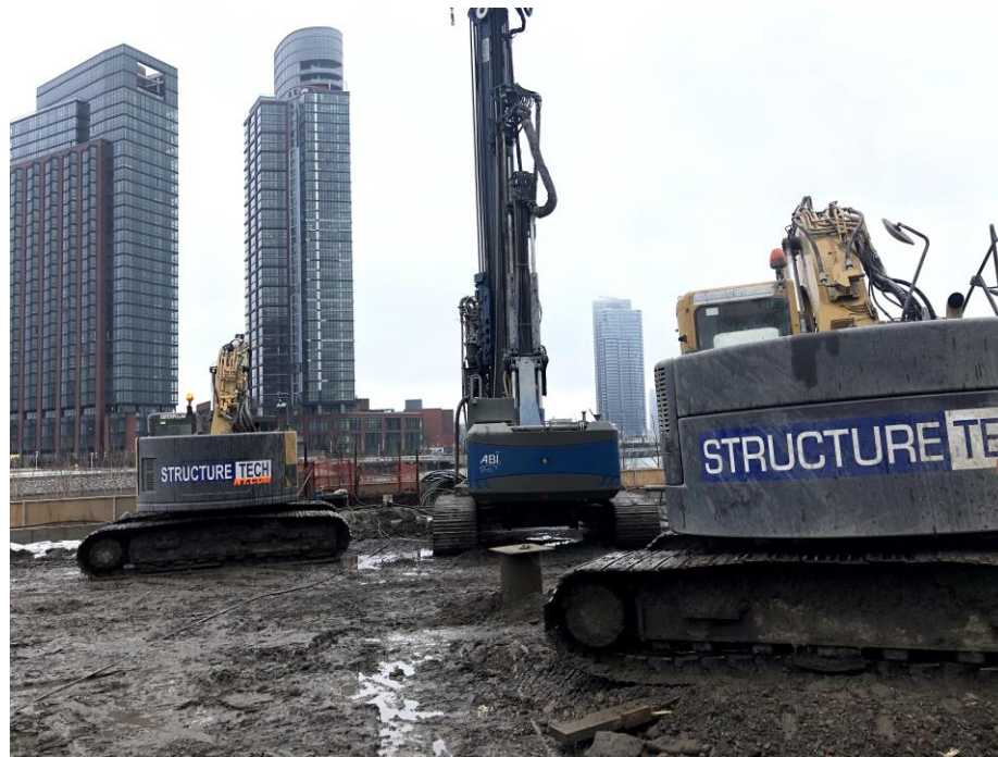
Photo 3: Looking southeast, StructureTech caisson drilling in WCG-2.
