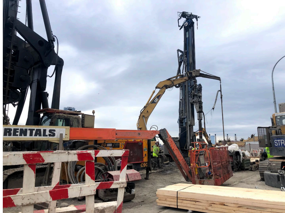
Photo 3: Looking southeast, status of northeast portion of site including StructureTech drilling and installing pile cap in WCG-4.
