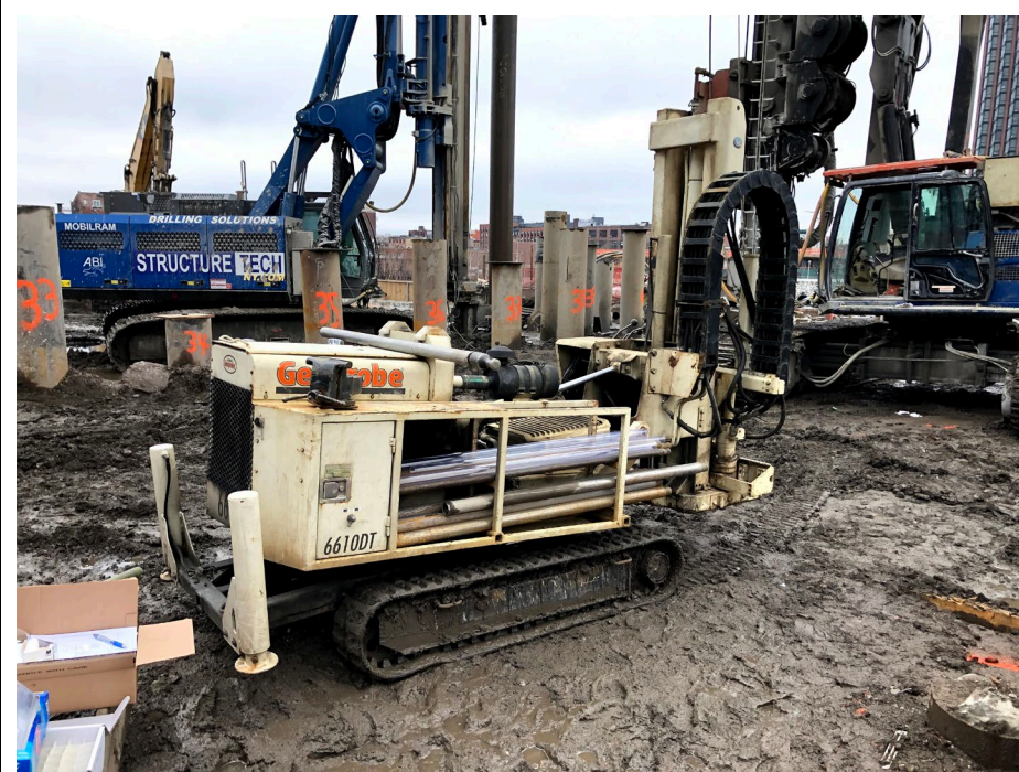
Photo 1: Looking east, view of geoprobe equipment used for soil sampling in WCG-3.
