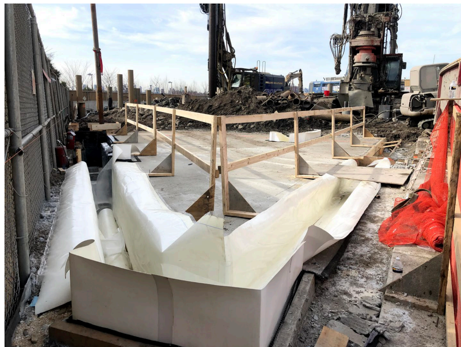
Photo 2: Looking south, status of northeast portion of site including rat slab in WCG-4 including waterproofing installation progress.
