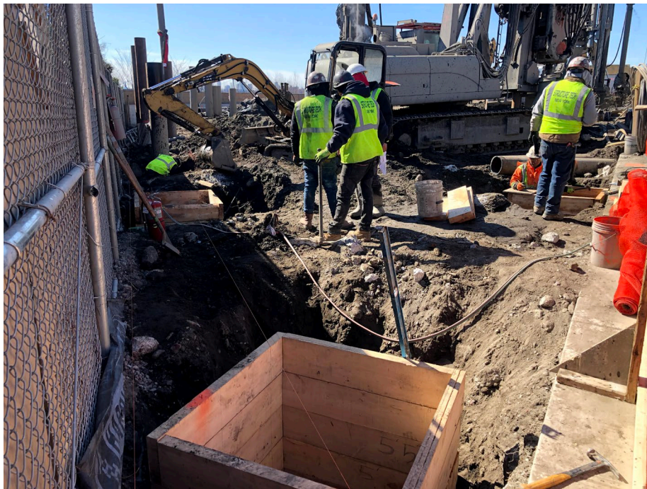
Photo 2: Looking southwest, StructureTech installing pile caps in WCG-4.
