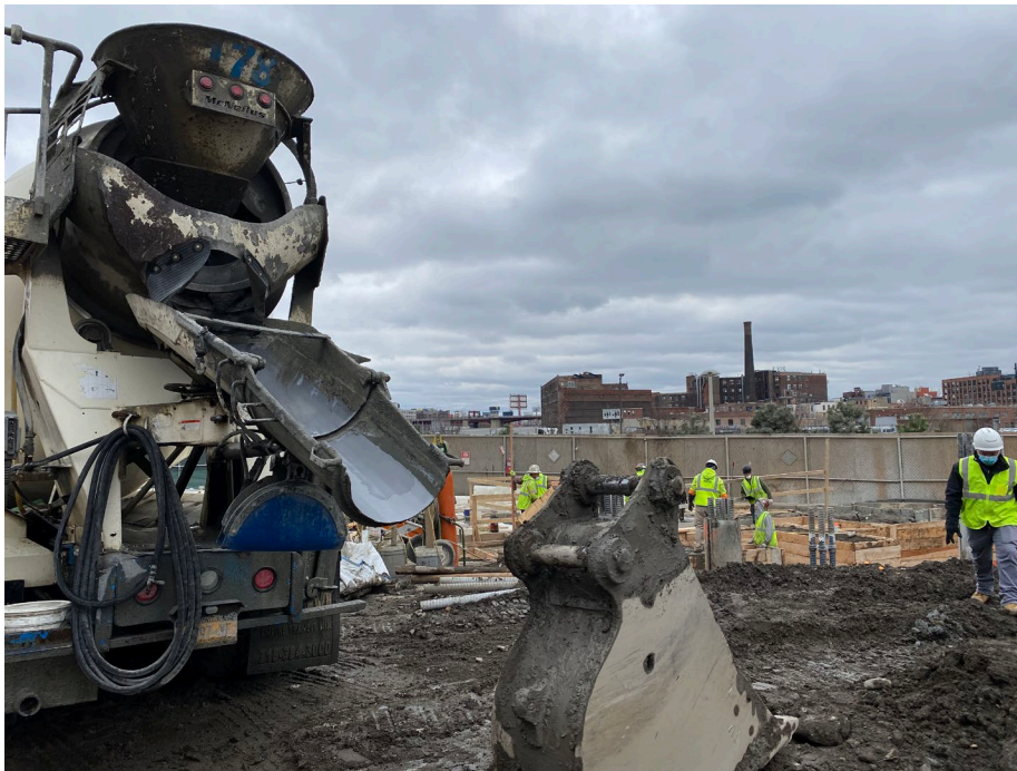
Photo 4: Looking West, StructureTech prepares to pour 6 yds of concrete for the next portion of their rat slab in Grid WCG-4.
