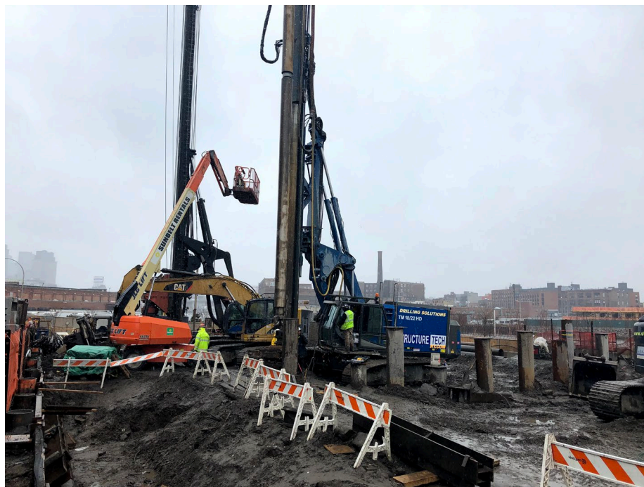
Photo 2: Looking east, StructureTech drilling caissons in WCG-2.
