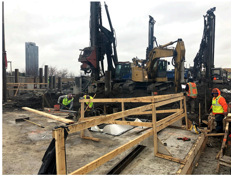
Photo 4: Looking east, view of StructureTech hand digging and installing pile caps/grade beams in WCG-4.
