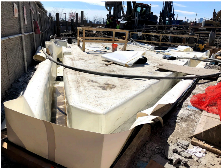
Photo 4: Looking south, status of water proofing in WCG-4.
