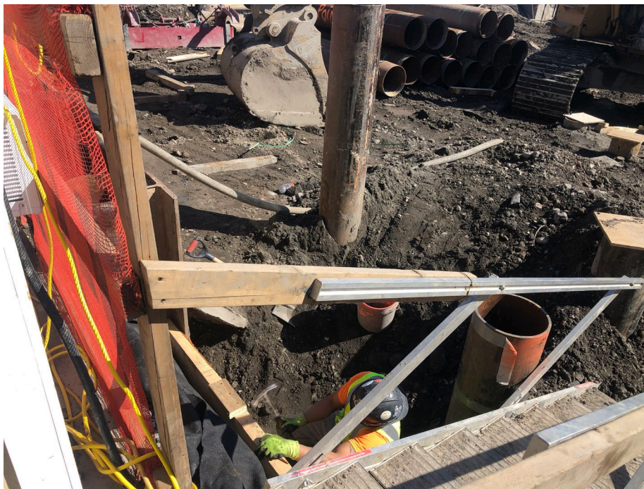
Photo 4: Looking southeast, StructureTech shoring in WCG-3.
