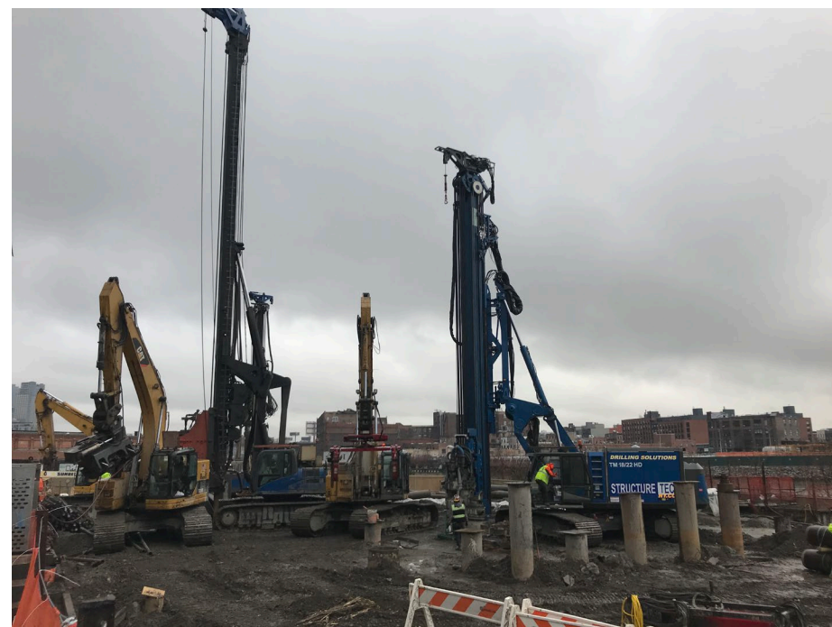
Photo 2: Looking southeast, site overview, StructureTech caisson drilling.
