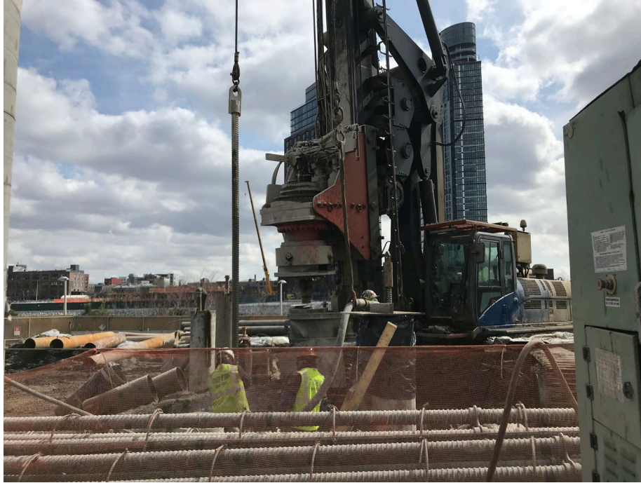
Photo 3: Looking southeast, StructureTech caisson drilling in WCG-2.
