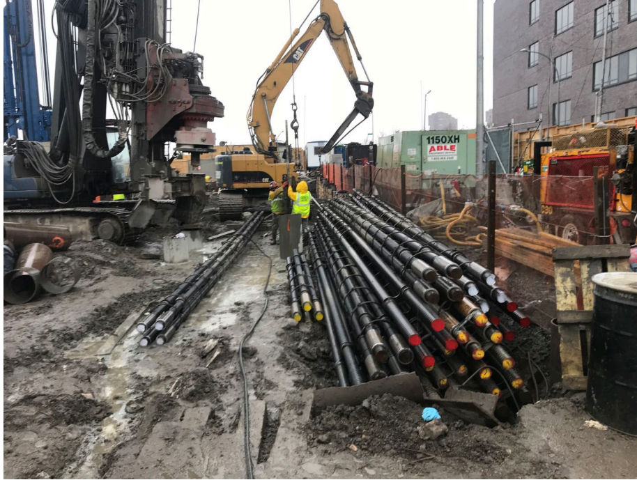
Photo 3: Looking west, StructureTech rigging rebar beams for piles.
