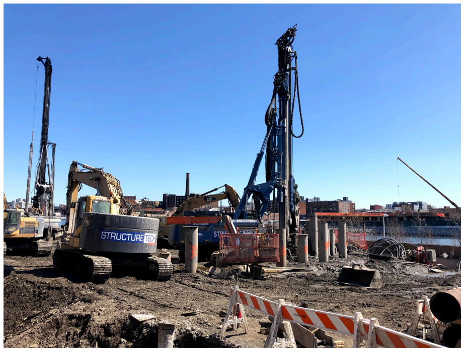
Photo 2: Looking east, StructureTech caisson drilling in WCG-2.
