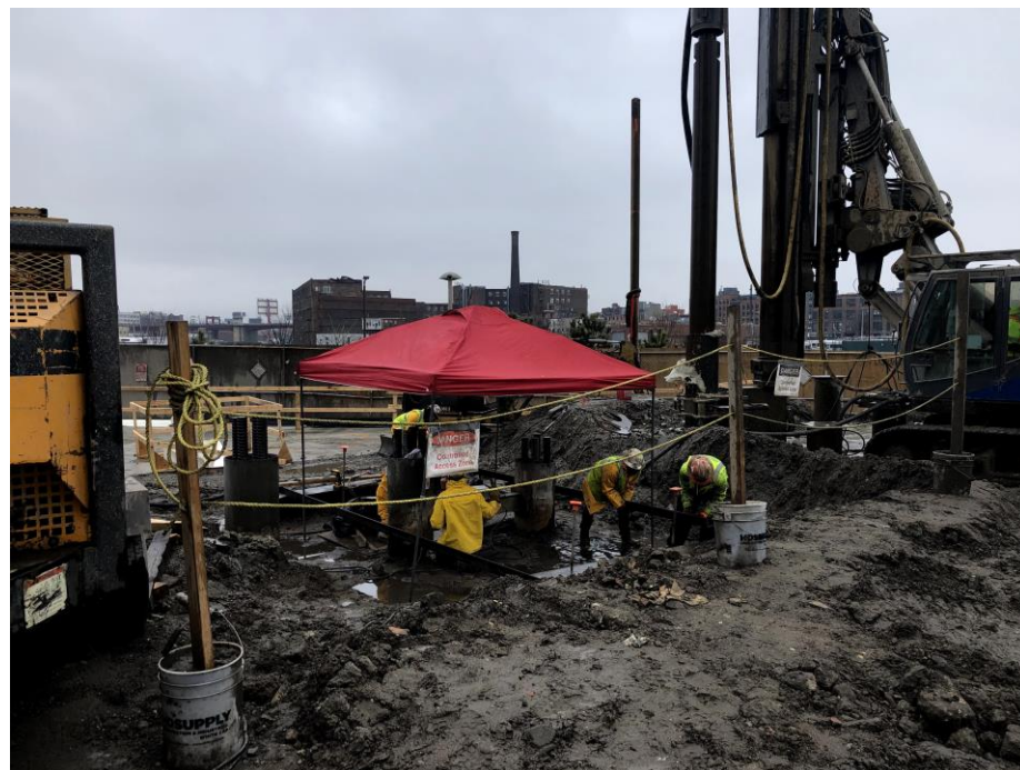
Photo 2: Looking east, StructureTech setting up load test platform in WCG-4.
