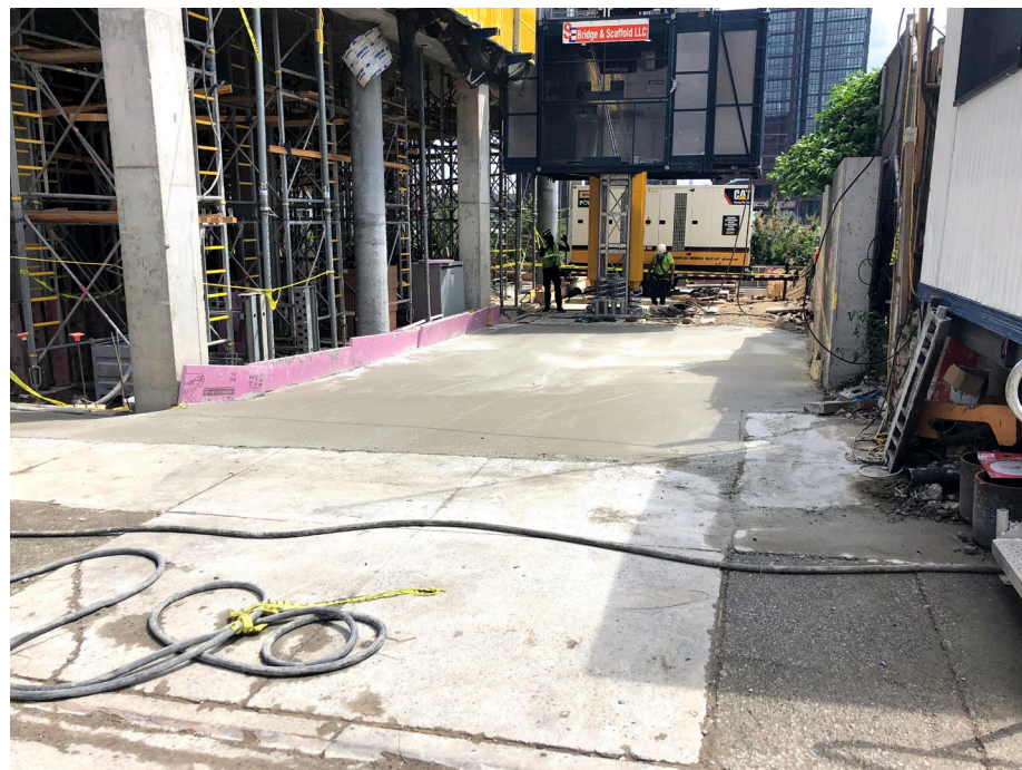
Photo 2: Looking southeast, view of freshly poured concrete to cover existing Site soil along the southwest perimeter of the Site in WCG-3.
