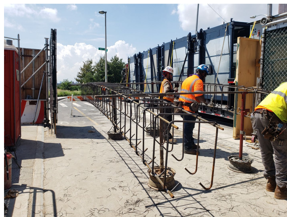
Photo 1: Looking west, a view of SBF prefabricating columns to be installed in the fifth floor of superstructure.
