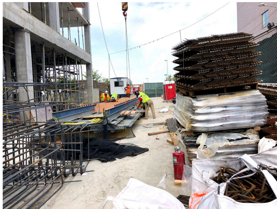
Photo 2: Looking southwest, SBF preparing safety cocoons for installation on building side.
