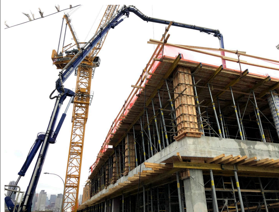
Photo 1: View of concrete pumping in progress to create the third-floor south deck.
