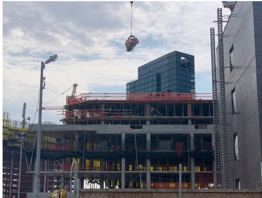
Photo 1: Looking south, SBF pouring concrete on top floor of the superstructure in grid WCG-4.
