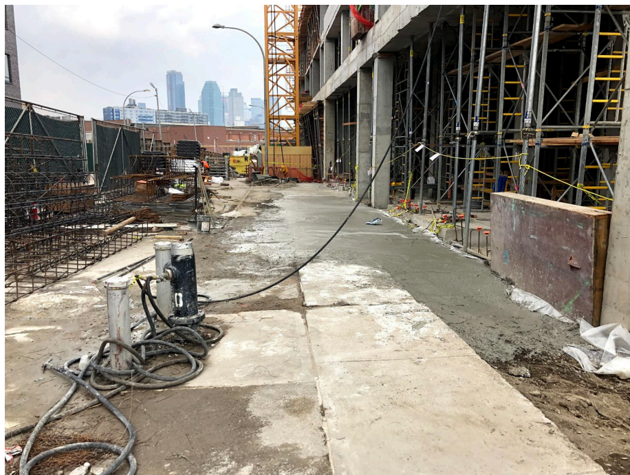
Photo 2: Looking northeast, view of concrete strip poured to cover existing Site soil.
