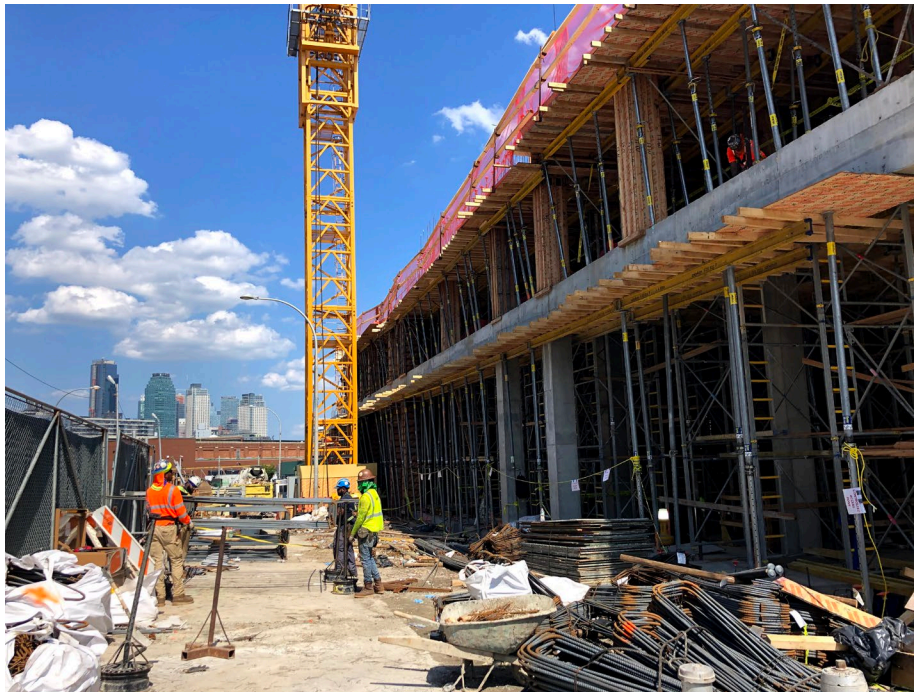
Photo 4: Looking northeast, Site status including SBF prefabricating rebar columns.
