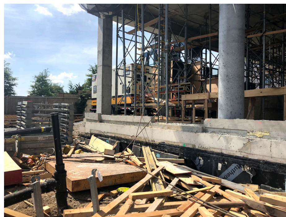
Photo 2: Looking west, view of concrete soil coverage and waterproofing progress in the south corner of the Site.
