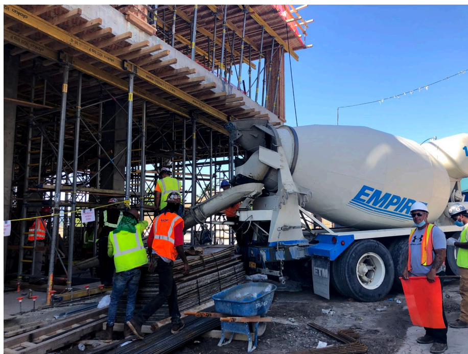
Photo 2: View of Empire concrete truck onsite and SBF pouring basement stairs.
