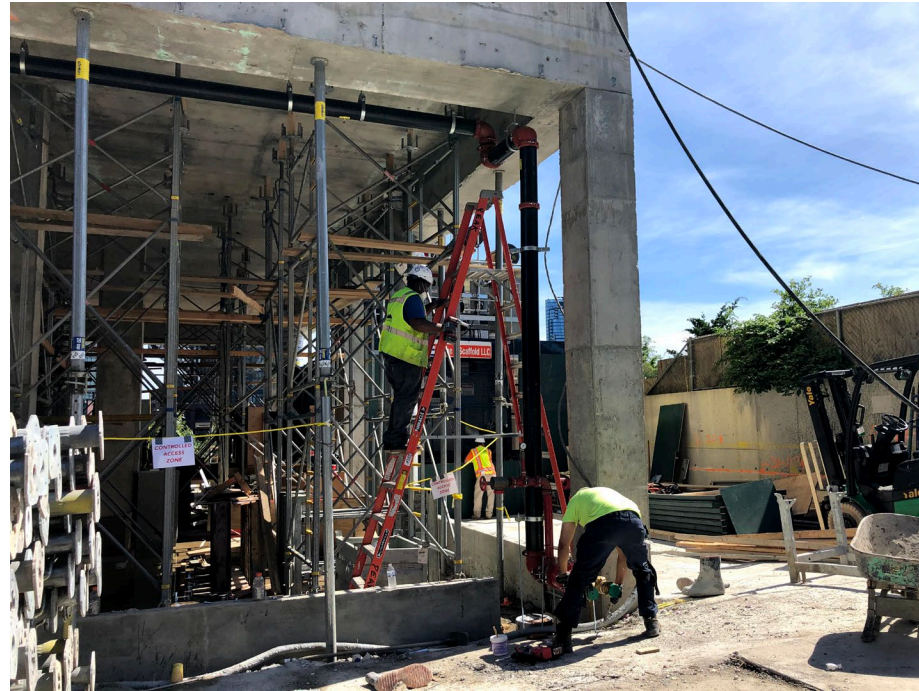
Photo 3: View of standpipe installation progress in WCG-3.
