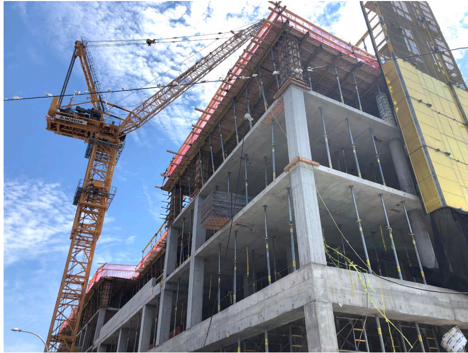
Photo 3: View of superstructure progress and installed safety cocoons from standing in WCG-3.
