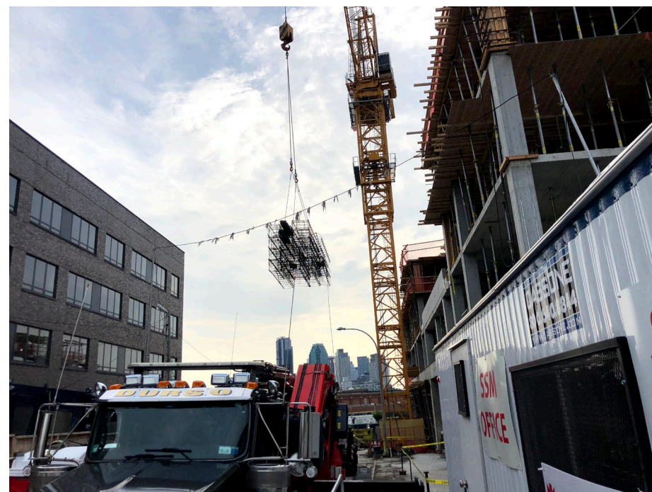
Photo 2: Looking northeast, view of crane transporting prefabricated rebar columns from the ground to superstructure.
