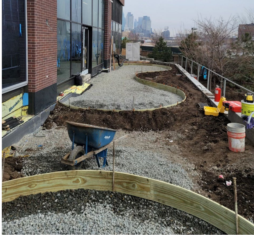
Photo 1: Photo of the permanent Site cover system installation.
