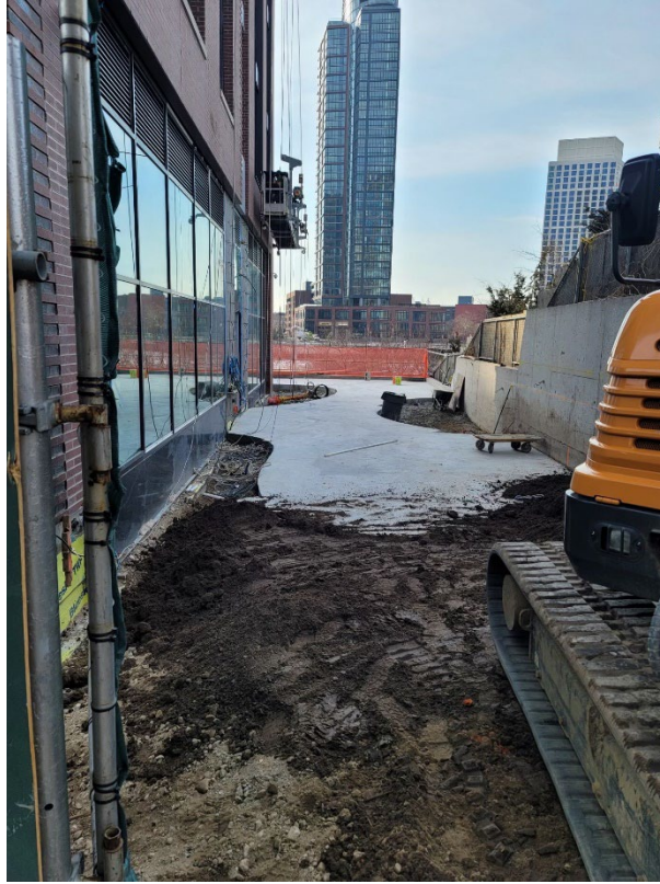
Photo 5: Photo of the Site cover system topsoil installation.
