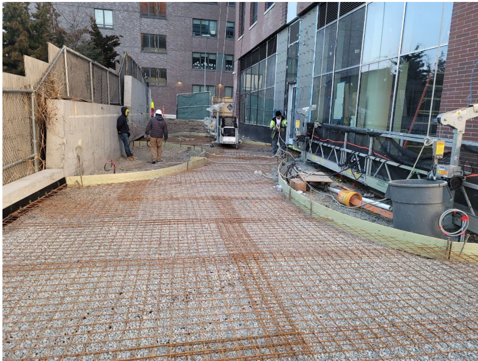
Photo 4: Photo of the permanent Site cover system installation.
