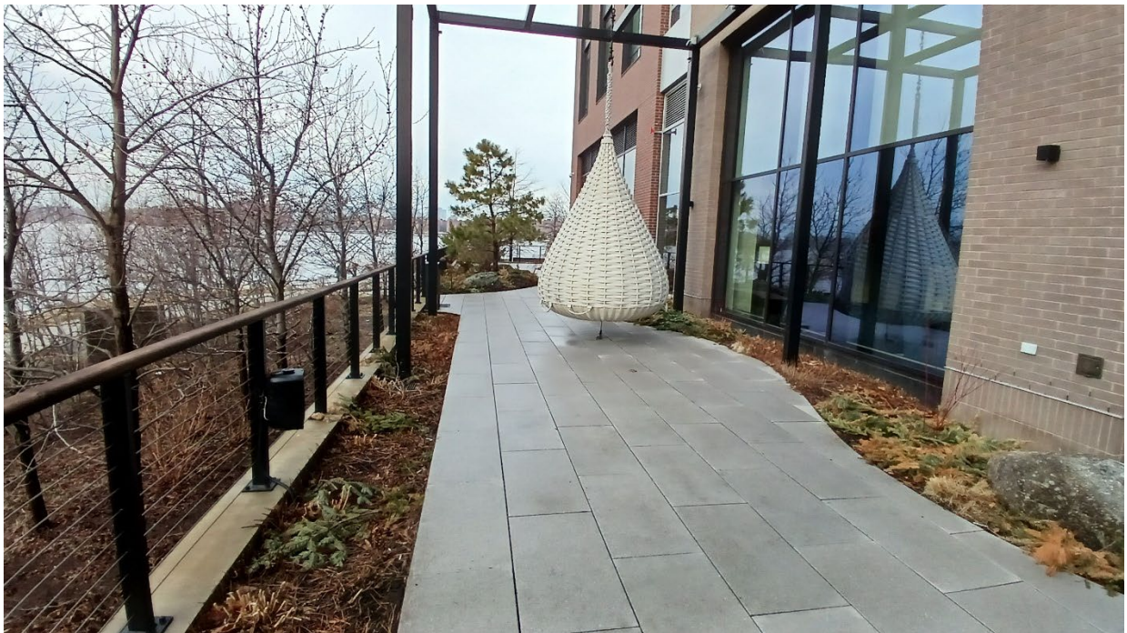
Photograph 2: View of the south outdoor patio area.
