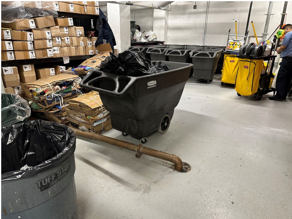
Photo 4: Trash compactor room with floor drain located in basement.
