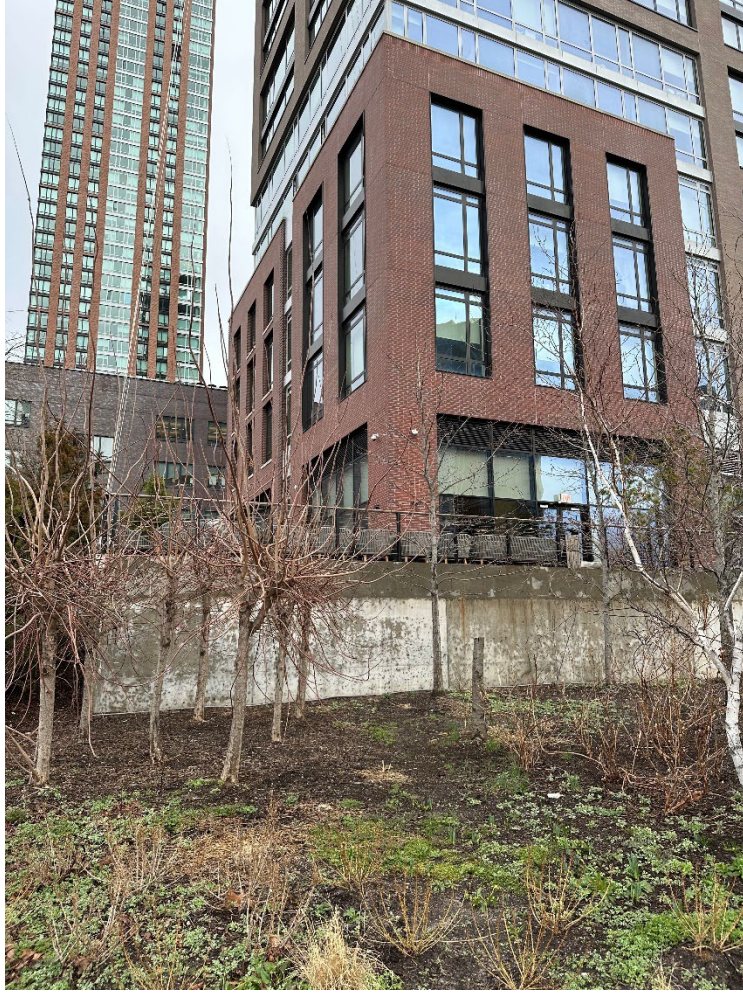
Photo 8: View of the concrete retaining wall.
