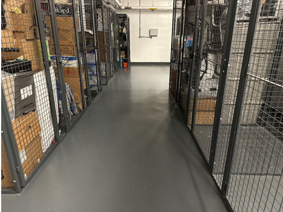
Photo 1: Residential storage area in basement.
