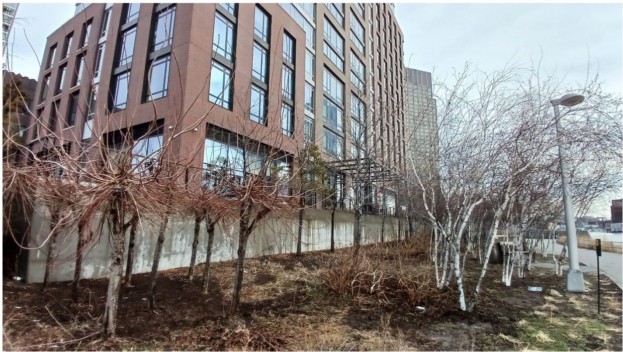
Photograph 11: View of the concrete retaining wall along the building's southern exterior.
