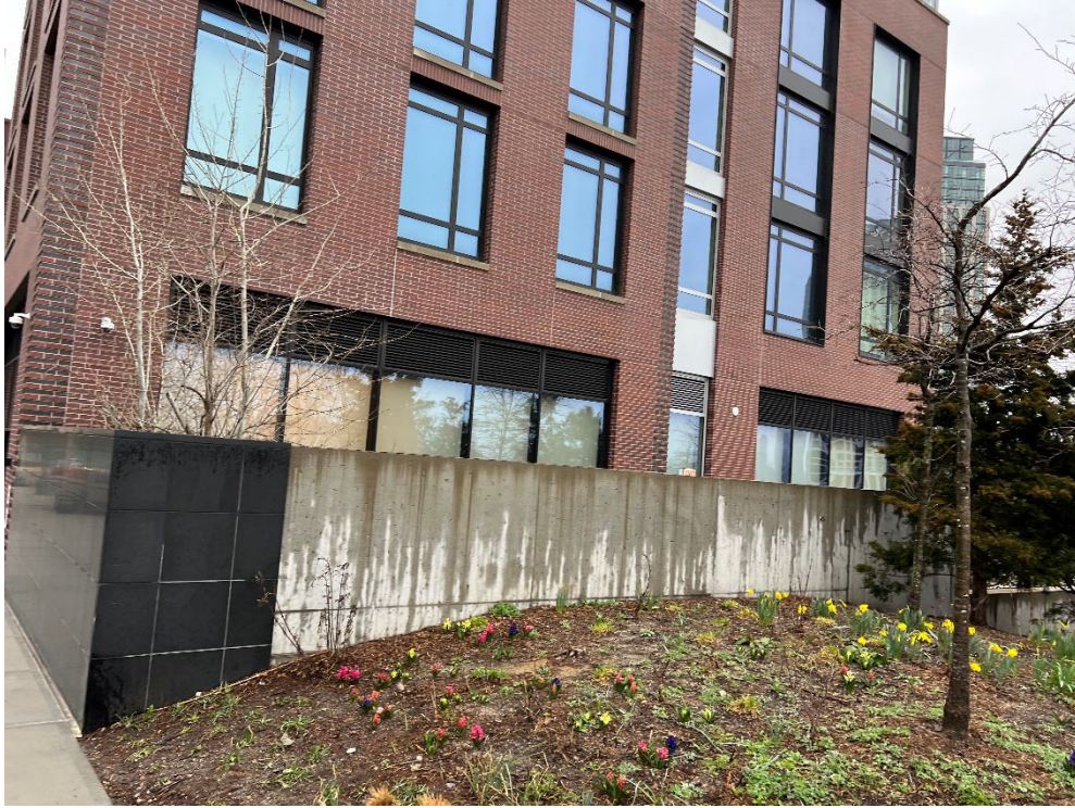
Photo 9: View of the concrete retaining wall outside of the building.
