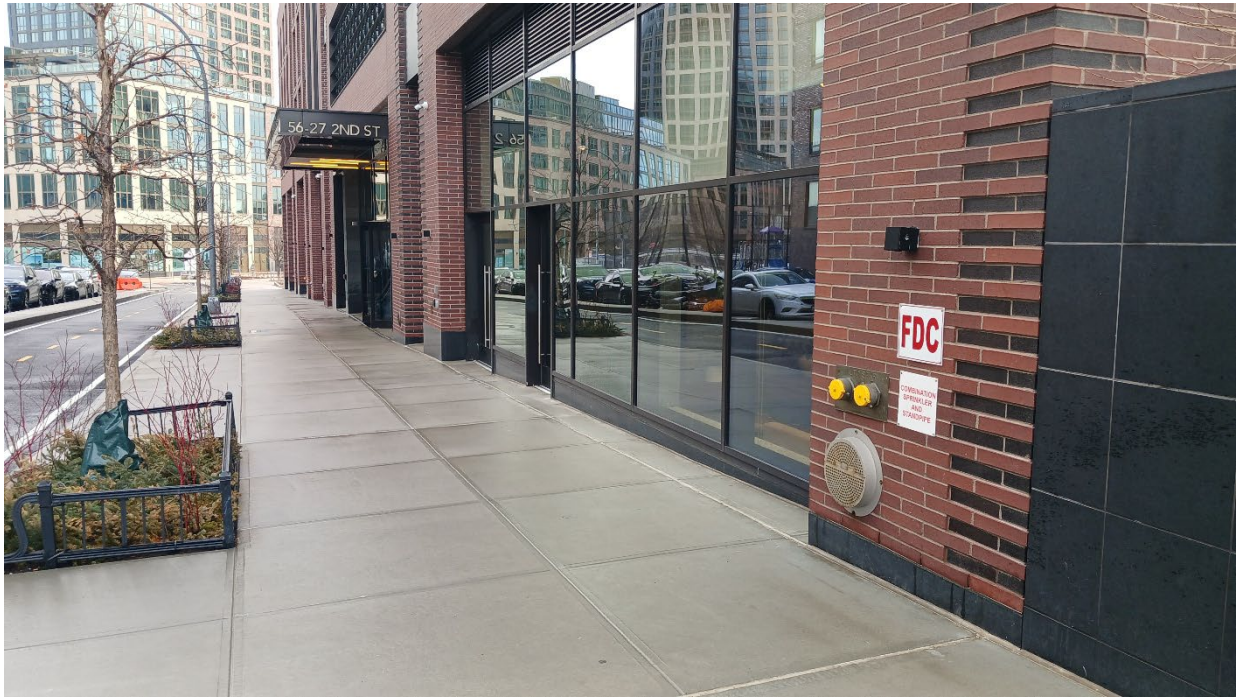
Photograph 1: View of the building exterior and sidewalk along 2 nd Street.
