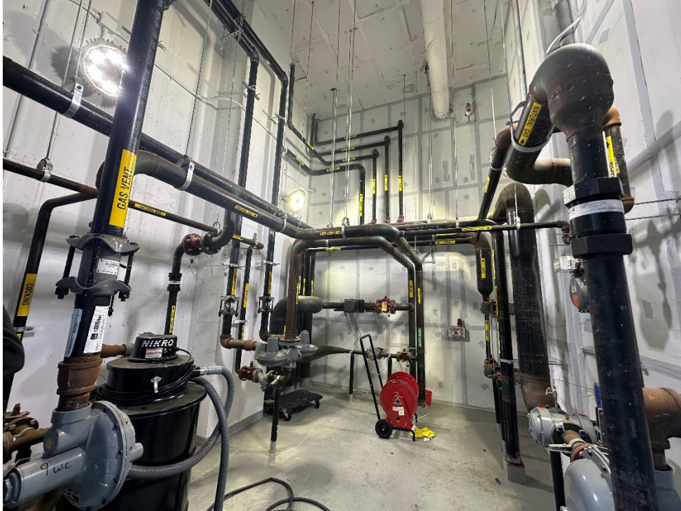
Photo 5: Gas room located next to the lobby.
