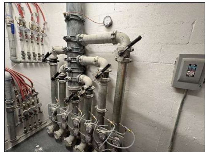
Photograph 4: SSDS manifold and accessories.
