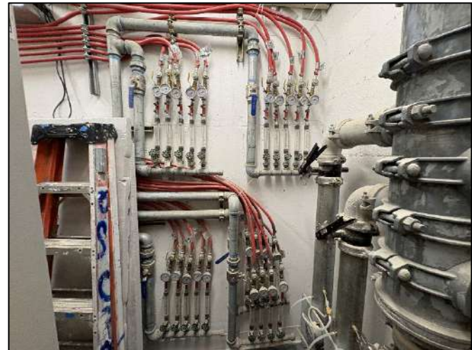
Photograph 2: Biosparge Manifold.
