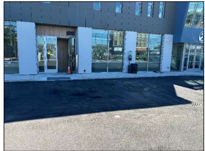
Photograph 4: The parking lot at the front of the building.
