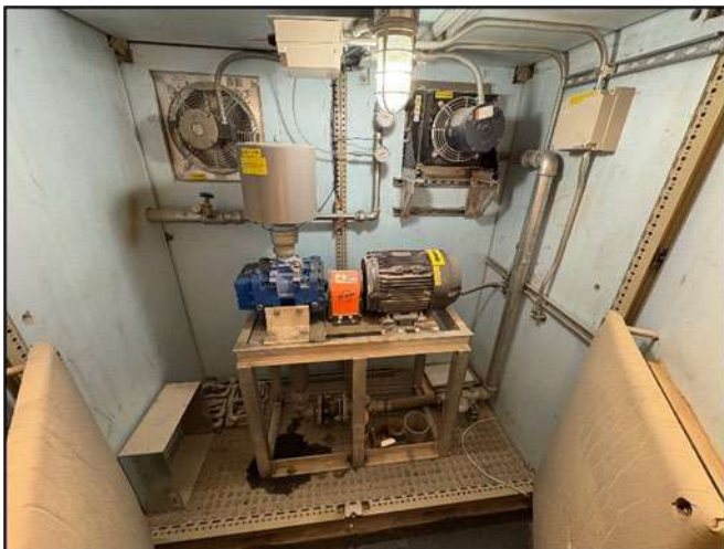
Photograph 3: Biosparge Compressor.
