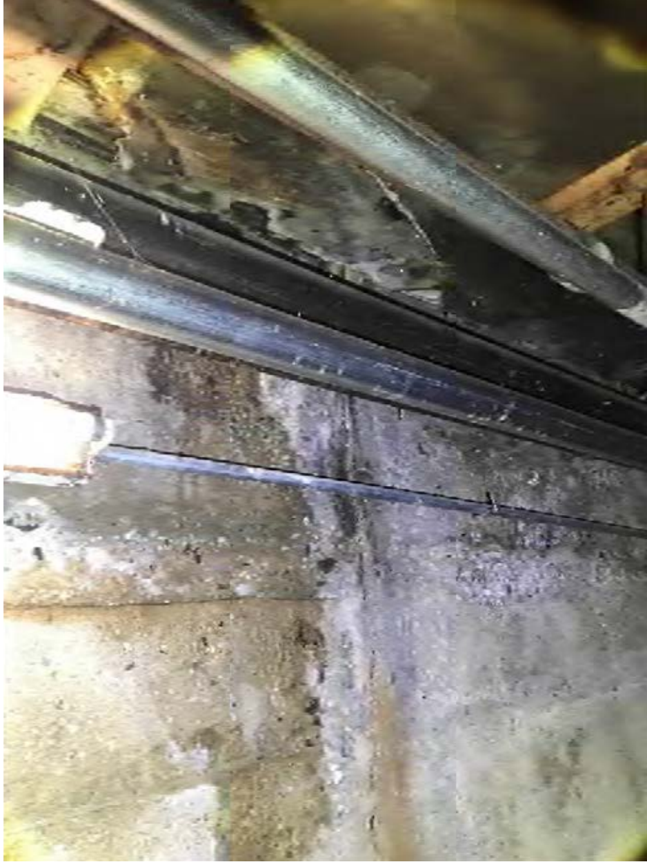
Photo 10 Moisture on basement walls.
