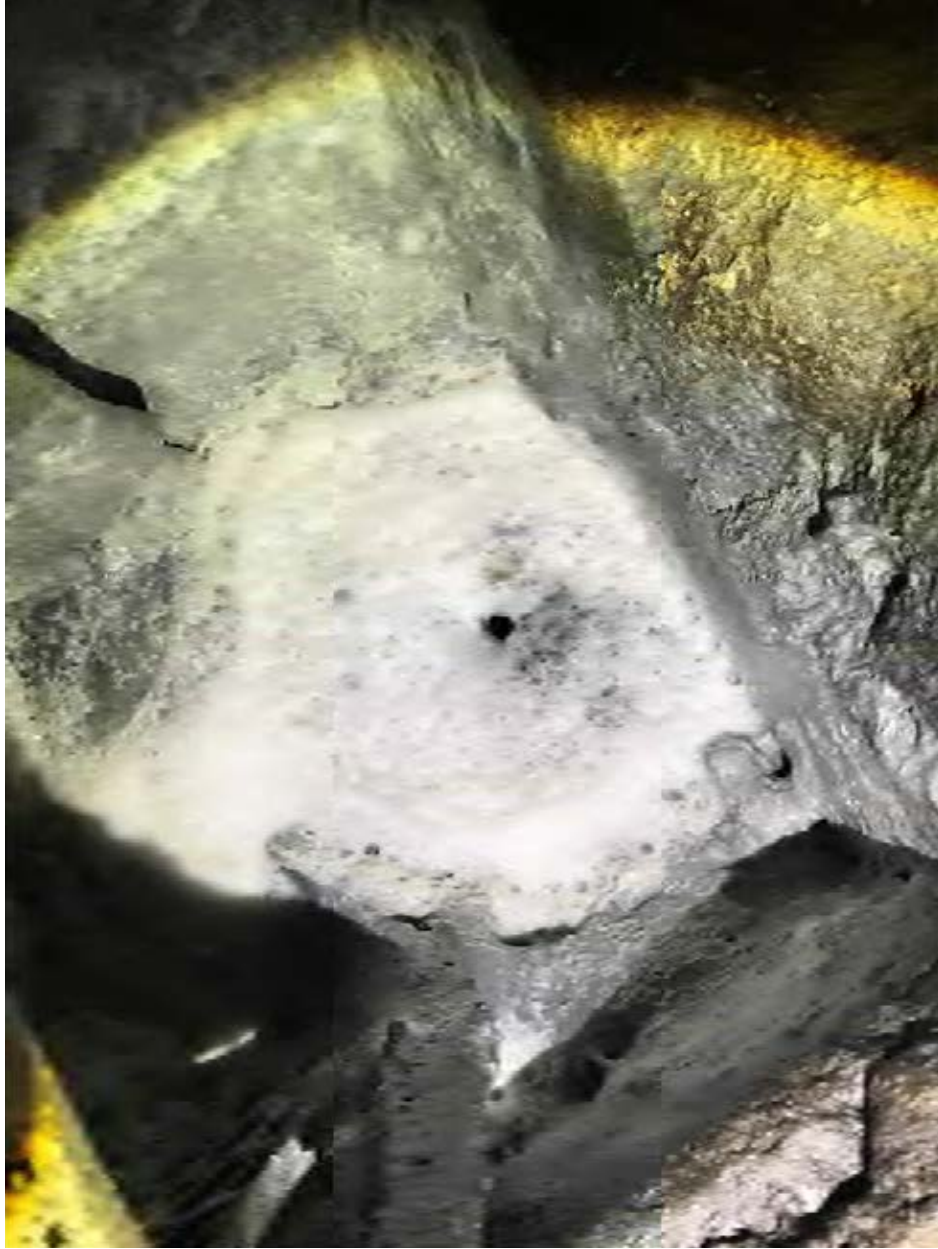
Photo 11 Soap discharge in basement sump.
