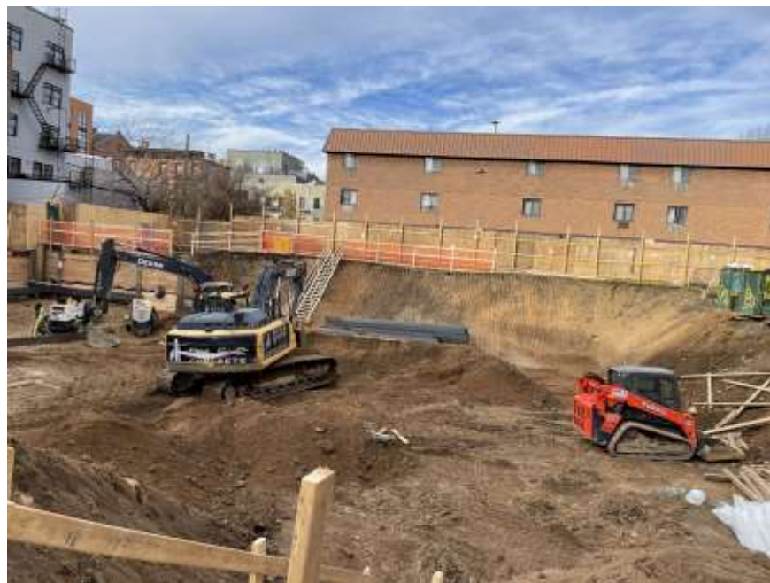
Photo 2: View of Rise grading non-hazardous fill in the north-central part of the site to create a stable working surface for equipment (facing northwest).
