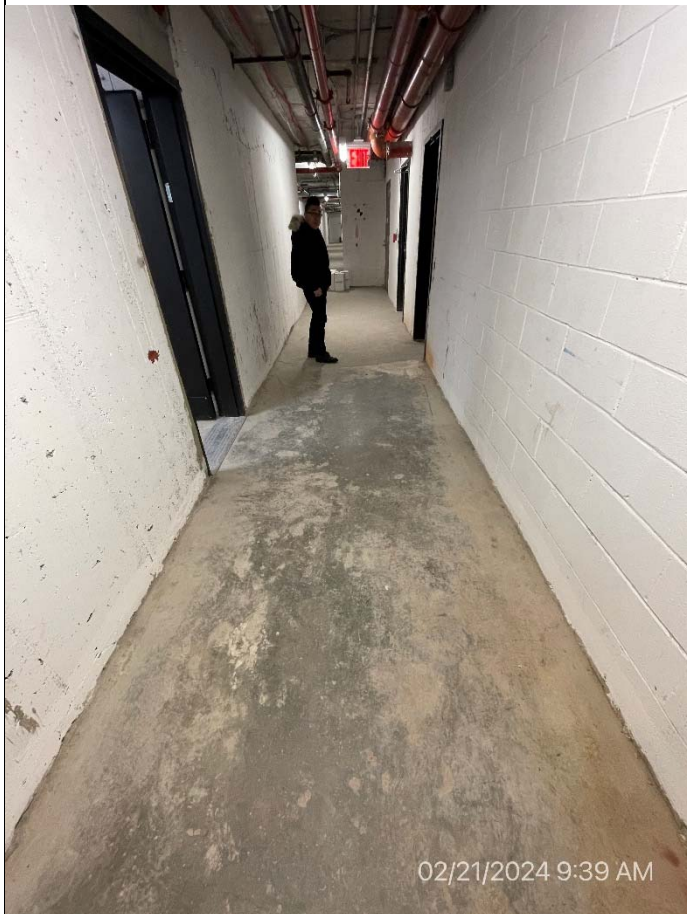
Hallway at western end of Site
