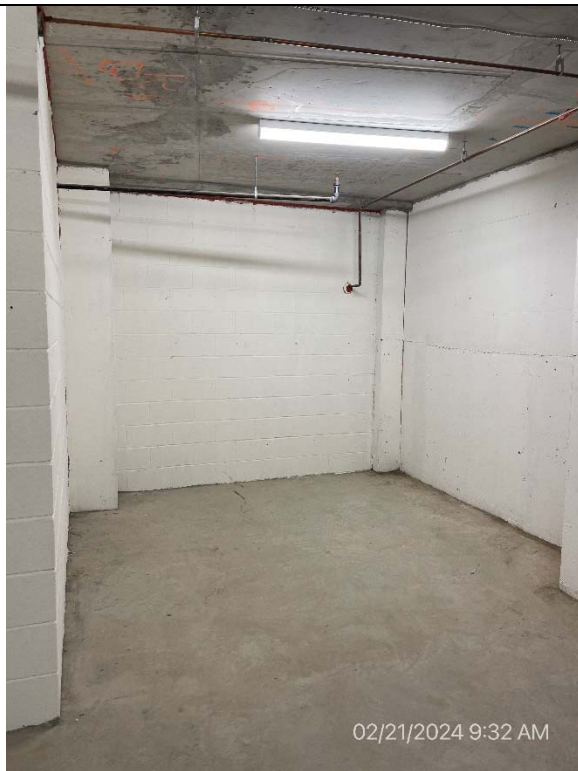
Large Storage Room (south eastern corner)
