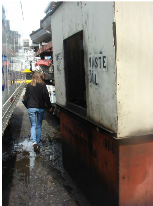
Photo 11: View of the exterior waste oil AST with a capacity of 450 gallons located adjacent to the repair shop
