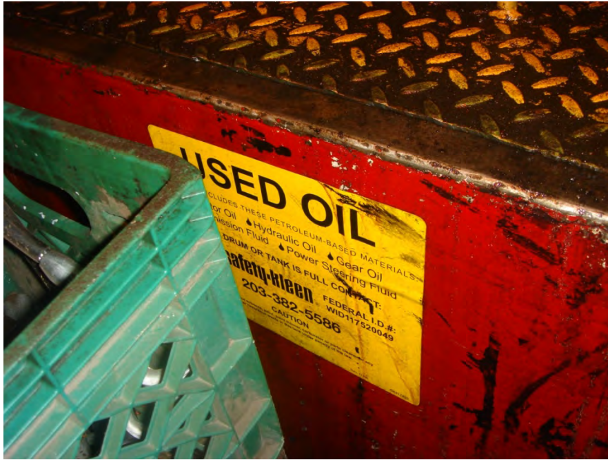
Photo 11: View of a waste oil AST with a capacity of 150 gallons located in the repair shop
