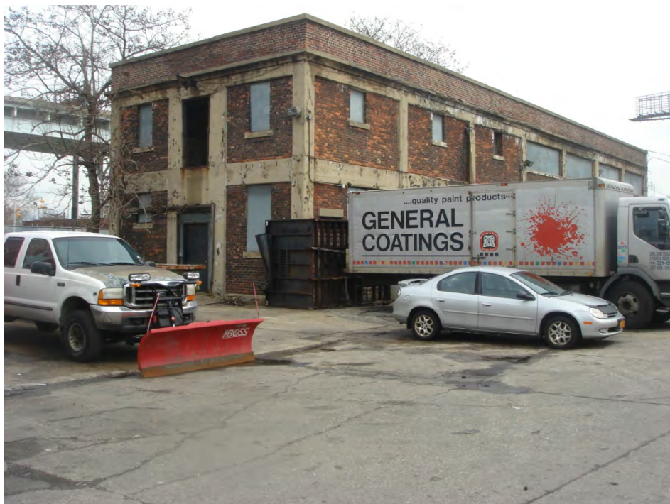
Photo 3: View of the two story vacant masonry building on the northern boundary of the Site
