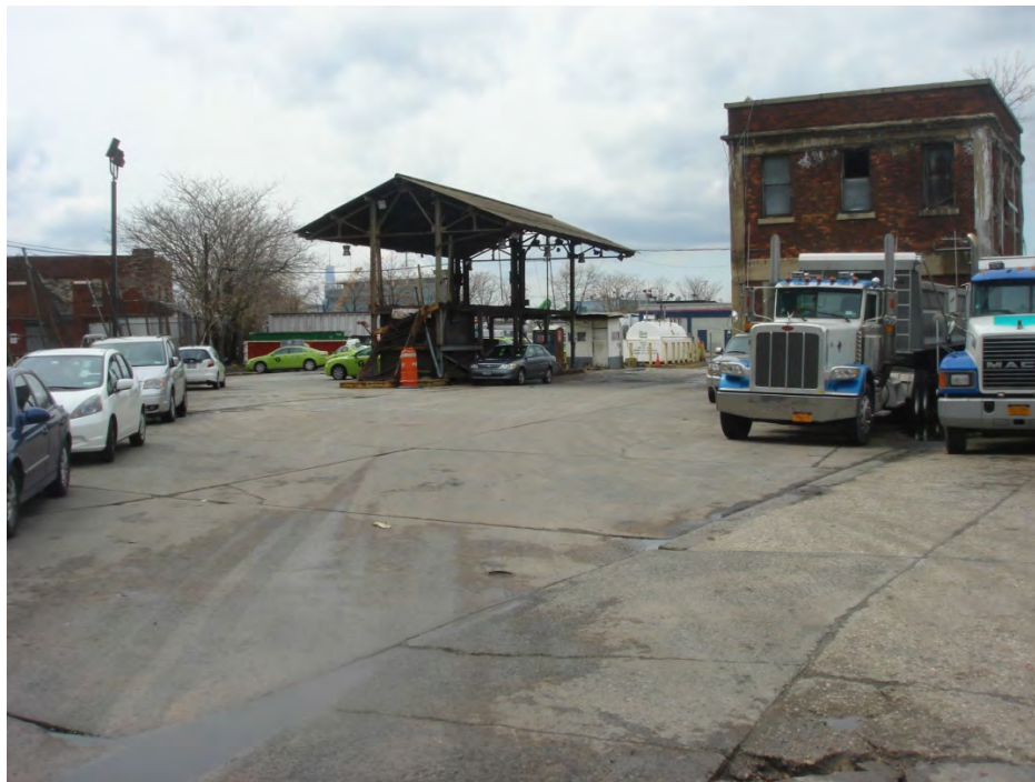
Photo 5: View of the former fueling racks and two story masonry building on the northern eastern boundary of the Site
