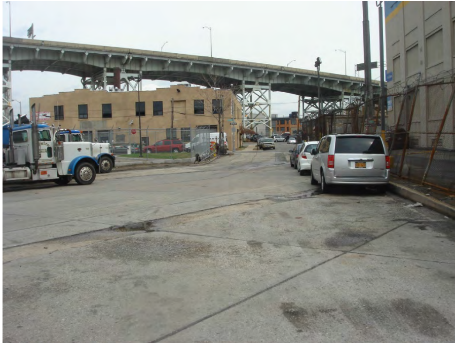
Photo 11: View of the Review Avenue street entrance onto the Site and adjacent eastern properties
