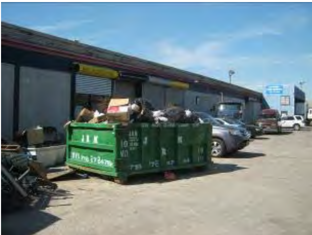
11. View of Building E on the subject property
