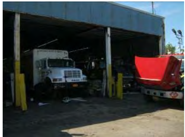
10. View of Building D on the subject property
