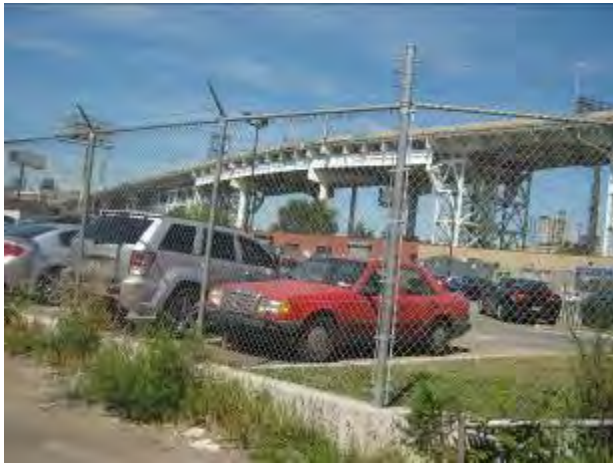
33. View of northern adjacent parking lot
