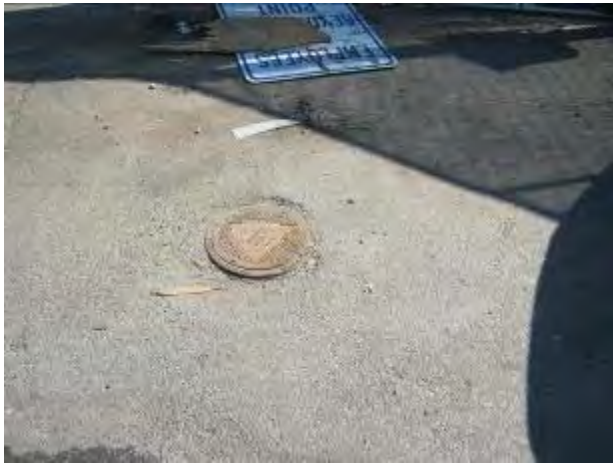
25. View of closed-in-place monitoring well
