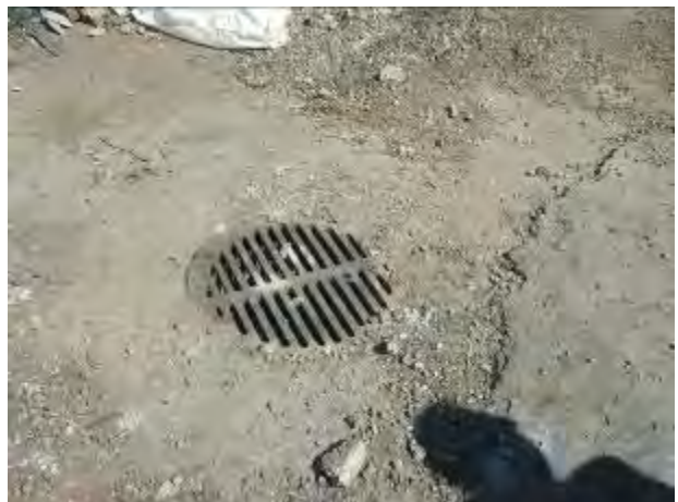
24. View of typical stormwater drain in the paved areas of the subject property
