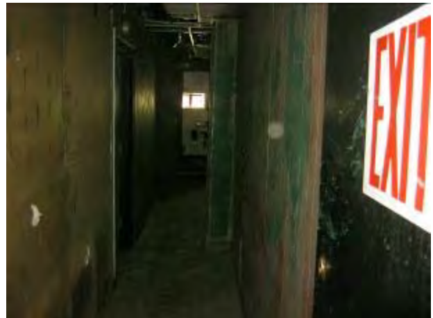
12. View inside Building E on the subject property
