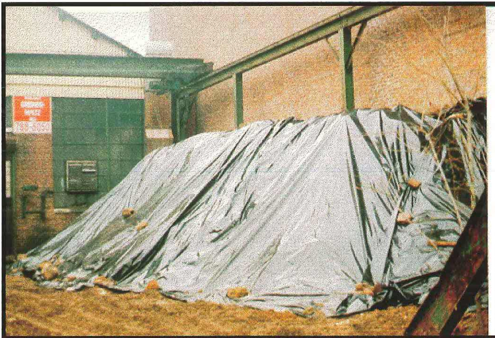
Stockpiled Contaminated Soils
