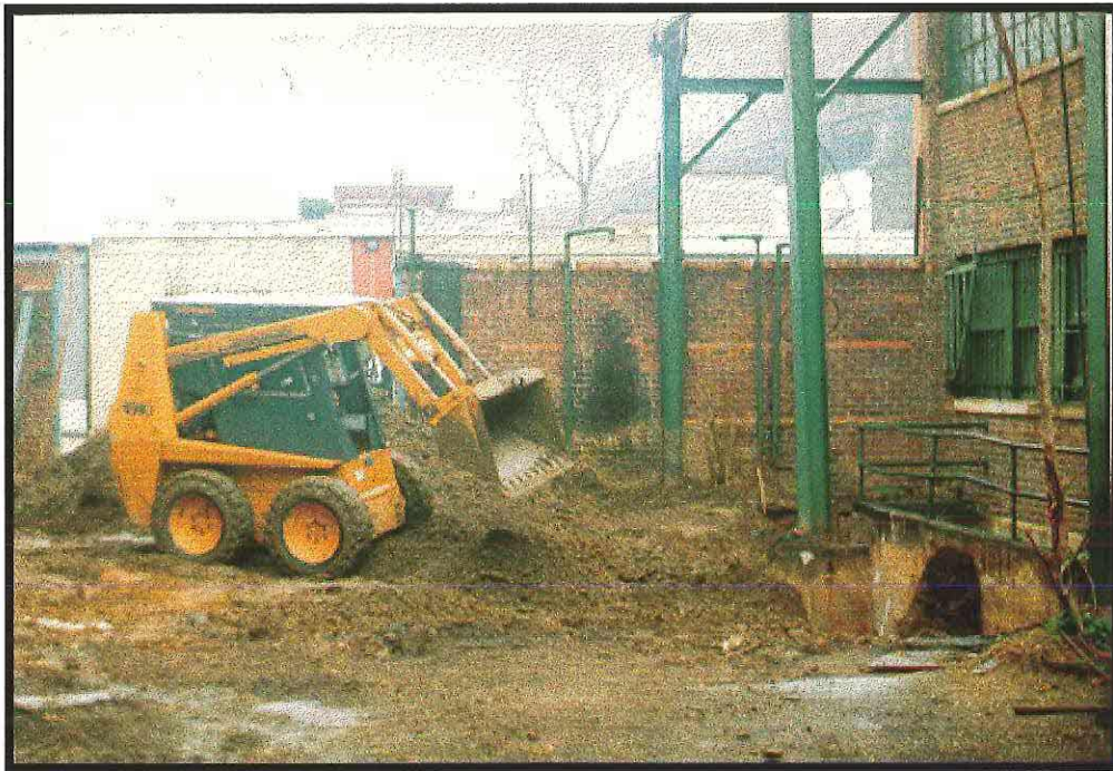
Backfill and Grading of Excavation
