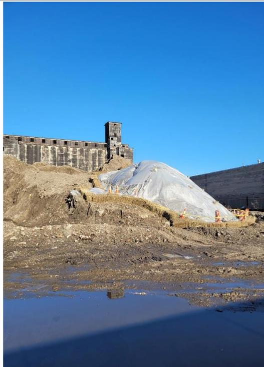
Photo 10: Stockpile covered with polyethylene sheeting and surrounded with hay bales, facing west. 03/21/2024.
