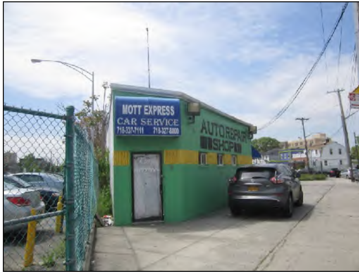
Photograph 9. An auto repair shop west-adjacent to the Property, view south from Beach 22 nd Street.
