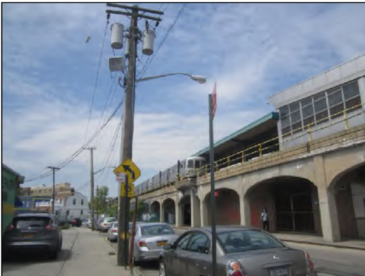
Photograph 11. Elevated MTA A Line tracks and Mott Avenue station west of the Property, view south from Mott Avenue.
