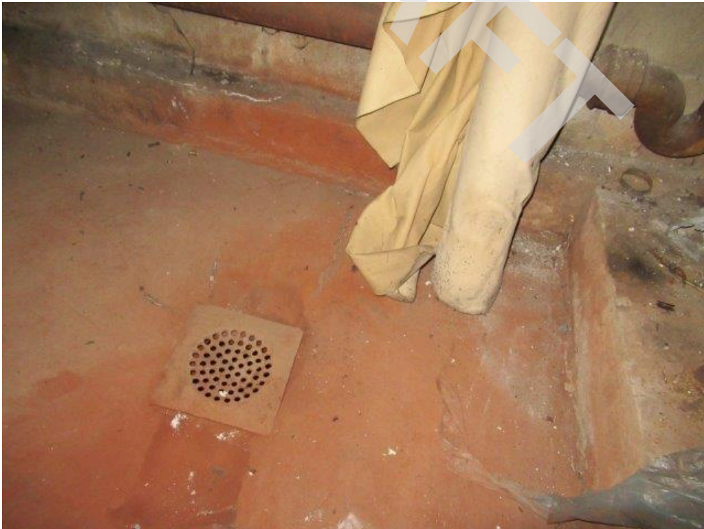
View of basement floor drain
