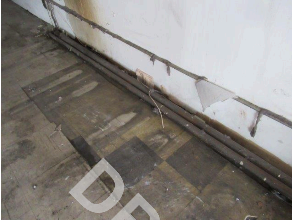
View of damaged 9" x 9" and 12" x 12" floor tile and piping
