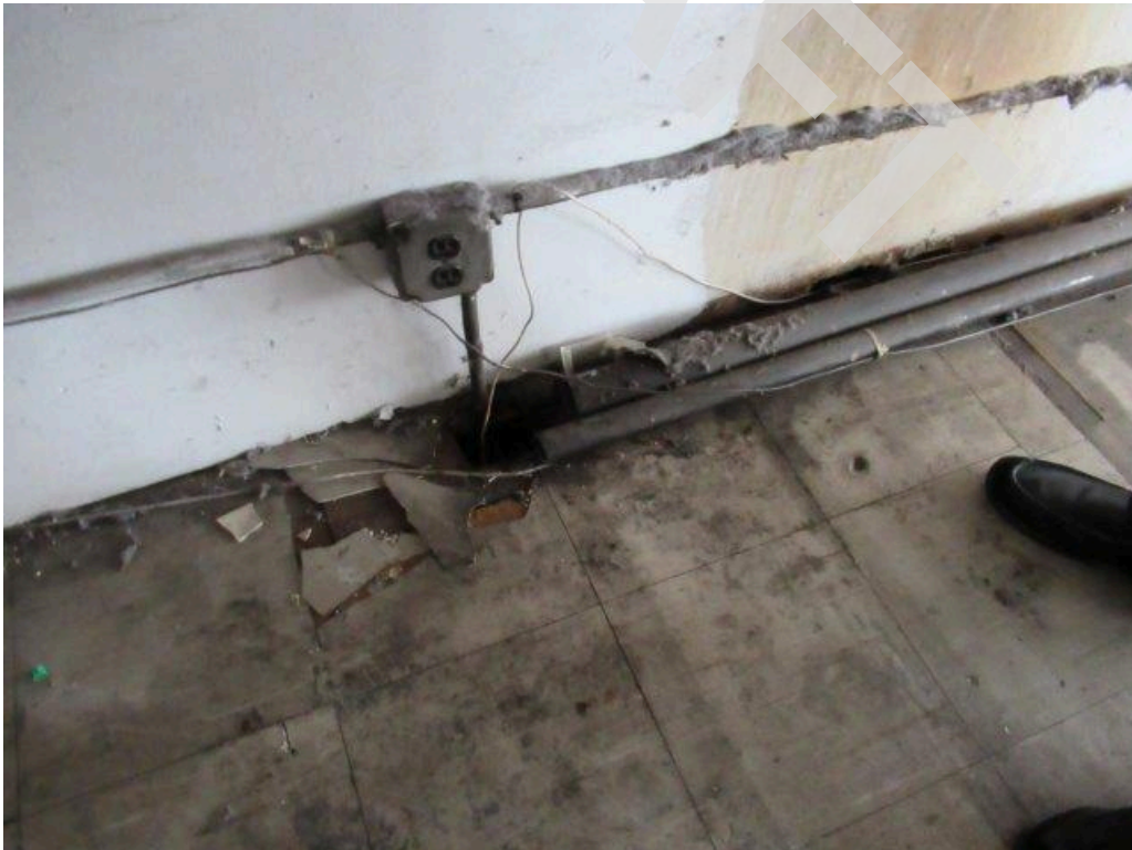
View of cut fill and vent lines to former AST
