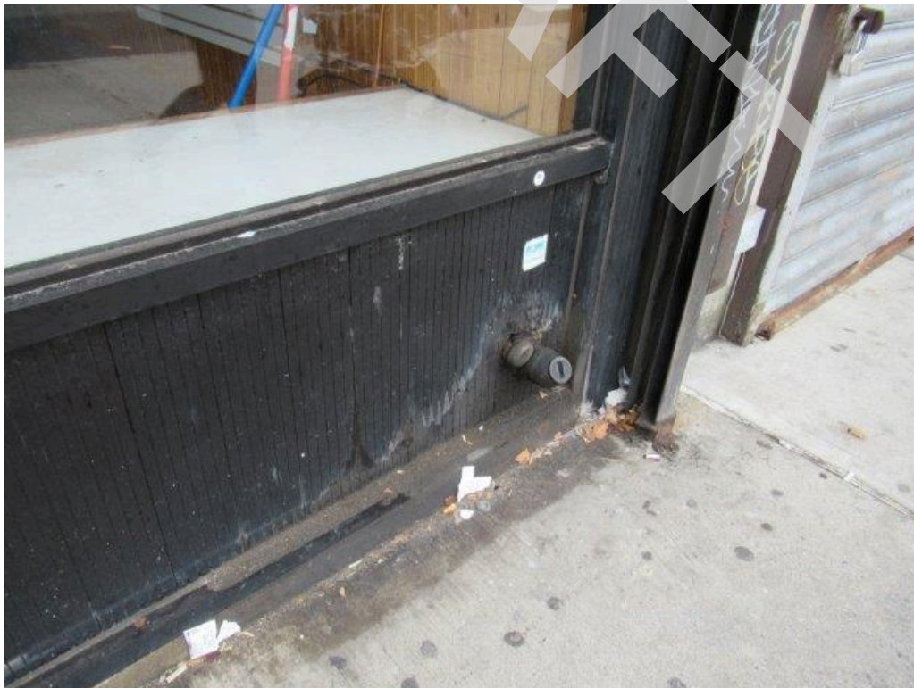
Fill and vent port for former oil AST
