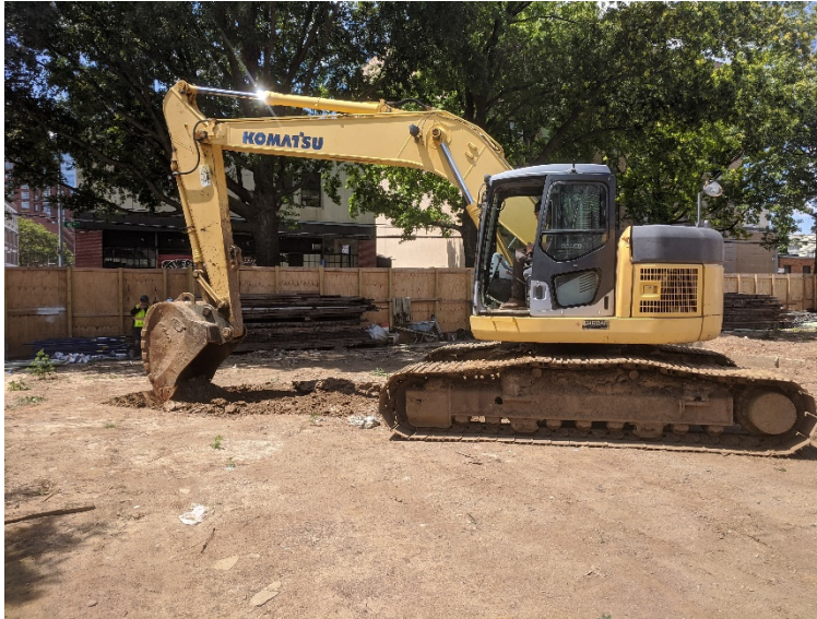
Photo 5, View of TP-1 being excavated.
