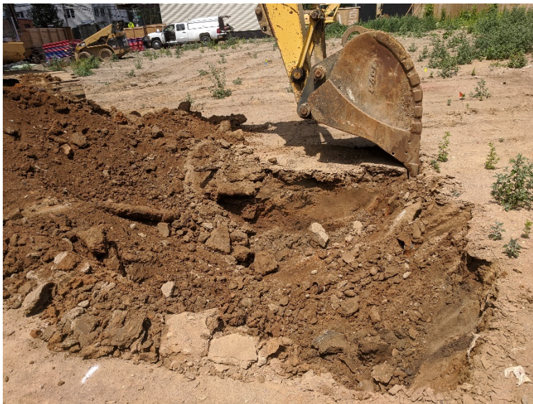
Photo 9, View of TP-2 being excavated.
