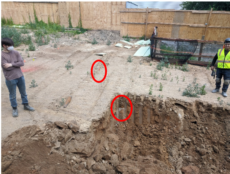
Photo 11, View of the discolored soil from TP-2 existing near the delineation soil boring area SB-102.
