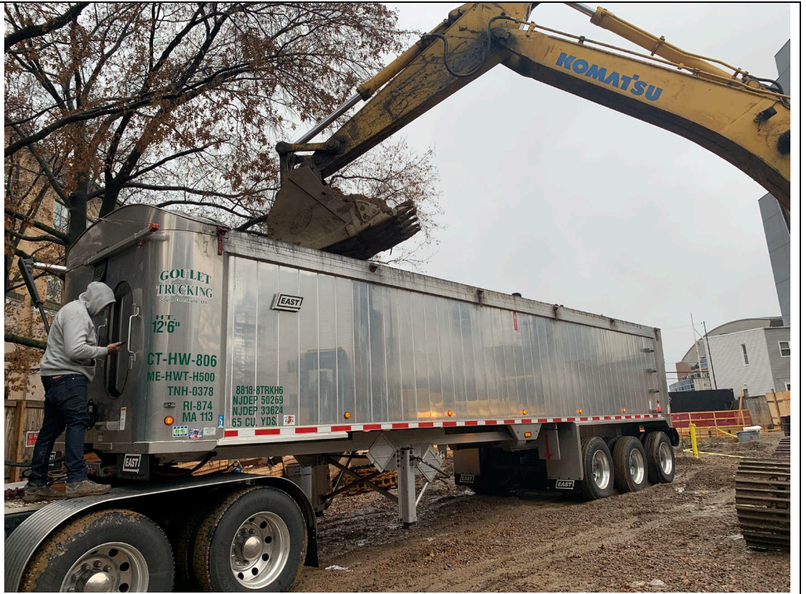
Photo 3 – View of second truck being loaded with hazardous waste from Quadrant 5
