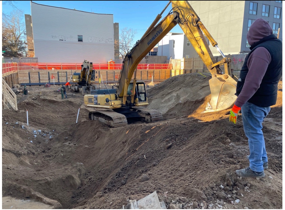
Photo 5 – View of excavator being used to create ramp on Quadrant 5
