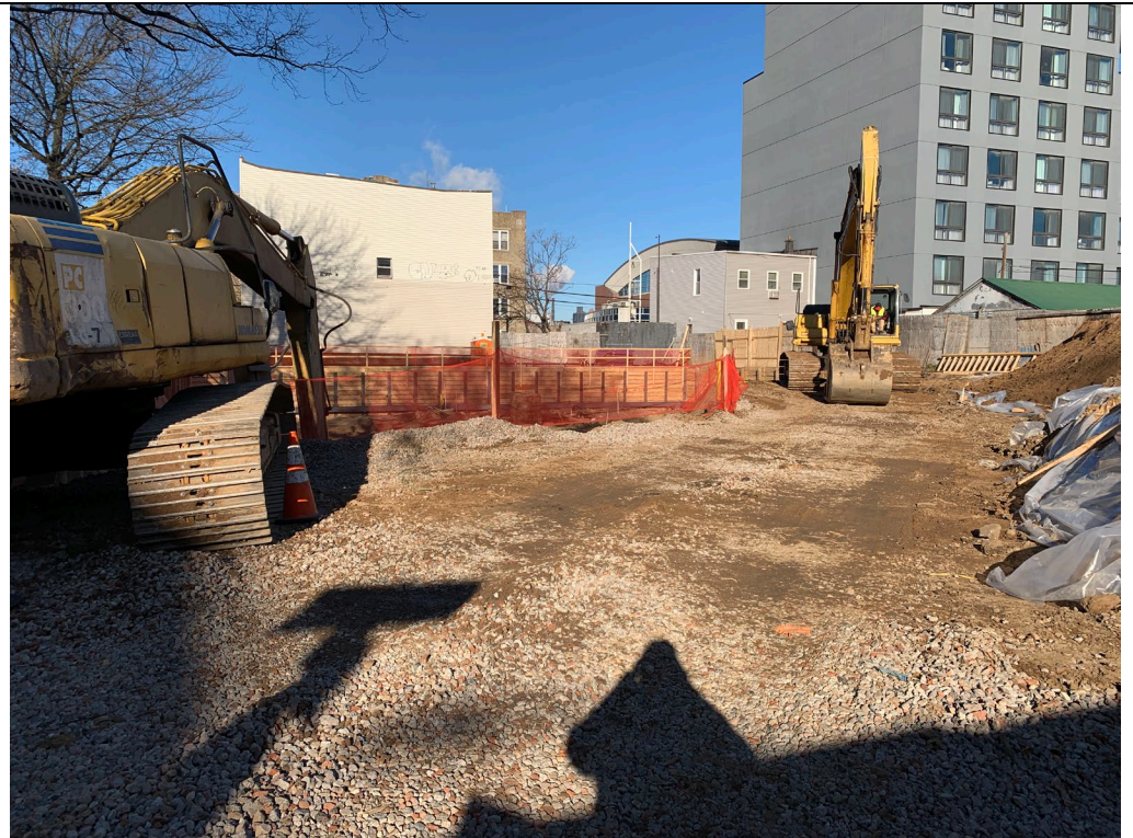
Photo 2 – View of the job site from the southeasterly entrance
