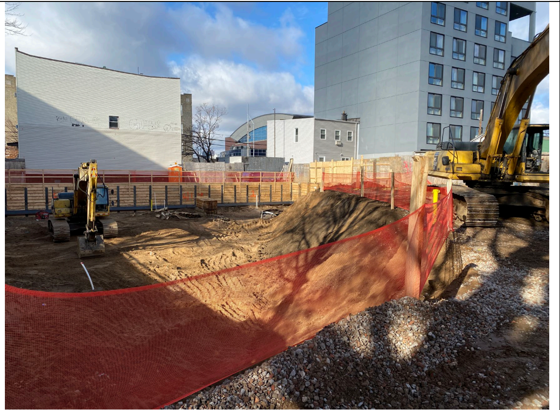
Photo 4 – View of the site facing west at end of day
