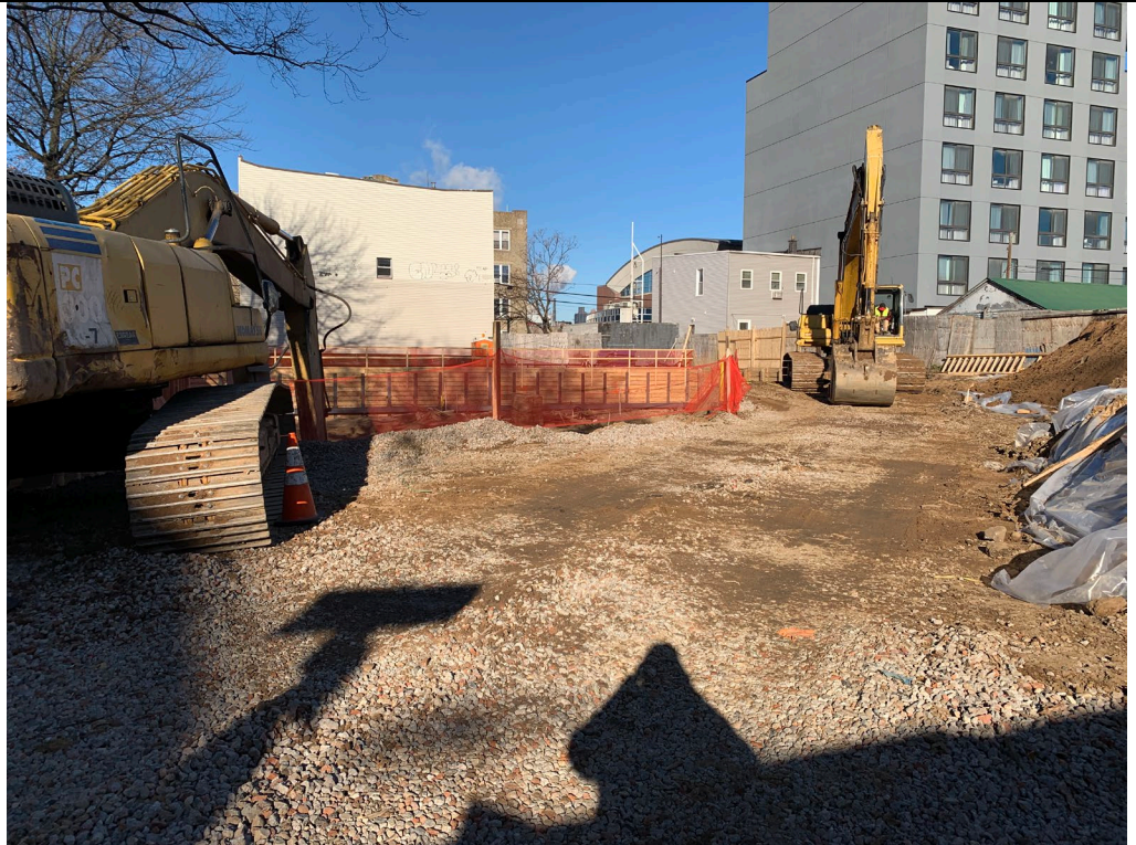
Photo 2 – View of the site facing west at end of day
