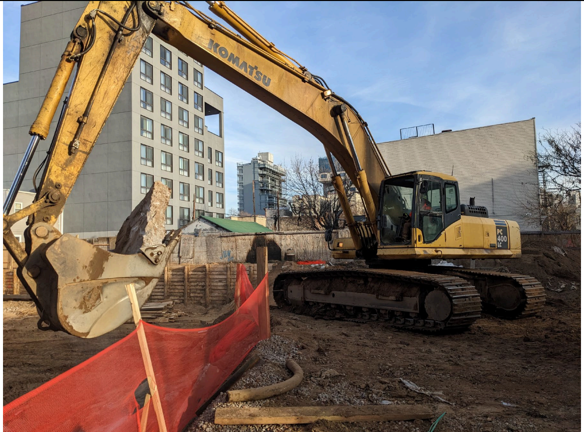
Photo 2 – View of excavator loading concrete debris, facing north
