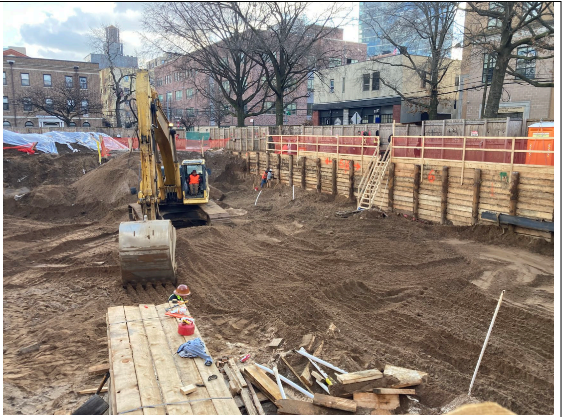
Photo 3 – View of the site at the end of day, facing east
