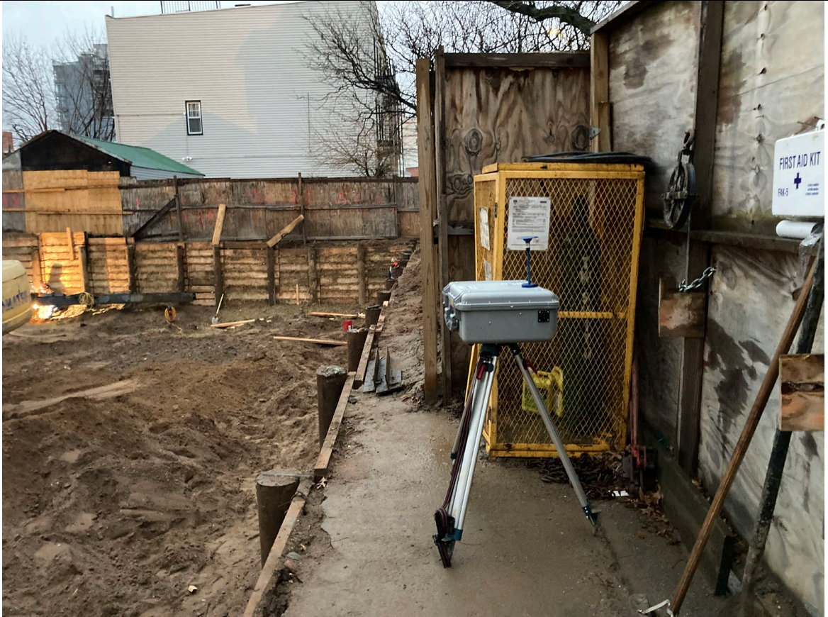
Photo 1 – View of welding being performed near the the Downwind CAMP unit
