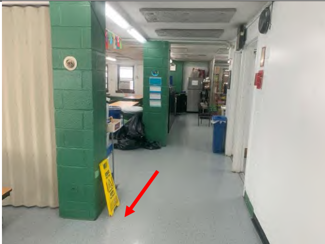
Proposed suction point (SP-1) location with one vacuum monitoring point (VMP) beneath the window on the western side of the cafeteria
