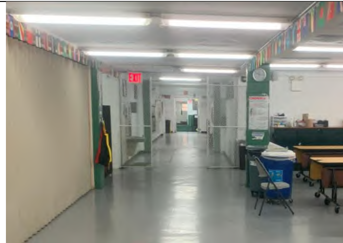
Proposed Pipe pathway from SP-5 to SP-1 and SP-3 connection along ceiling with VMP behind gate
