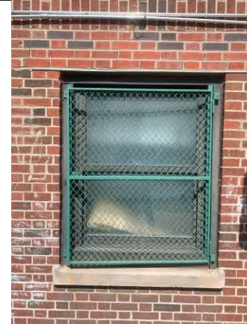
Window with grate that will be partially removed for SSDS piping pathway
