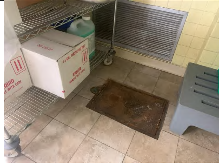
Hatch in southeast corner of kitchen near proposed SP-5
