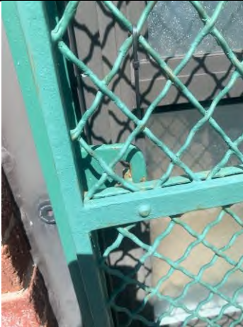
Window grate material to be cut for SSDS piping pathway
