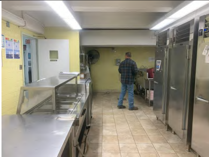
Proposed piping along ceiling in the kitchen
