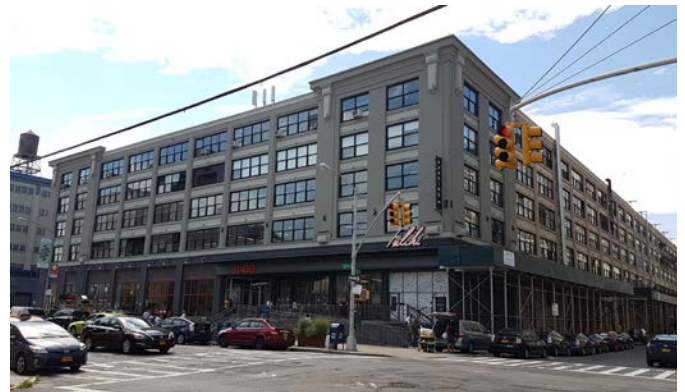
The Falchi Building in the LIC Industrial Business Zone, east of Sunnyside Yards
