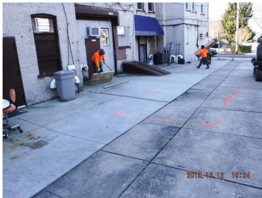
Photograph 2: Outline of the UST in red spray paint as established by the GPR survey. Photographer facing west.
