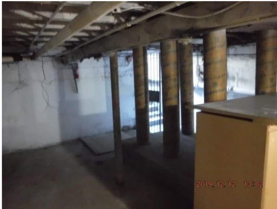
Photograph 3: View of Sump1 in the basement of 161-03 29 th Avenue (sump is under plywood cover at background). Support posts for former dry cleaning machine visible at right.
