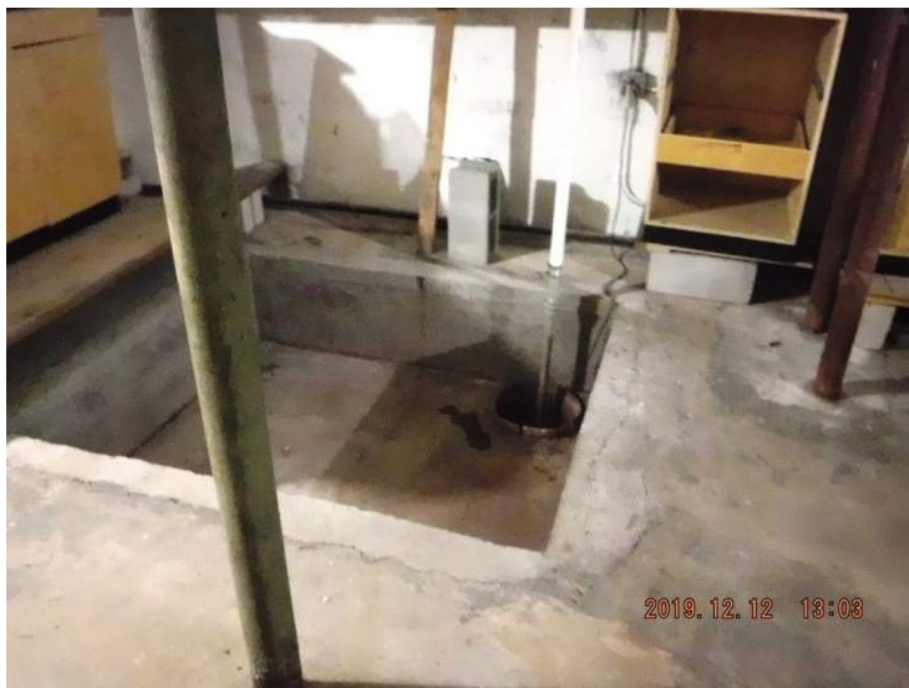
Photograph 4: Sump2 in the basement of 161-03 29 th Avenue.
