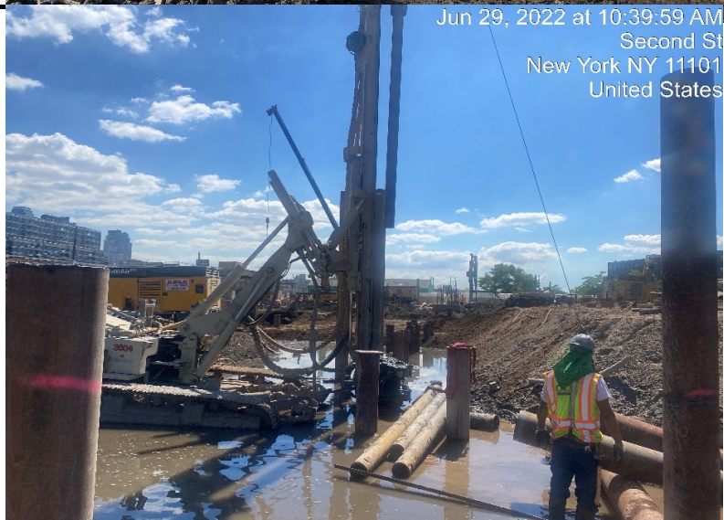
Photograph 3 - Civetta continues drilling caissons, view facing east.
