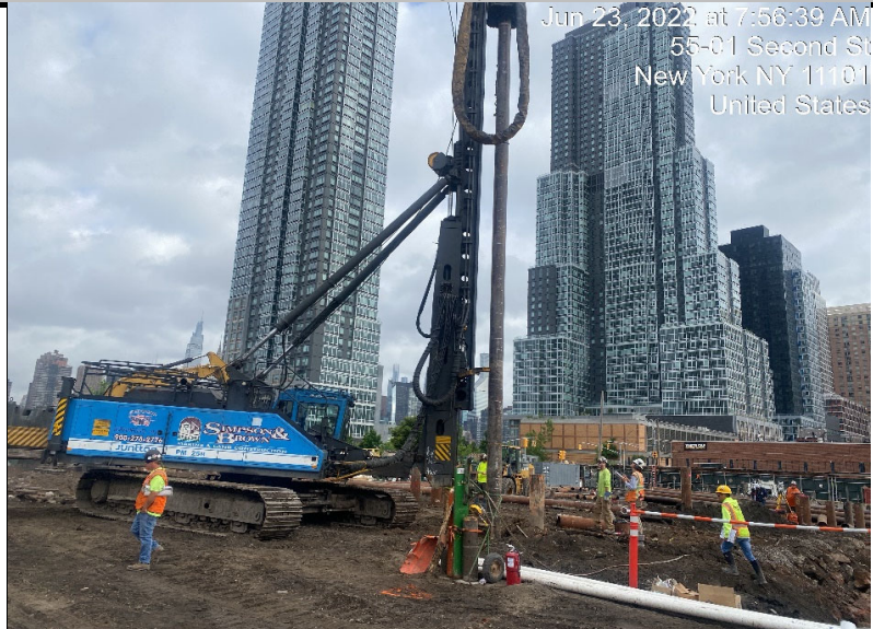
Photograph 1 - Civetta drives piles, view facing northwest.
