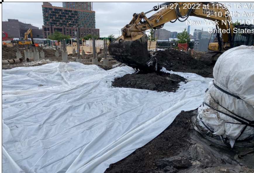
Photograph 2 - Soil with apparent petroleum staining and odors stockpiled on-site, which was covered with plastic sheeting at the end of the day. View facing west.
