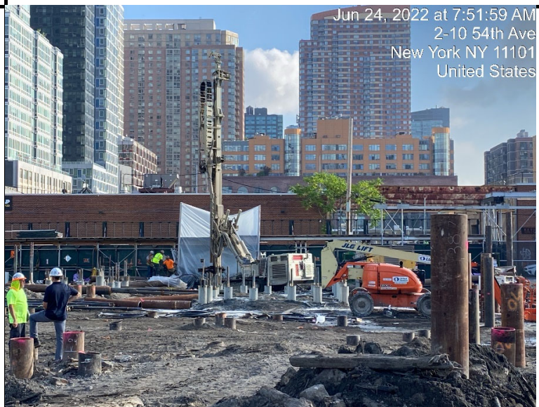
Photograph 3 - Civetta continues drilling caissons, view facing north.
