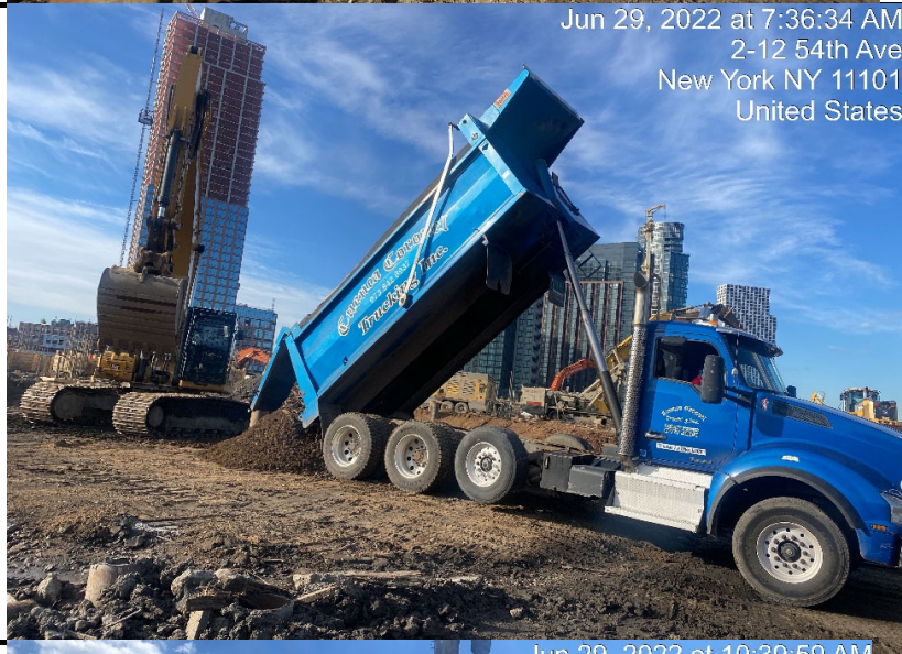
Photograph 2 - Civetta imports approved fill, view facing southeast.
