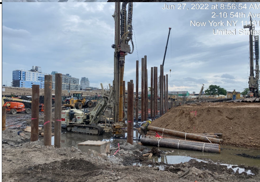
Photograph 3 - Civetta continues drilling caissons, view facing north.
