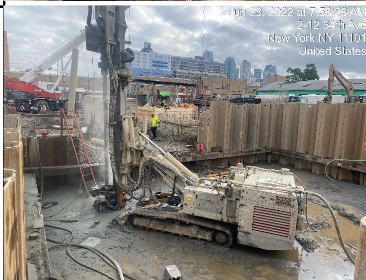
Photograph 3 - Civetta continues drilling tie downs, view facing northeast.
