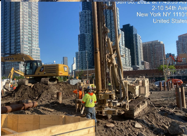
Photograph 3 - Civetta continues drilling caissons, view facing northeast.
