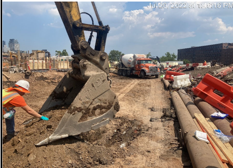
Photograph 1 - AKRF takes end point soil samples in WC-19, view facing east.
