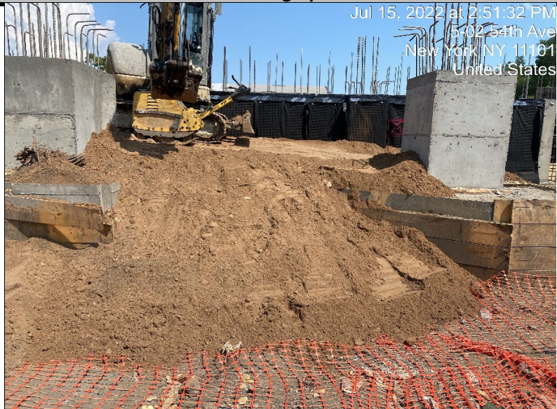
Photograph 1 - Civetta grades imported fill in Grid WC-08, view facing east.
