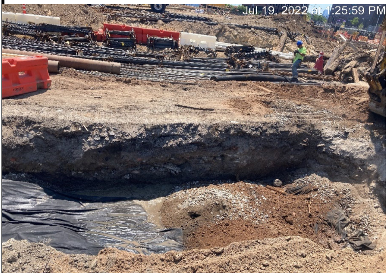
Photograph 2 - Civetta lays down demarcation barrier before backfilling in petroleum treatment area, view facing south.
