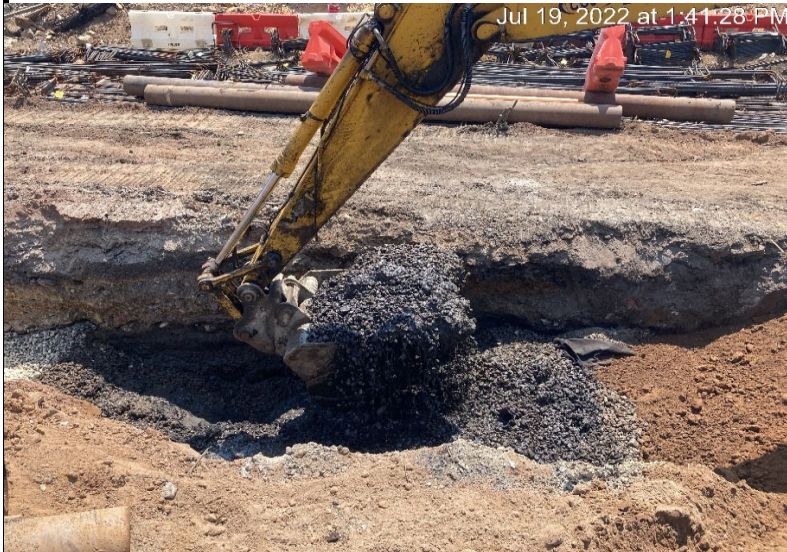
Photograph 1 - Civetta mixes Regenesis Persuflox and ORC in petroleum treatment area with imported gravel, view facing south.
