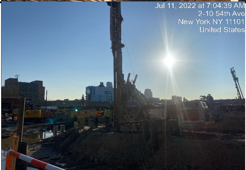
Photograph 3 - Civetta continues drilling caissons, view facing east.
