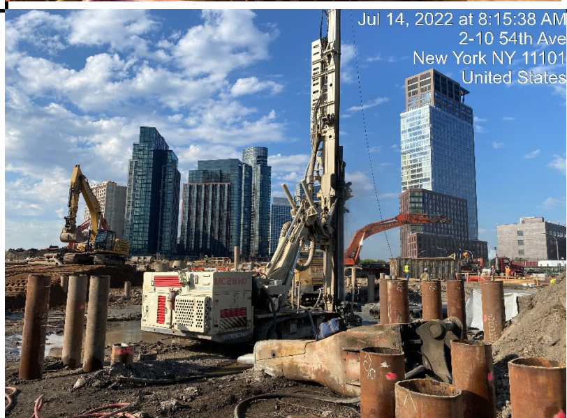
Photograph 3 - Civetta continues drilling caissons, view facing south.
