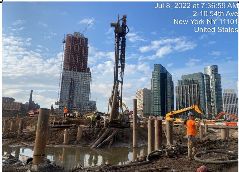
Photograph 3 - Civetta continues drilling caissons, view facing south.
