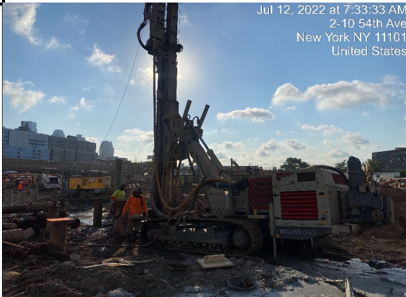
Photograph 3 - Civetta continues drilling caissons, view facing east.
