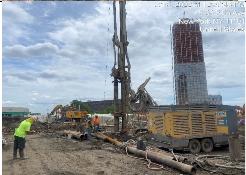
Photograph 3 - Civetta continues drilling caissons, view facing east.
