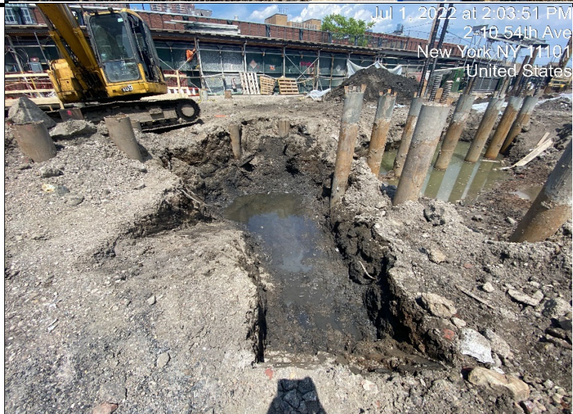
Photograph 2 - Excavated UST grave from USTs, view facing north.
