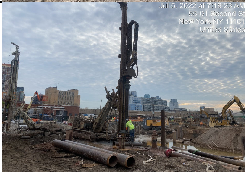
Photograph 3 - Civetta continues drilling caissons, view facing northeast.
