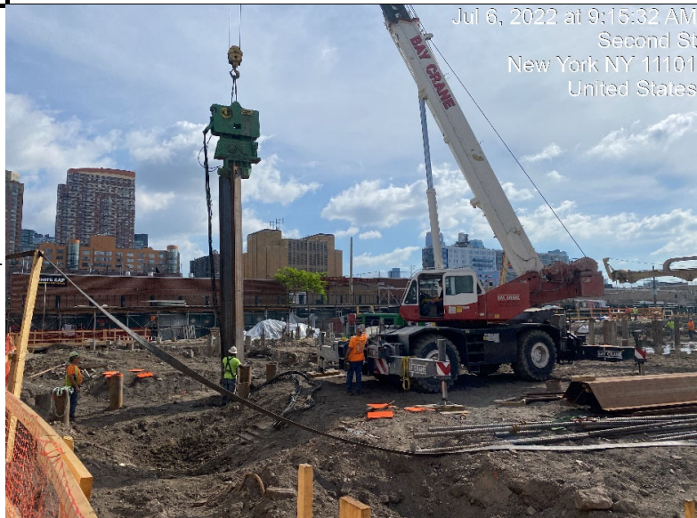
Photograph 2 - Civetta drives sheeting in Grid WC- 09, view facing north.
