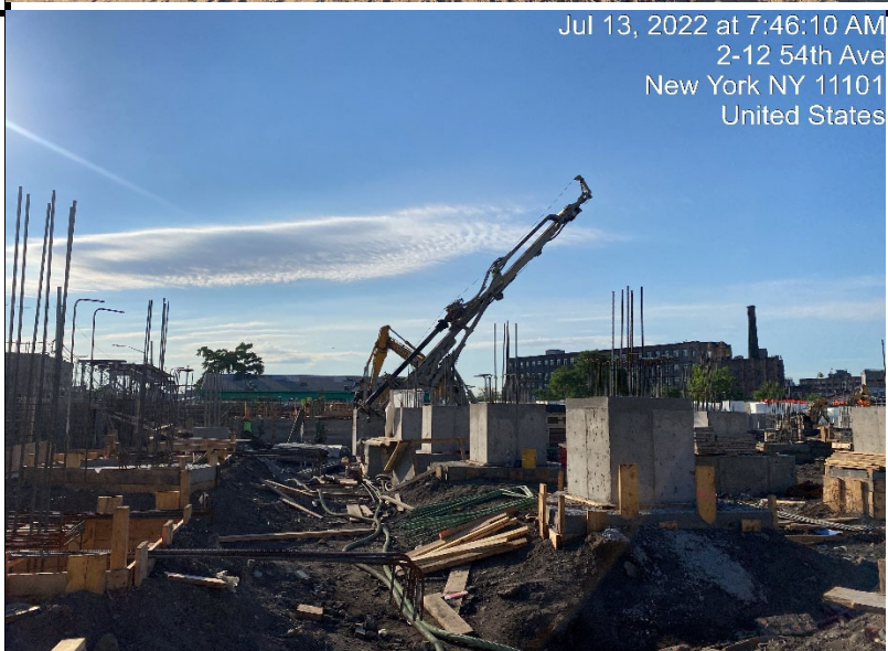
Photograph 3 - Civetta continues drilling caissons, view facing east.
