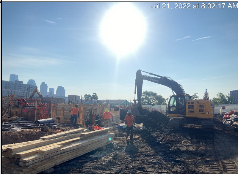
Photograph 3 - Civetta backfills around pile caps, view facing east.
