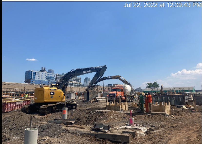
Photograph 3 - Civetta pours concrete and backfills around pile caps, view facing east.
