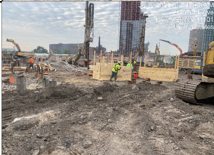
Photograph 2 - Civetta continues pile cap form installation, view facing southeast.
