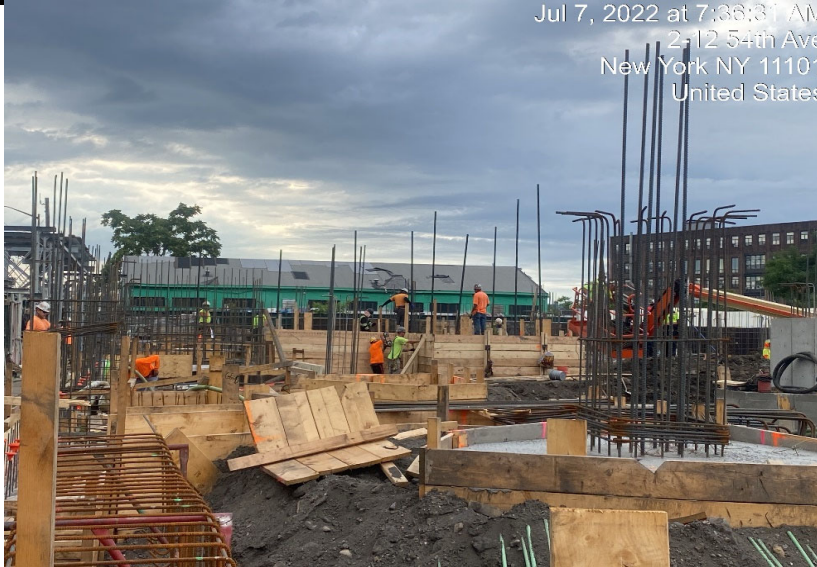
Photograph 1 - Civetta continues installing rebar for foundation elements, view facing east.
