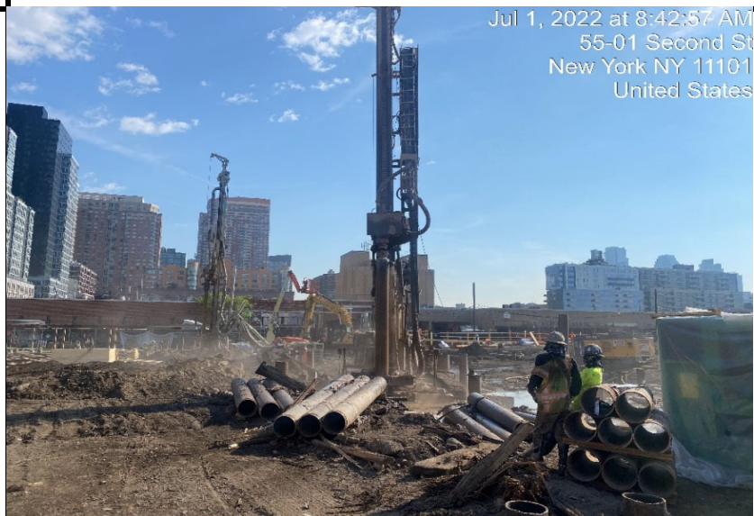
Photograph 3 - Civetta continues drilling caissons, view facing northeast.
