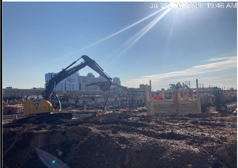
Photograph 1 - Civetta moves equipment for installation of pile cap molds, view facing northeast.
