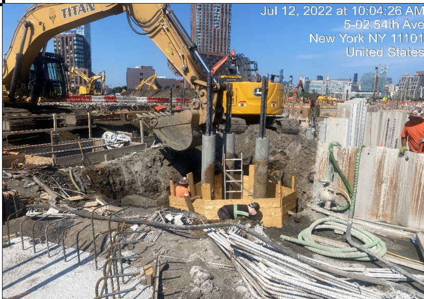
Photograph 2 - Civetta continues installing pile cap forms, view facing west.
