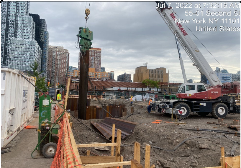
Photograph 2 - Civetta drives sheeting in Grid WC- 09, view facing north.
