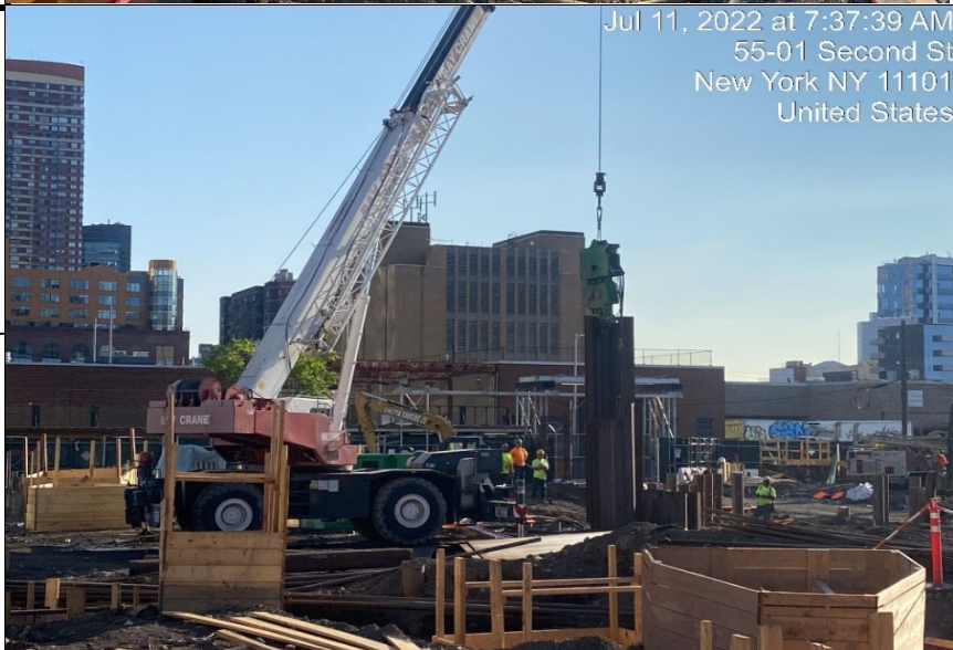
Photograph 2 - Civetta drives sheeting in Grid WC- 10, view facing north.
