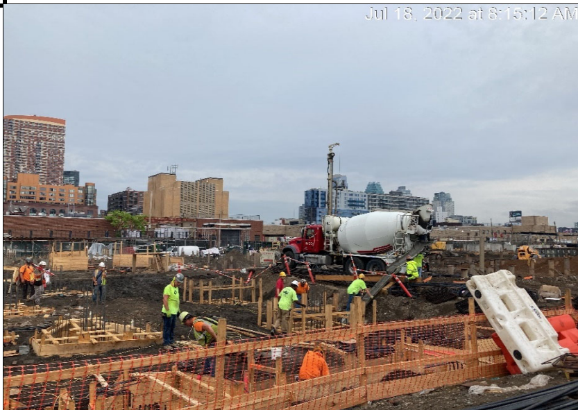
Photograph 3 - Civetta installs forms and pours concrete, view facing northeast.
