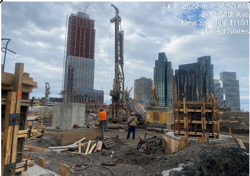
Photograph 3 - Civetta continues drilling caissons, view facing south.
