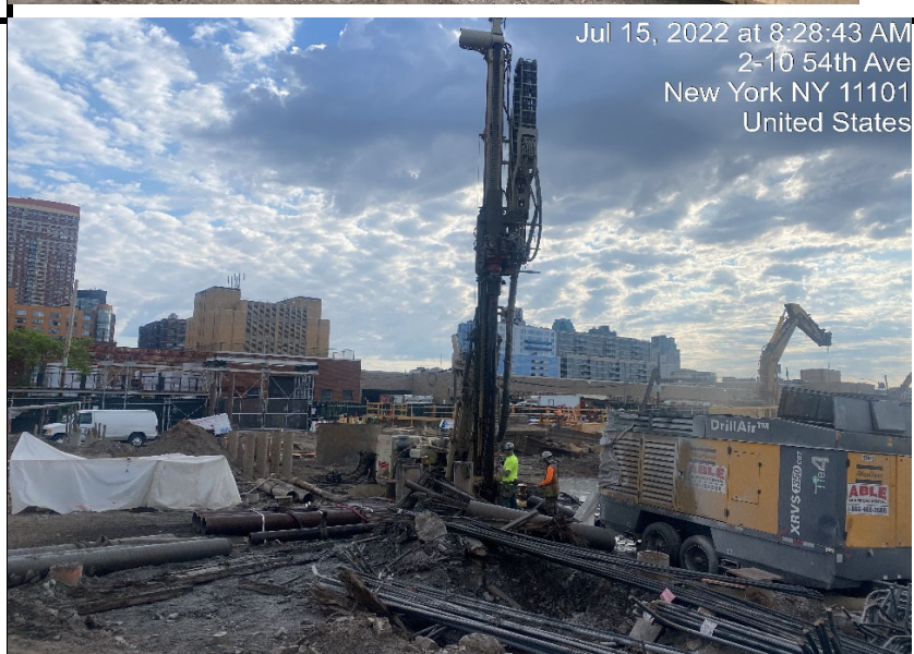
Photograph 3 - Civetta continues drilling caissons, view facing northeast.
