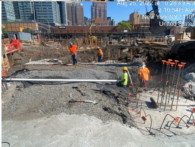
Photograph 2 - Installation of SSDS piping, view facing north.
