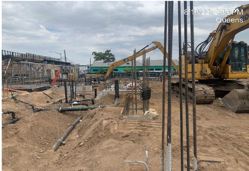
Photograph 2 - General fill graded over WC-07, WC-08. View facing east.
