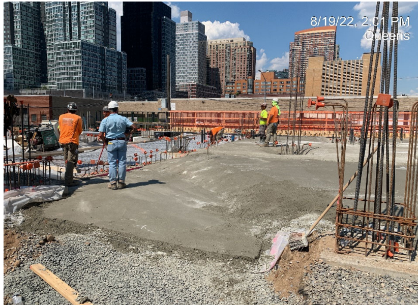
Photograph 2 -Mud slab poured in WC- 07.
