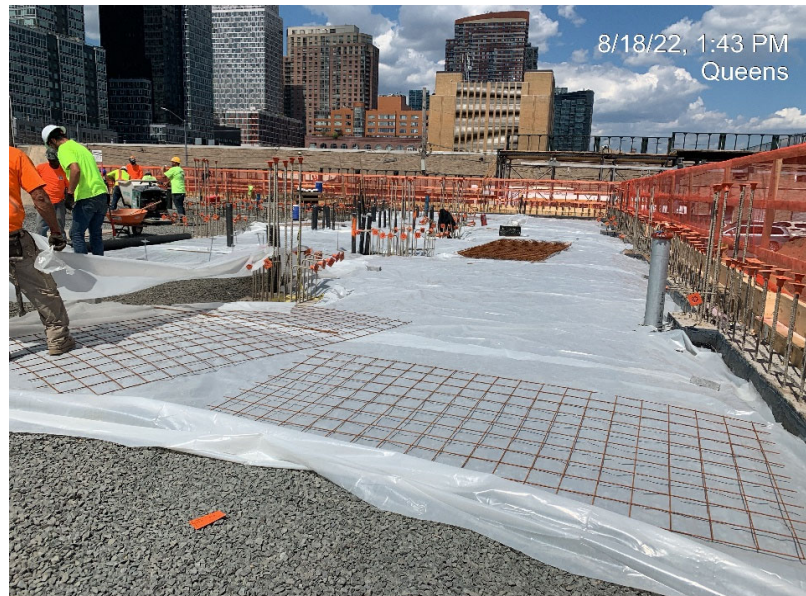
Photograph 2 - Vapor barrier install in WC-08.
