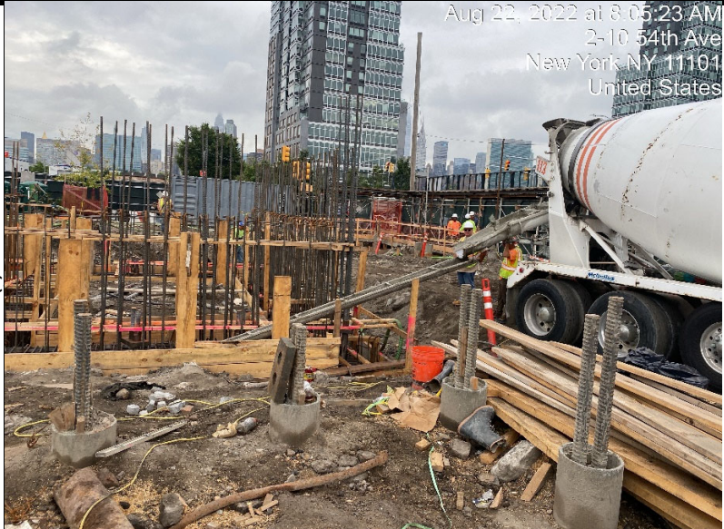
Photograph 1 - Pouring concrete for foundation element in Grids WC 01/02, view facing south.
