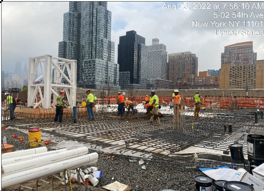
Photograph 2 - Installation of rebar and waterproofing, view facing northwest.
