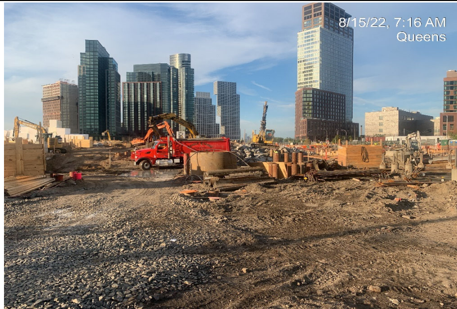
Photograph 2 - Civetta importing 3/4" stone to WC- 10. View facing south.
