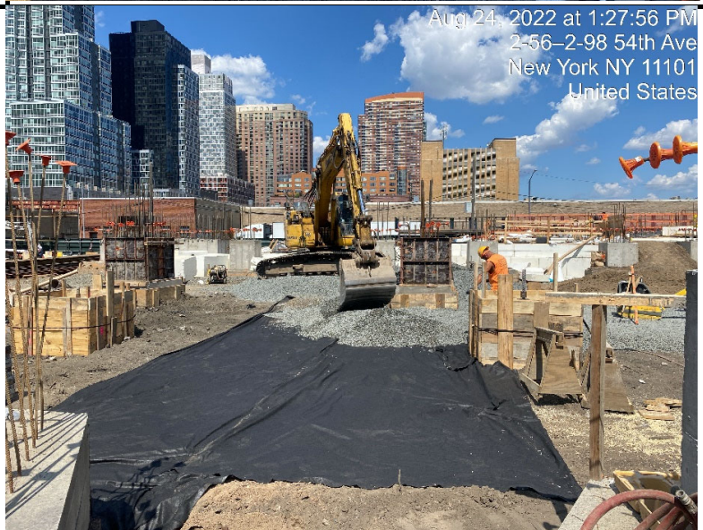
Photograph 2 - Installation of geotextile and stone, view facing north.
