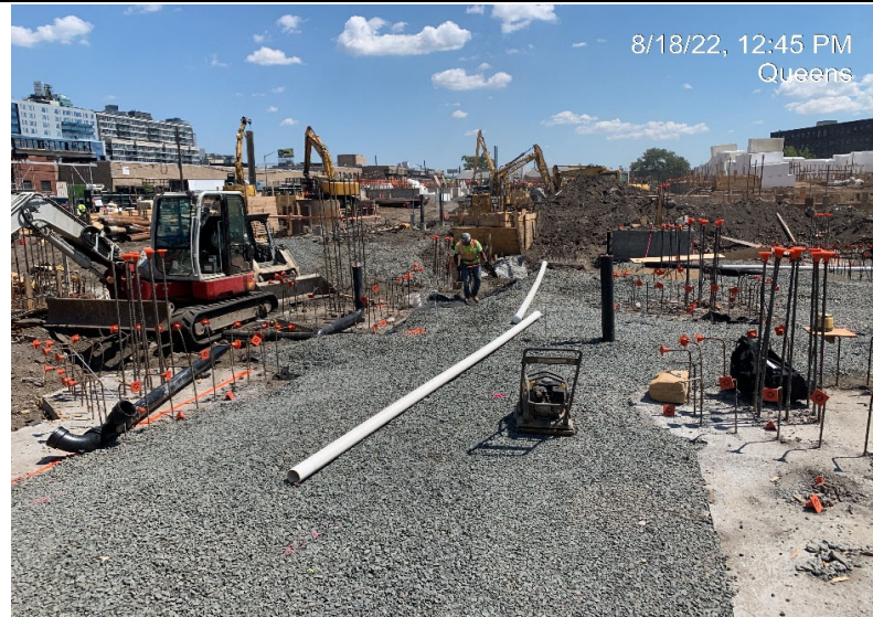
Photograph 1 - SSDS install in WC-09.
