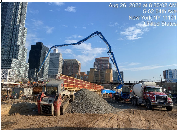
Photograph 3 - Concrete pour of foundation slab, view facing north.
