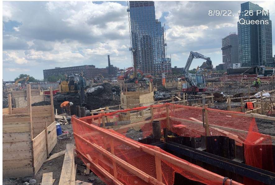
Photograph 2 - Civetta inserts pile cap forms WC-02. View facing southeast.
