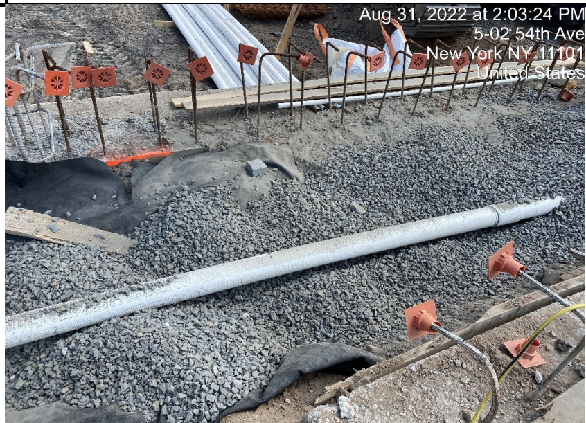
Photograph 2 - Installation of SSDS piping, view facing west.
