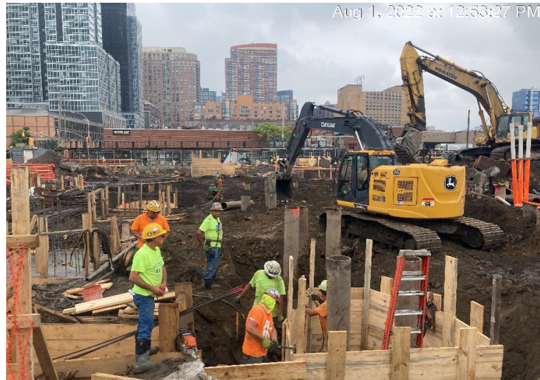
Photograph 1 - Civetta installs pile cap molds in WC-09, view facing north.
