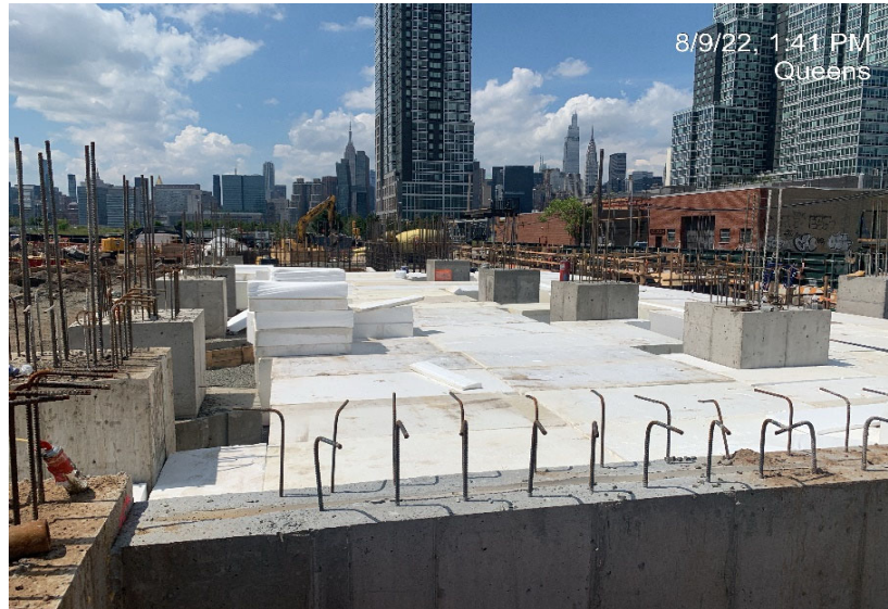
Photograph 1 - Styrofoam blocks installed in WC-05, WC-06. View facing West.
