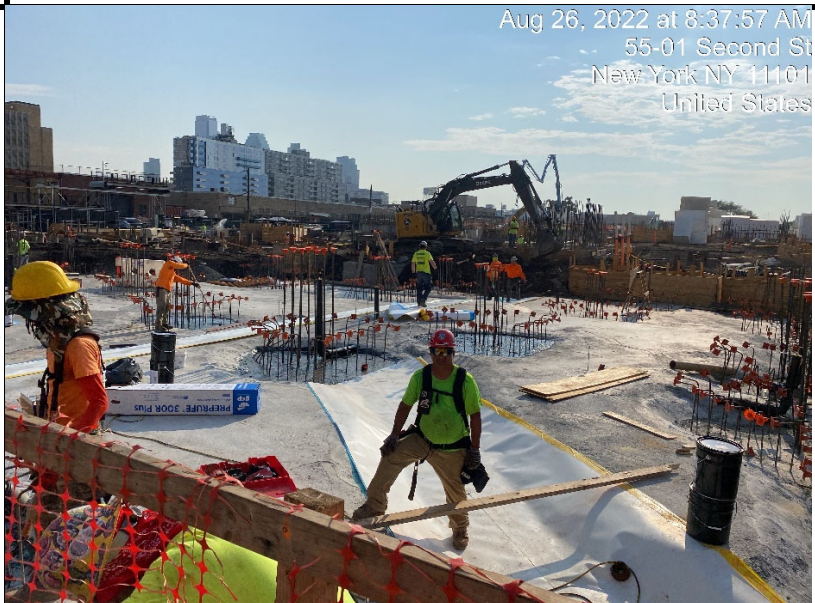
Photograph 2 - Installation of waterproofing, view facing northeast.
