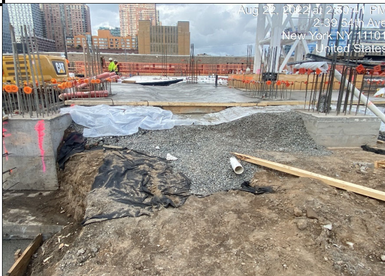
Photograph 3 - Installation of mud slab and SSDS piping, view facing north.
