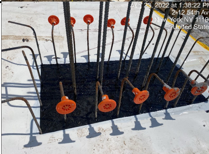
Photograph 3 - Waterproofing installation.
