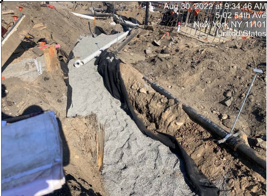
Photograph 2 - Installation of SVE piping, view facing northwest.
