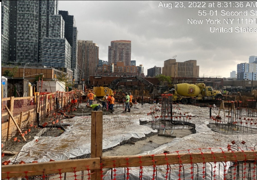
Photograph 1 - Pouring concrete for mud slab in Grids WC-09/10, view facing north.
