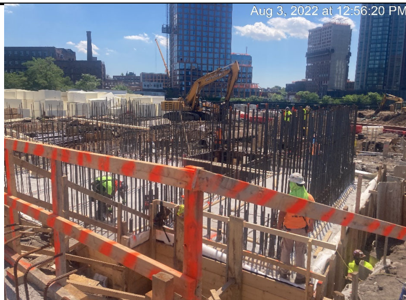
Photograph 2 - Civetta installs rebar formwork, view facing south.
