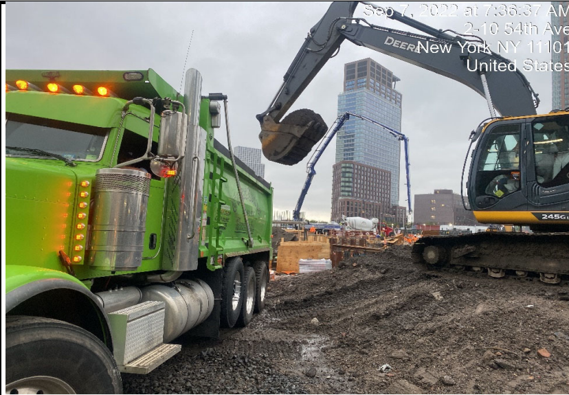
Photograph 1 - Export of soil from Grid WC-02, view facing southeast.
