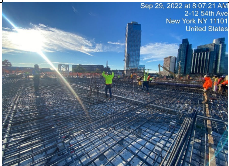
Photograph 3 - Rebar installation, view facing southeast.
