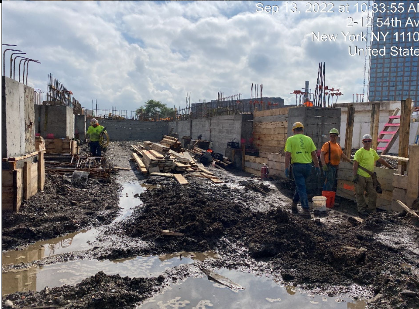
Photograph 2 - Rebar installtion, view facing east.
