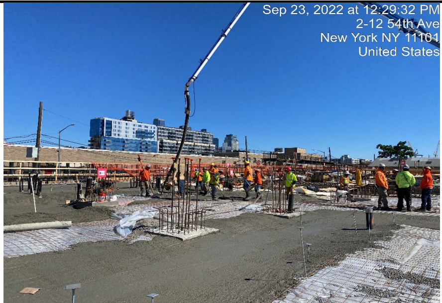
Photograph 2 - concrete pour of the mud slab, view facing northeast.
