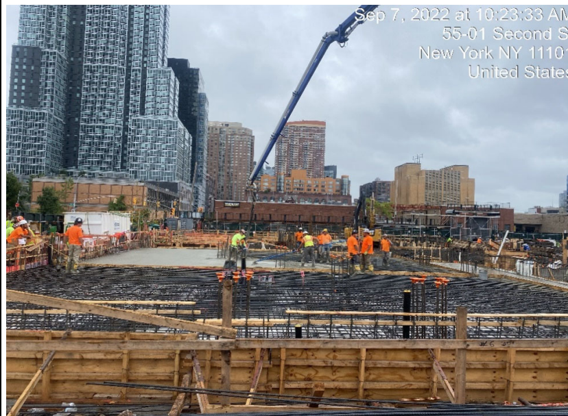
Photograph 2 - Concrete pour of foundation slab in Grid WC-09, view facing north.
