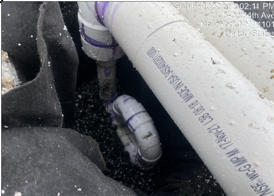
Photograph 2 - Installation of SSDS piping, view facing east.
