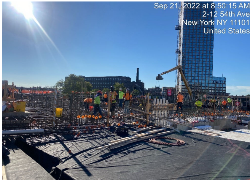
Photograph 2 - Rebar installation, view facing southeast.
