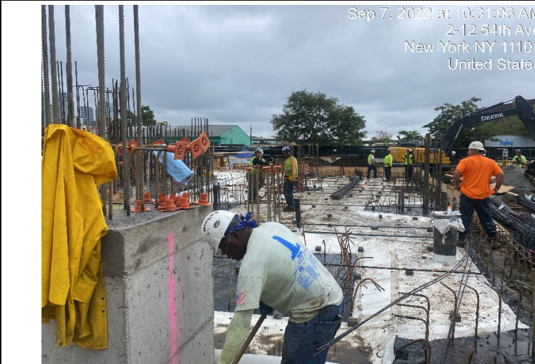
Photograph 3 - Rebar installation in Grid WC-16, view facing east.
