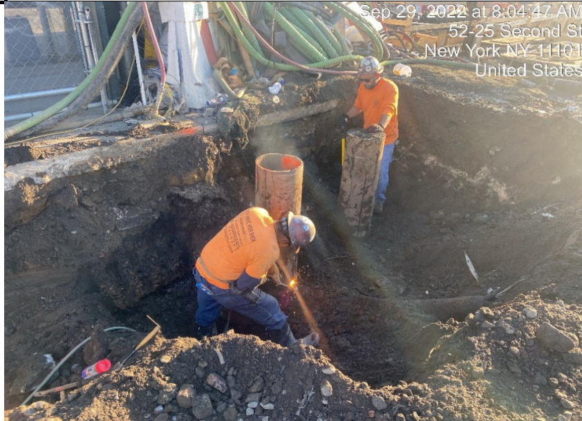
Photograph 2 - Cutting piles in Grid WC-03, view facing northeast.
