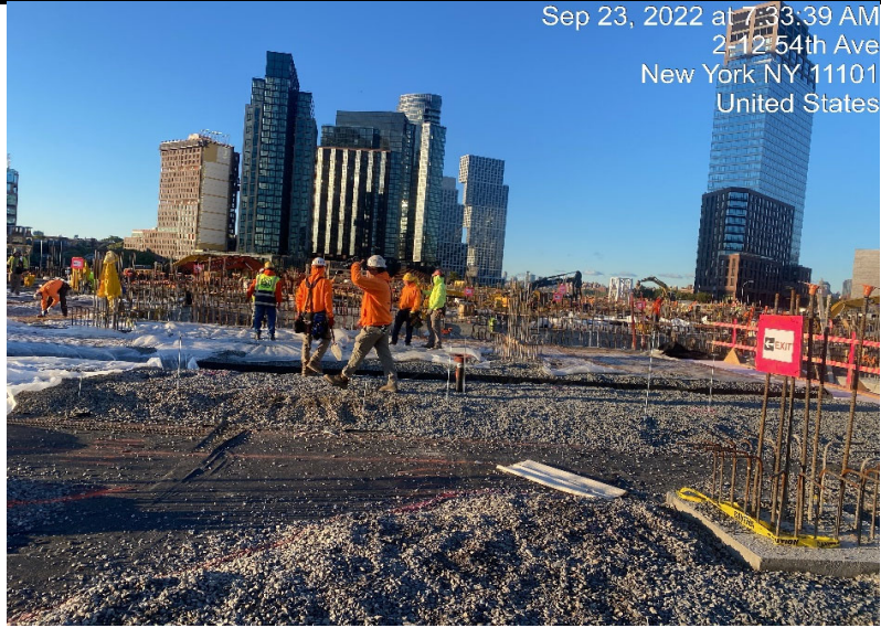
Photograph 1 - Vapor barrier and rebar installation, view facing south.
