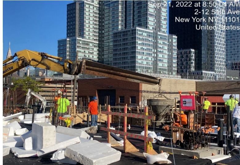
Photograph 1 - Concrete pour of foundation element, view facing northwest.
