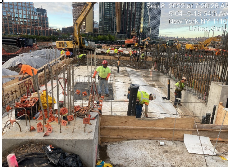
Photograph 3 - Rebar installation in Grid WC-16, view facing south.
