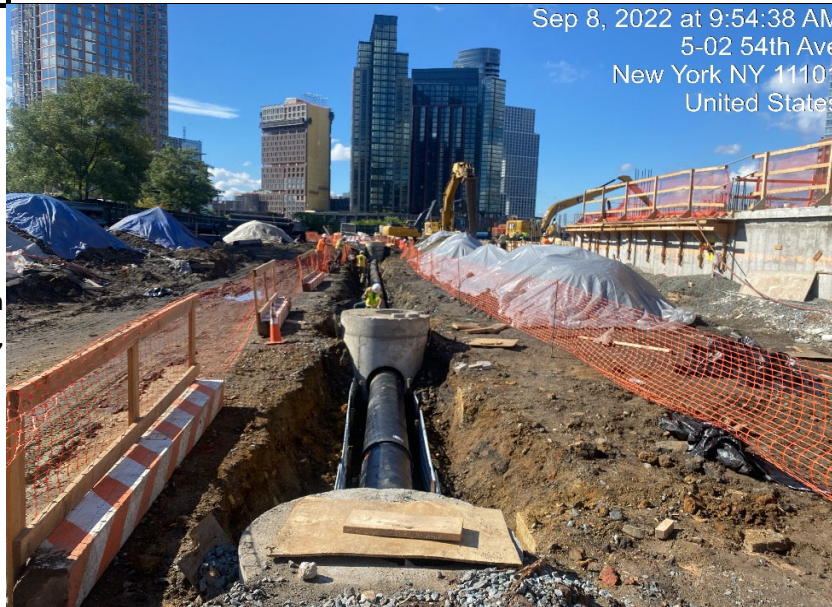
Photograph 2 - Dubner's installation of the sewer system, view facing south.
