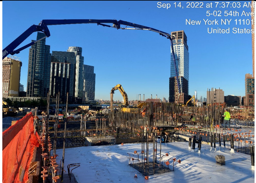
Photograph 2 - Concrete pour of foundation slab in Grid WC-16, view facing southwest.
