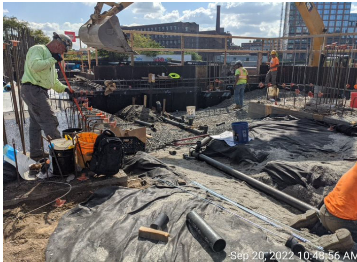
Photograph 3 - Plumbing & waterproofing adjacent to installed pipe, view facing southeast.
