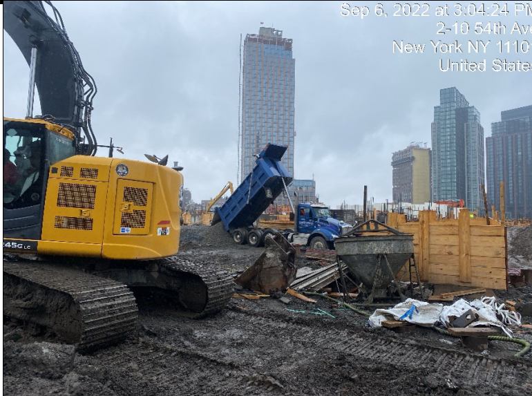
Photograph 1 - Import of stone, view facing southwest.
