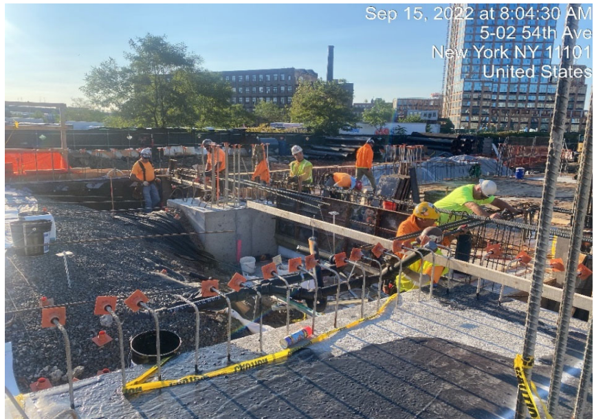
Photograph 2 - Rebar installation in Grid WC-16, view facing southeast.
