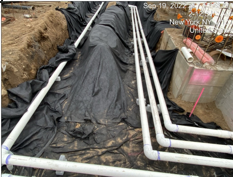
Photograph 2 - Installation of SVE piping, view facing west.
