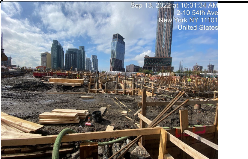
Photograph 3 - General view of the Site, view facing south.
