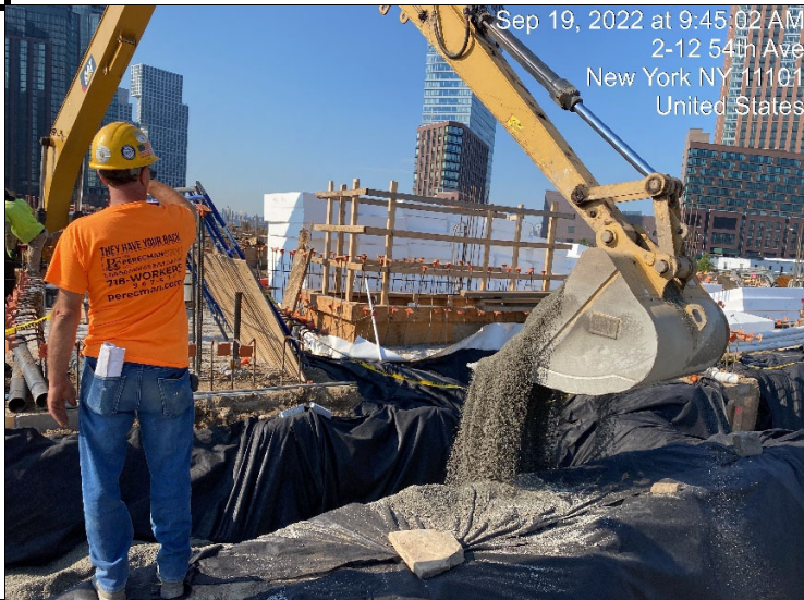
Photograph 3 - Installation of sand for the SVE system, view facing south.
