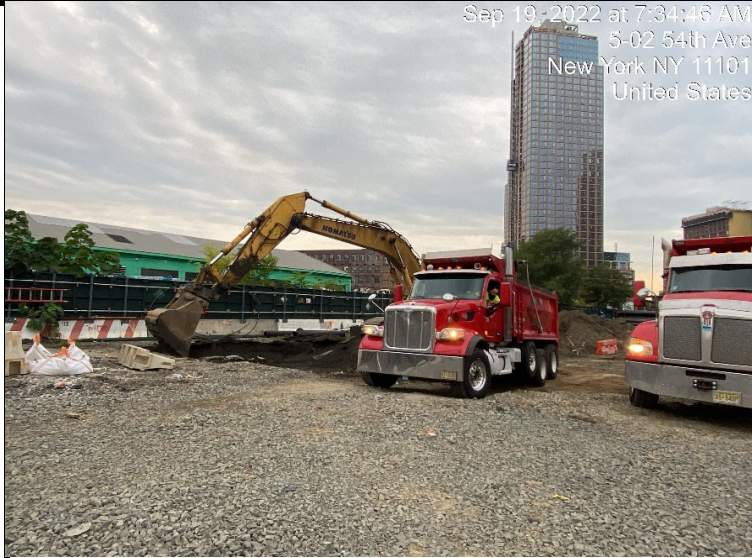
Photograph 1 - Export of soil from Grid WC-25 to Bayshore facility in Kearny, NJ, view facing southeast.
