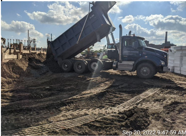
Photograph 2 - Import of stone, view facing east.
