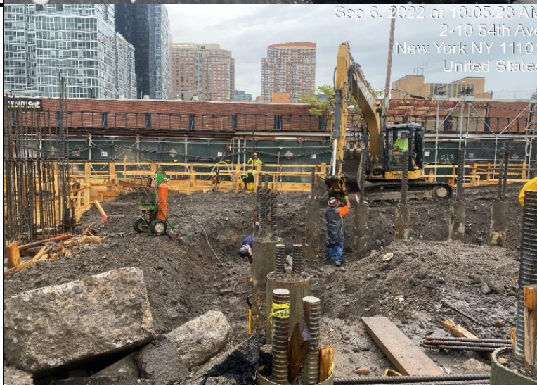
Photograph 3 - Excavation for foundation elements, view facing north.
