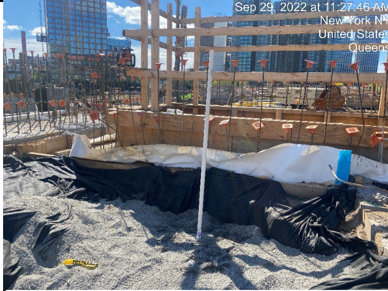
Photograph 1 - Installation of SVE monitoring point, view facing south.
