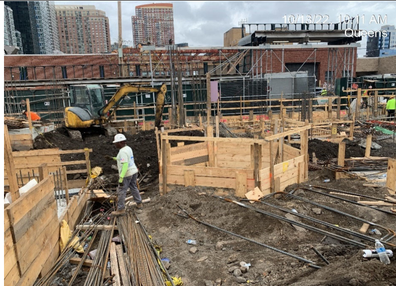
Photograph 1 - Excavation around pile cap forms in grid WC-02, and WC- 03. View facing north.
