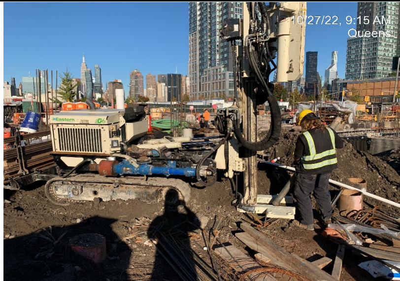
Photograph 1 - Eastern Environmental drilling MW-01, view facing west.
