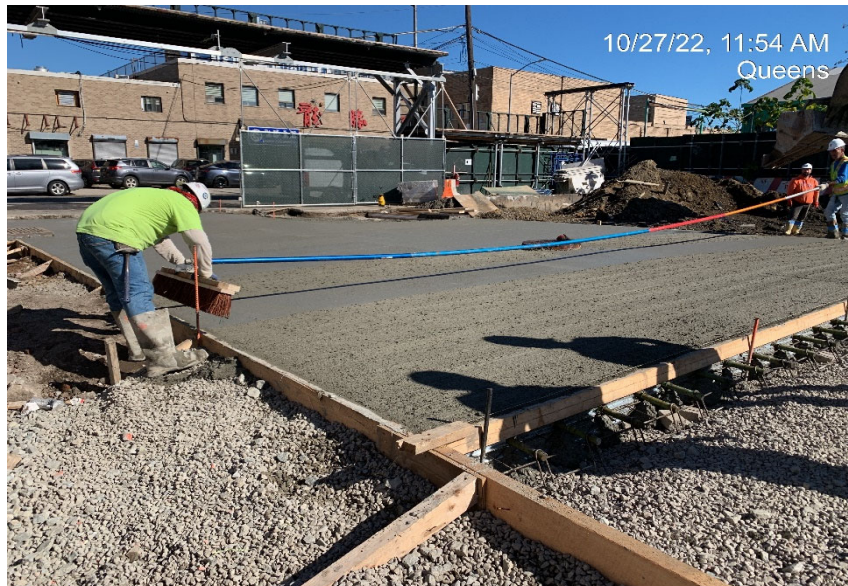
Photograph 2 - The landscaping contractor spreading concrete in WC-25, view facing northeast.
