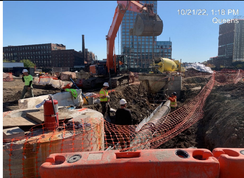
Photograph 1 - The landscaping contractor pouring concrete over the sewer pipes in grid WC-22, view facing southwest.
