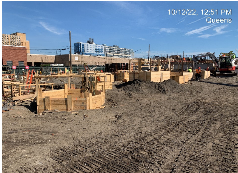
Photograph 2 - Pile cap form installation in WC-4, view facing northeast.
