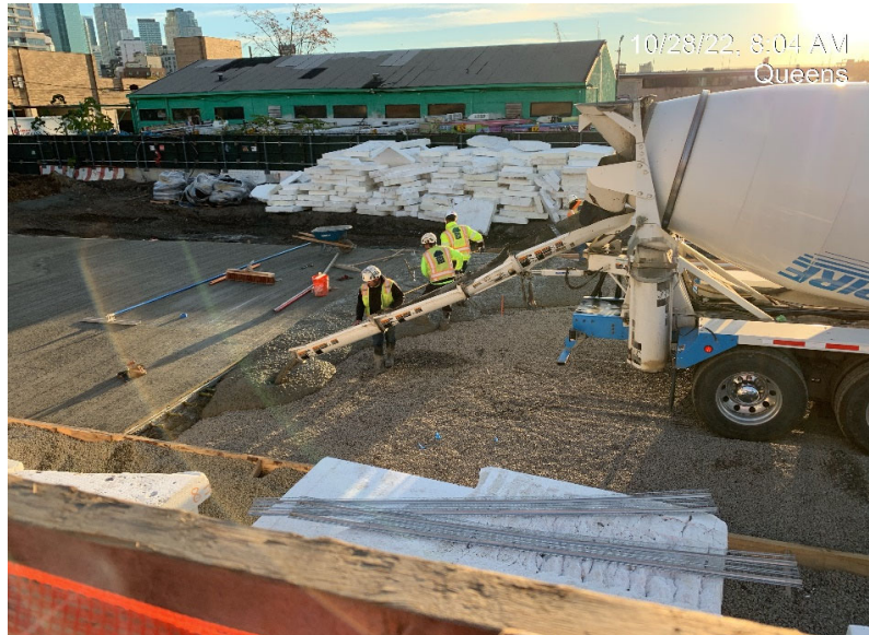
Photograph 2 - The landscaping contractor spreading concrete in WC-25, view facing northeast.
