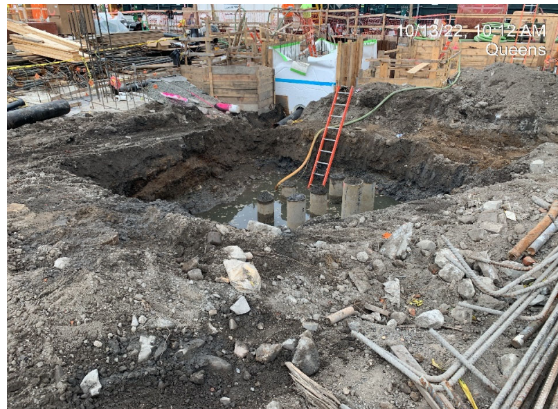
Photograph 2 - Excavation for pile cap, grid WC-01. View facing southwest.
