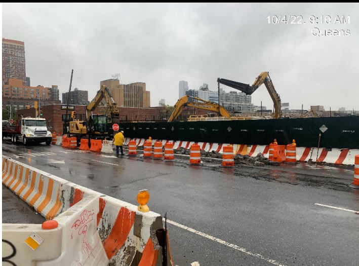
Photograph 3 - The landscaping crew breaks up the sidewalk to prep for a crane pad installation.
