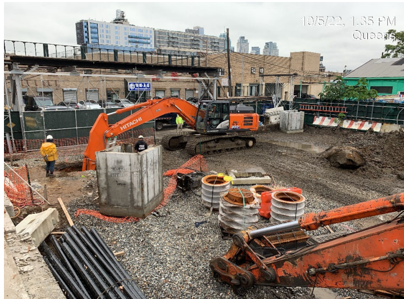
Photograph 2 - Landscaping crew excavates for installation of sewer system, view facing northeast.
