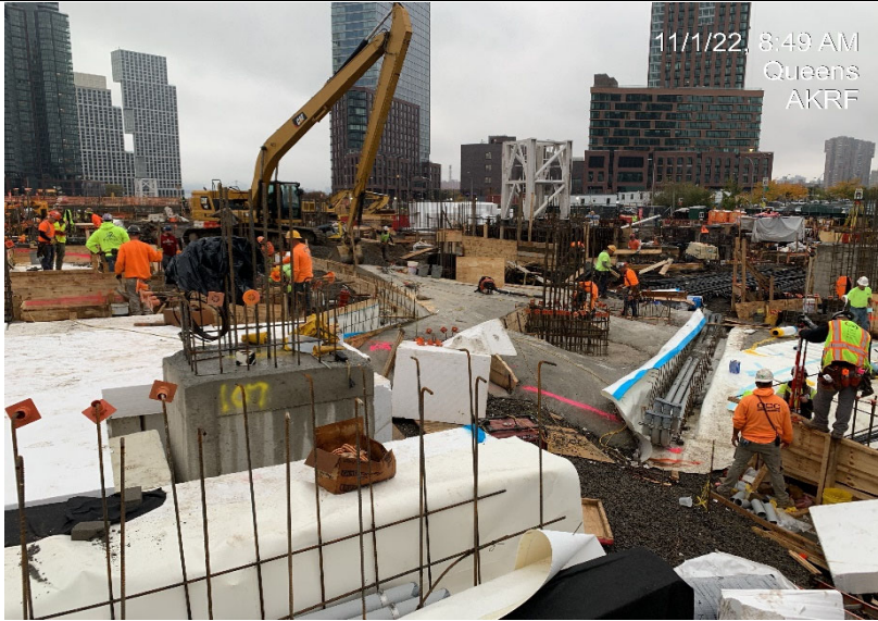
Photograph 1 - Civetta pouring concrete in WC-03.
