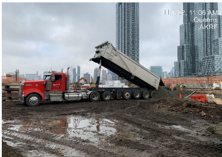
Photograph 3 - The landscaping contractor importing gravel to WC-21.
