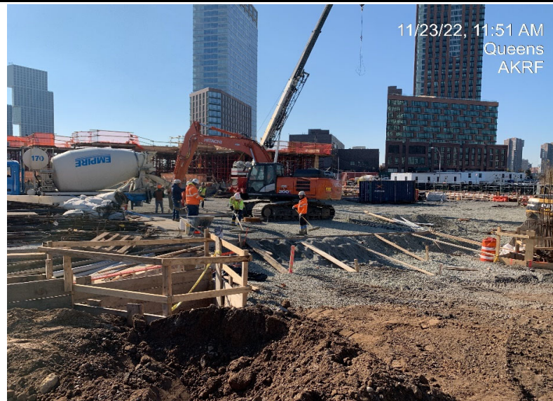
Photograph 2 - The landscaping contractor pouring concrete in WC-18.
