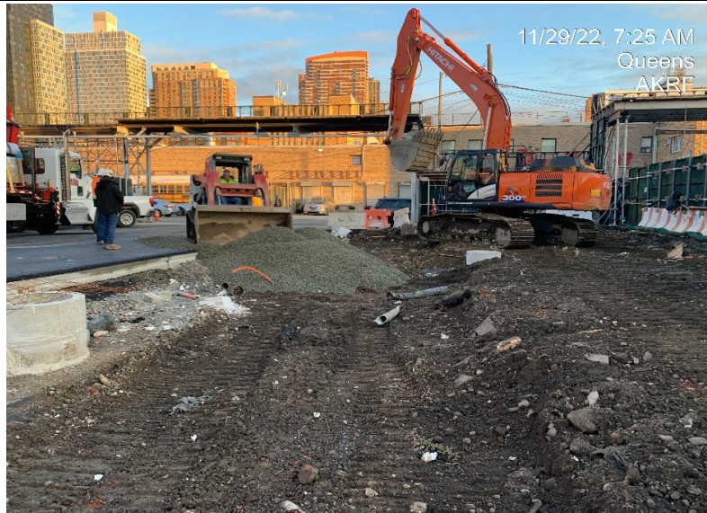
Photograph 2 - The landscaping contractor grading gravel in WC-25, view facing north.
