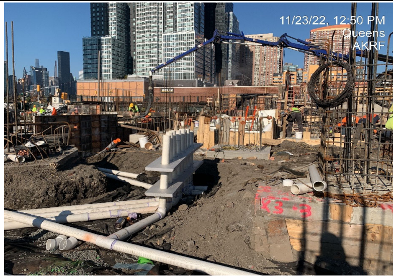
Photograph 1 - Civetta Pouring concrete in WC-03.
