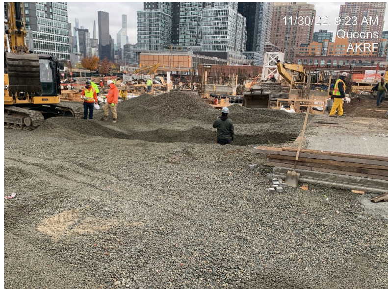
Photograph 2 - The landscaping contractor excavating in WC-18, view facing northwest.
