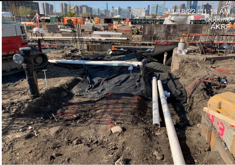
Photograph 1 - Civetta installing SSDS piping in WC-10, view facing west.
