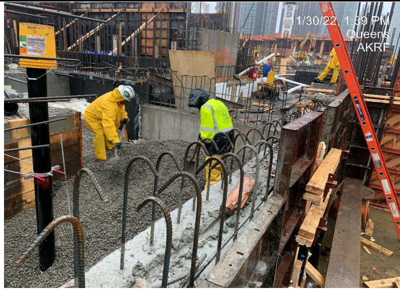
Photograph 1 - Civetta backfilling with gravel WC-02, view facing southeast.
