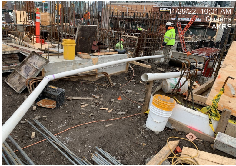
Photograph 1 - Civetta installing SSDS in WC-02, view facing northwest.
