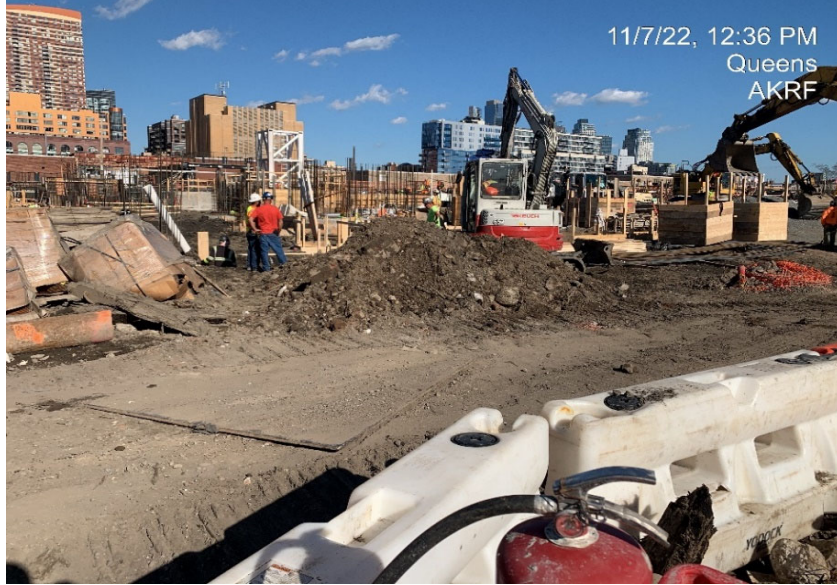
Photograph 1 - Civetta excavating for pile caps in WC-11, view facing northeast.
