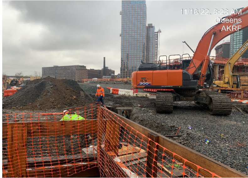
Photograph 1 - The landscaping contractor installing sewer section in WC 17, view facing northeast.
