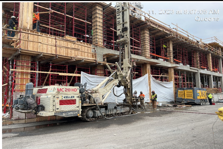
Photograph 3 - CCJV drilling hoist caissons in WC-24, view facing northwest.
