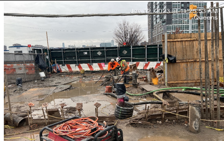
Photograph 3 - CCJV flushing out hoist caissons in WC-01, view facing west.
