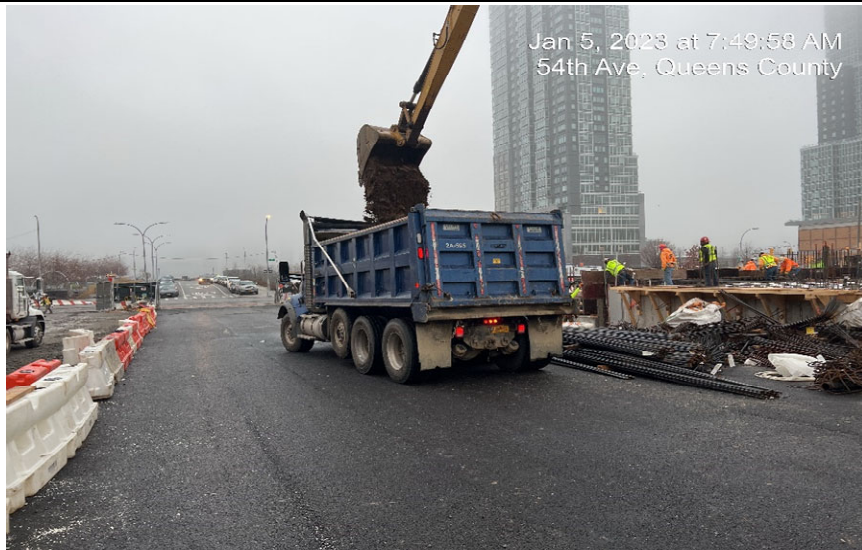
Photograph 1 - Civetta exports one load from WC-11 (0-4') to Bayshore, view facing west.
