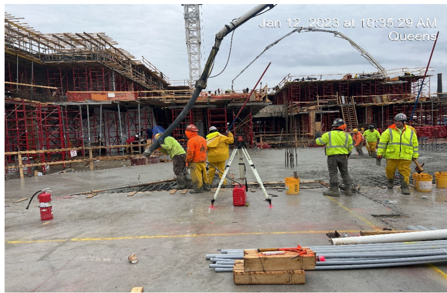
Photograph 2 - CCJV pouring concrete slab in WC-11, view facing east.
