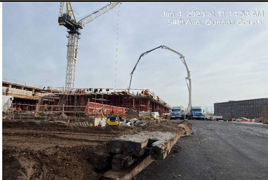
Photograph 3 - CCJV pouring concrete in forms of superstructure, view facing east.
