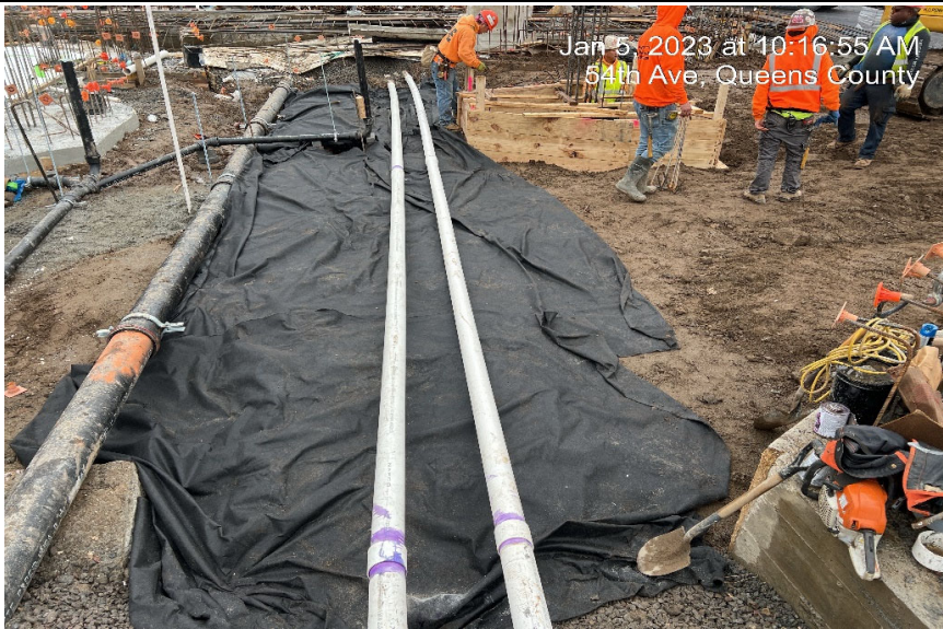
Photograph 2 - CCIJV completes installation of SSDS system in WC-11, view facing east.
