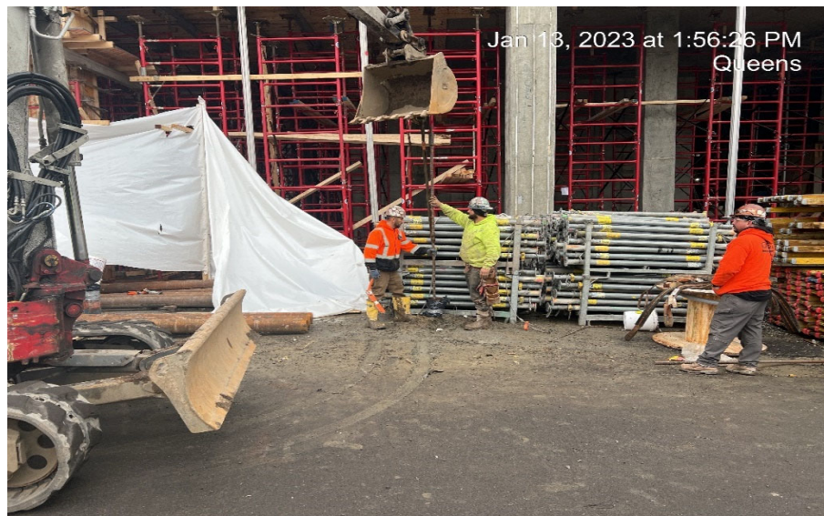
Photograph 3 - CCJV installing rebar in hoist caissons in WC-24, view facing west.
