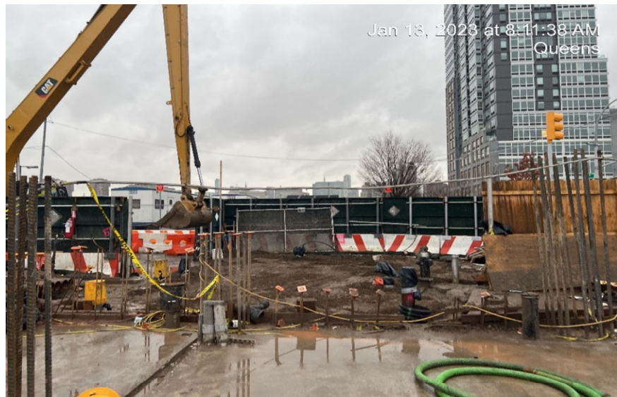
Photograph 2 - CCJV grading soil around hoist caissons in WC-01, view facing west.
