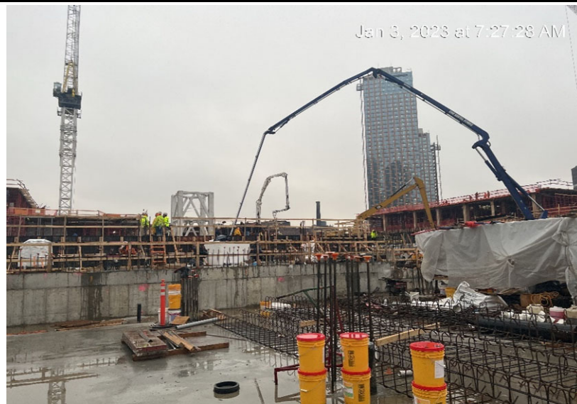
Photograph 2 - CCJV pours concrete slab in sections of WC-11, view facing east.
