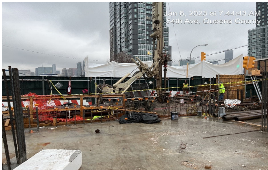
Photograph 3 - CCJV drilling caissons in WC-01, view facing northwest.
