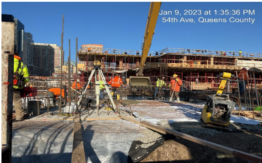
Photograph 2 - CCJV pouring concrete in WC-11, view facing north.
