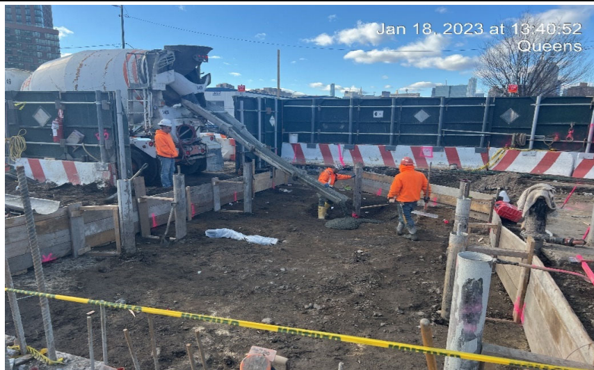
Photograph 3 - CCJV pouring concrete around hoist cassettes in WC-01, view facing east.
