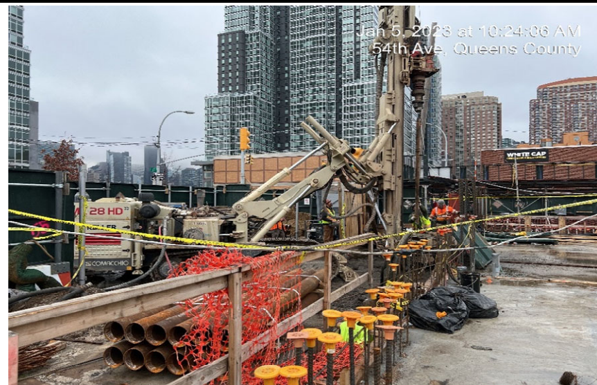
Photograph 3 - CCIJV drilling caissons in WC-01, view facing north.
