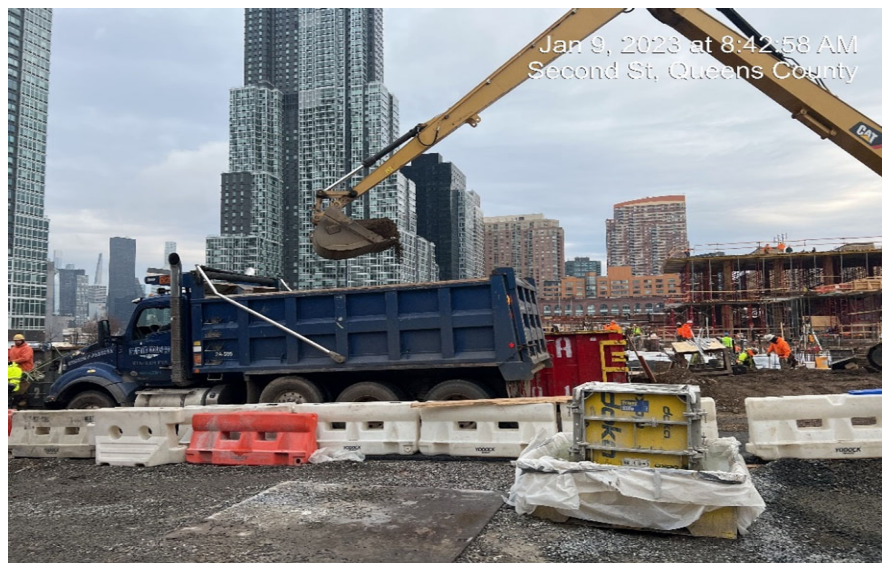
Photograph 3 - CCJV exporting one load from WC-11 (0-4') to Bayshore, view facing north.
