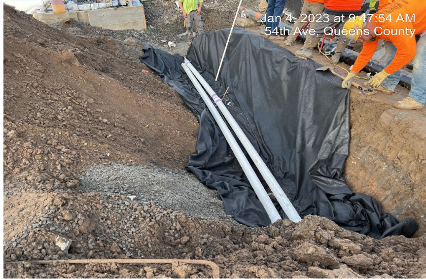
Photograph 1 - Civetta installs SVE system in WC-11, view facing west.
