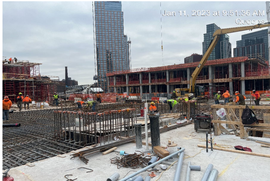
Photograph 2 - CCJV installing rebar in WC-11, view facing southeast.
