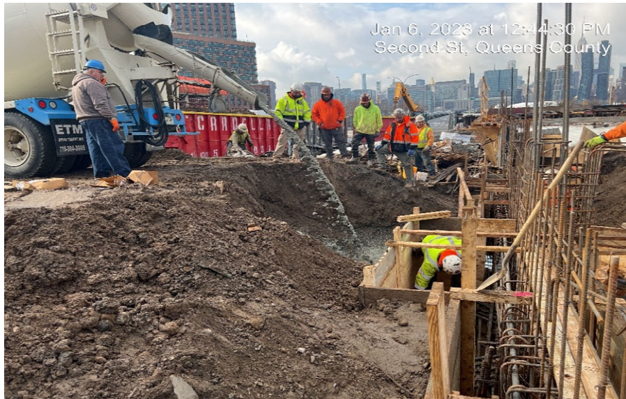
Photograph 2 - CCJV pouring concrete at the footing of WC-11, view facing west.
