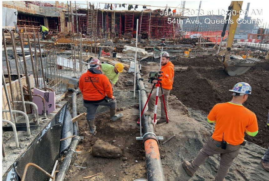
Photograph 2 - CCJV installs SVMP-3 in WC-11, view facing east.
