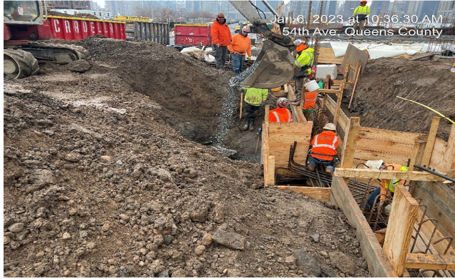
Photograph 1 - Civetta backfills No. 2 stone around pile cap WC-11, view facing west.
