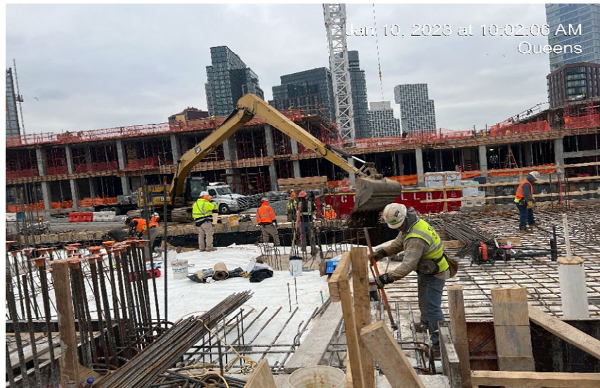
Photograph 2 - CCJV backfilling No. 2 at the footing of WC-11, view facing south.
