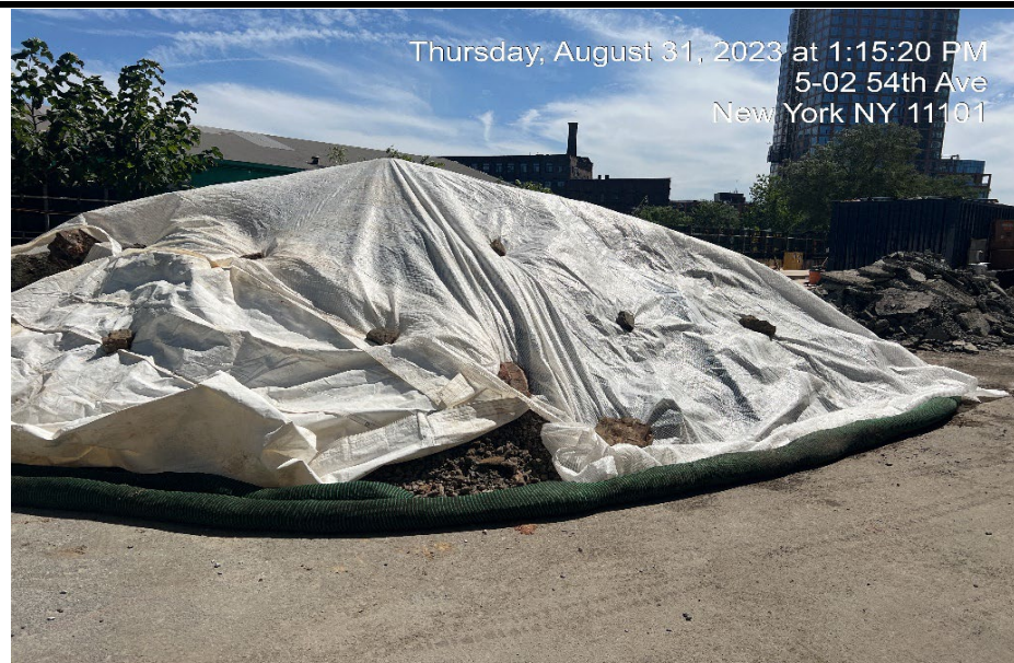
Photograph 3 - Stockpiled soil covered with poly sheeting, view facing southeast.
