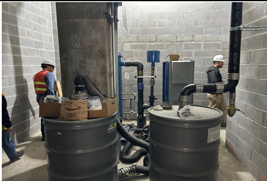
Photograph 3 - AKRF commissioning the SVE system in the new building.
