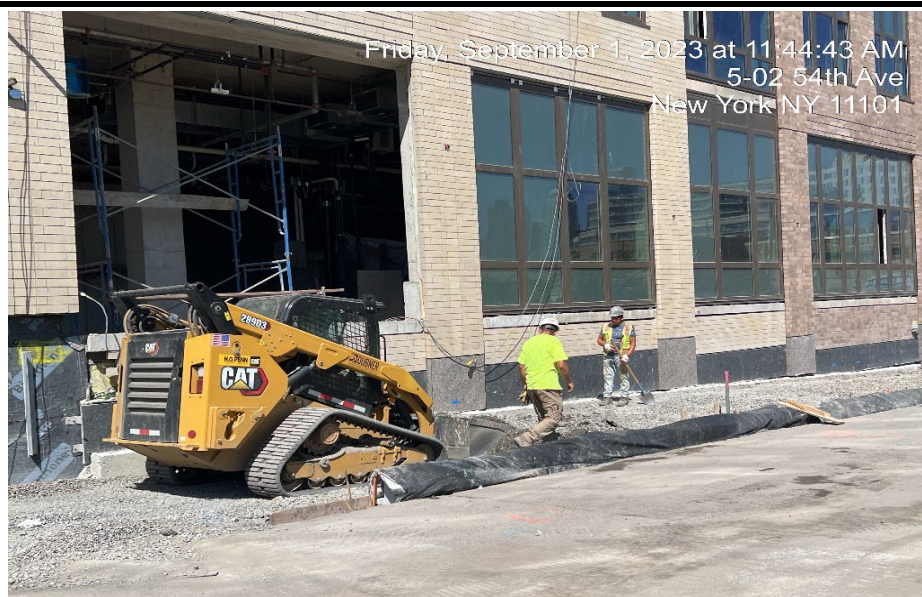
Photograph 3 - Dubner removing excess stone to lower grade in WC- 24, view facing northwest.
