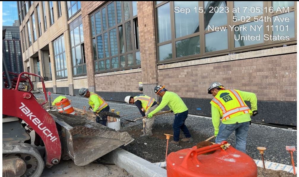
Photograph 1 - Dubner removing gravel for soil compaction test on west side of grid WC- 25, view facing south west.
