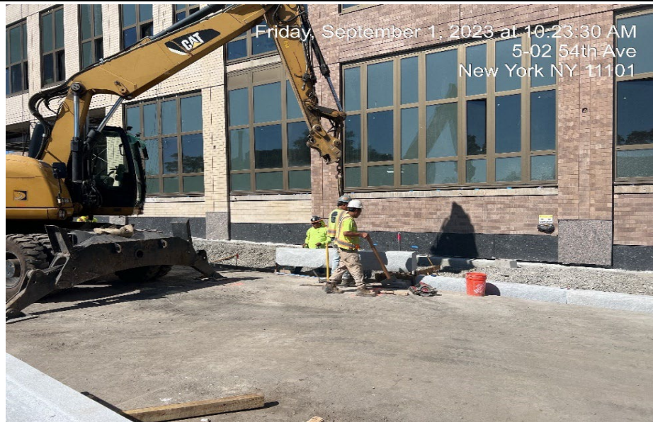
Photograph 1 - Dubner installed stone curbing in WC- 24, facing southwest.
