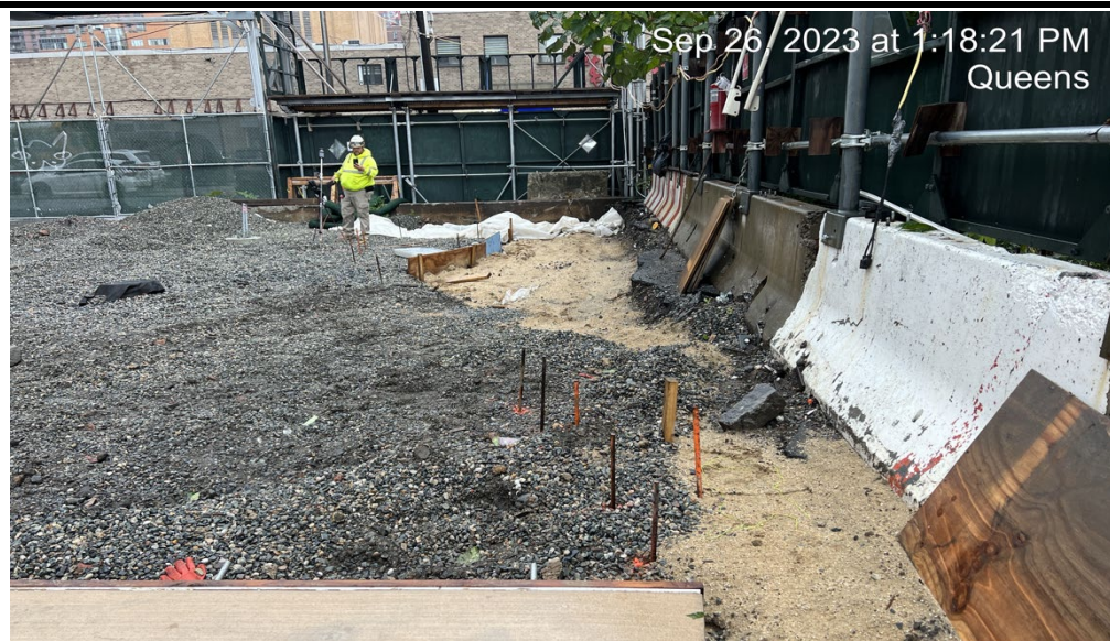
Photograph 3 - Dubner grading with gravel in grid WC- 25, view facing north.
