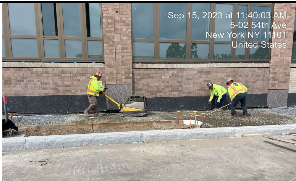
Photograph 3 - Dubner compacting gravel after it was replaced after the soil compaction test for the preparation for concrete, view facing west.
