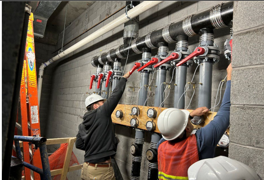
Photograph 1 - Opening the valves on the SSDS eastern manifold.
