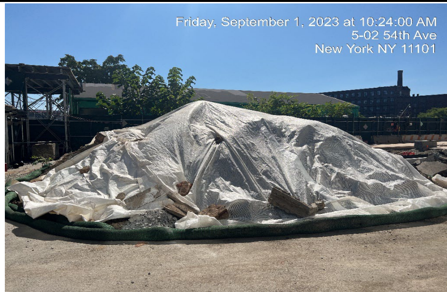
Photograph 2 - Stockpiled soil covered with poly sheeting, view facing east.
