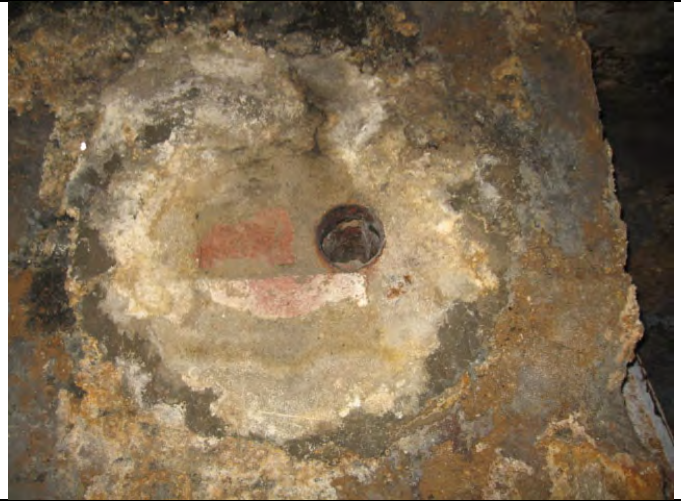
CUT PIPING IN COMMERCIAL BUILDING PARTIAL BASEMENT
