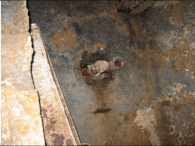
CUT PIPING IN COMMERCIAL BUILDING PARTIAL BASEMENT
