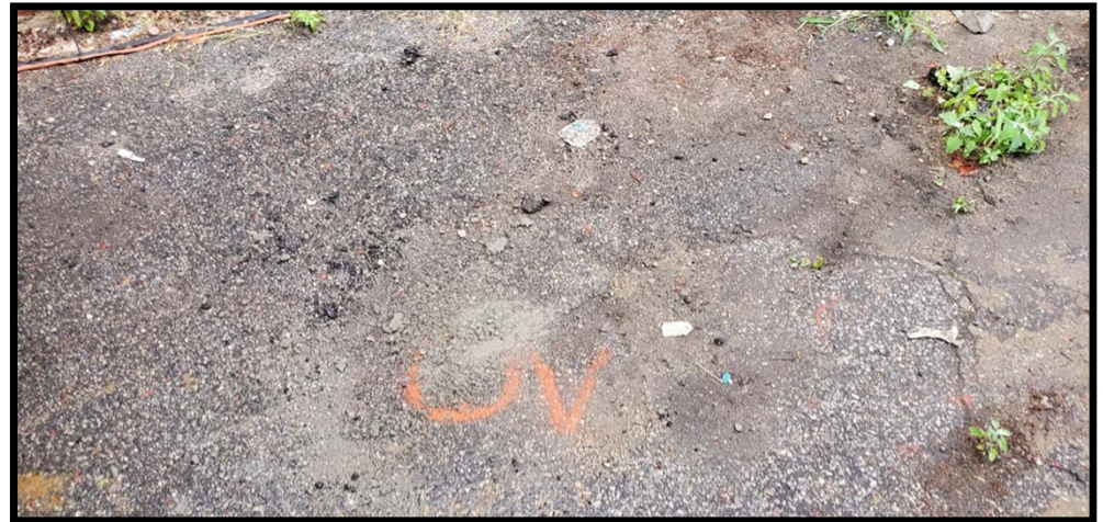
View of a monitoring well properly abandoned and covered with concrete.
