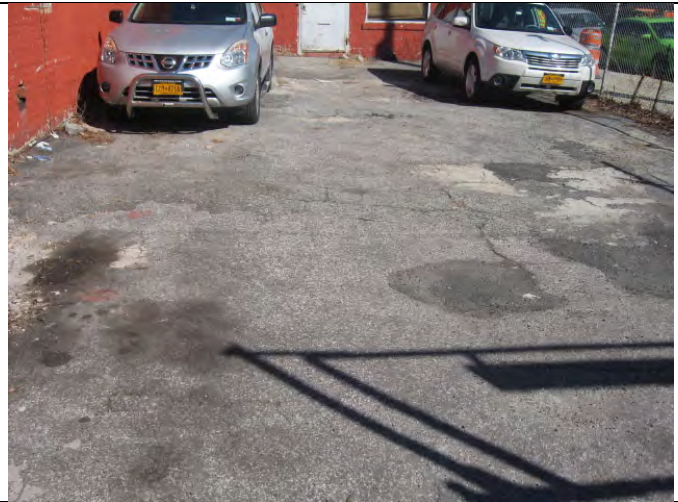
SUBJECT PROPERTY (EASTERN PARKING AREA)
