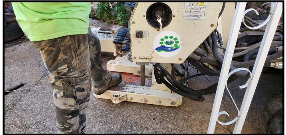
View of a soil boring being advanced.
