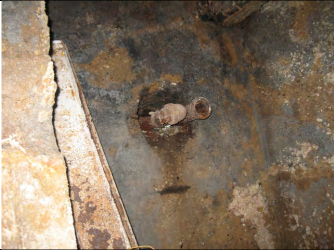
CUT PIPING IN COMMERCIAL BUILDING PARTIAL BASEMENT
