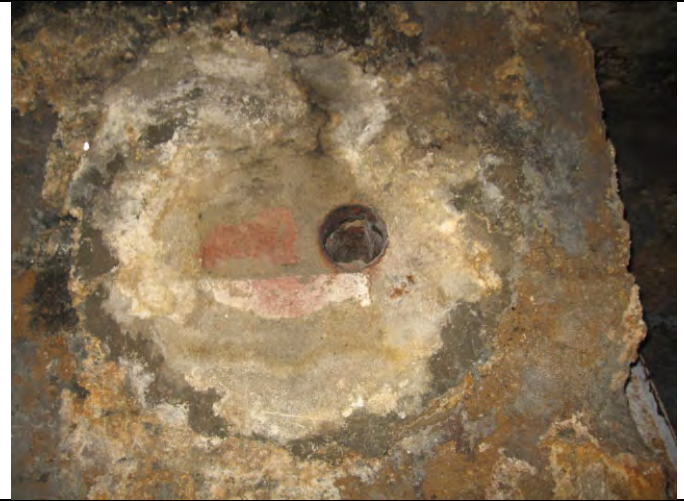
CUT PIPING IN COMMERCIAL BUILDING PARTIAL BASEMENT
