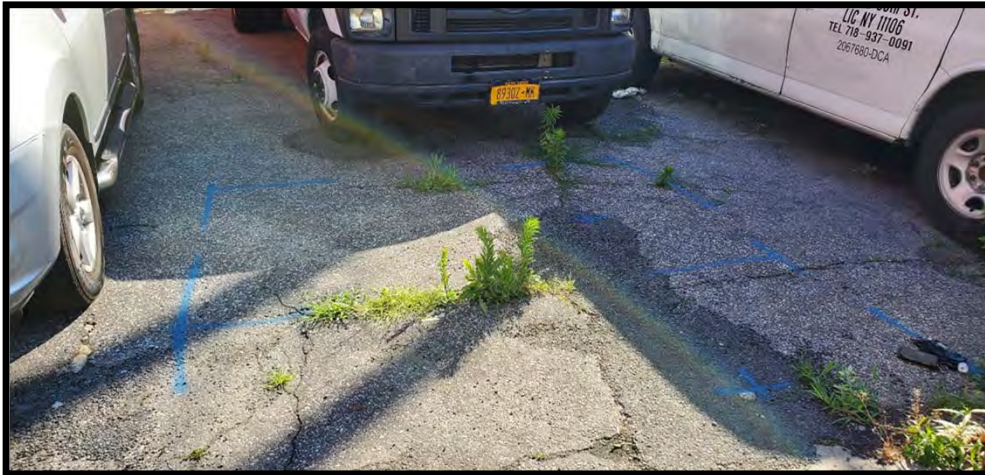
View of a subgrade anomaly marked out during the geophysical survey.
