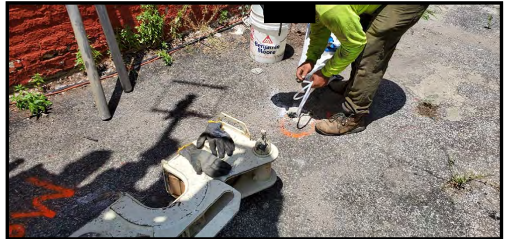
View of a soil vapor sampling point being installed.
