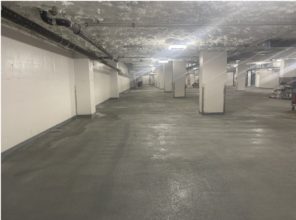
Photograph 4: Facing east, view of Site Cover System intact above the subgrade Track 1 area comprised of concrete building foundation, NYSDEC approved clean stone, and a demarcation layer.
