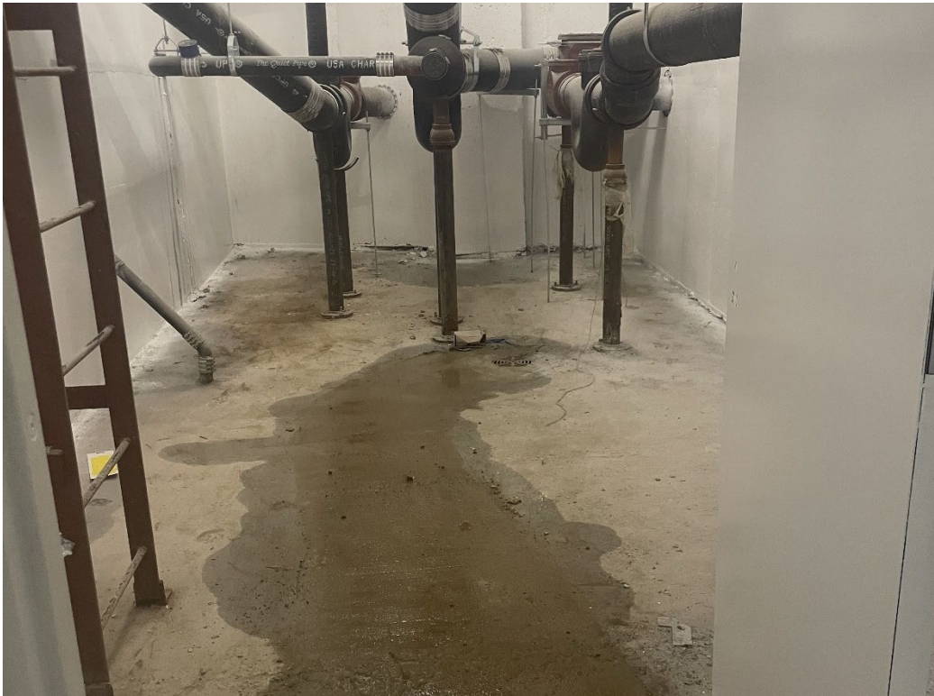
Photograph 6: Facing south, view of basement room with floor drain within the Site Cover System intact above the subgrade Track 1 area comprised of concrete building foundation, NYSDEC approved clean stone, and a demarcation layer.
