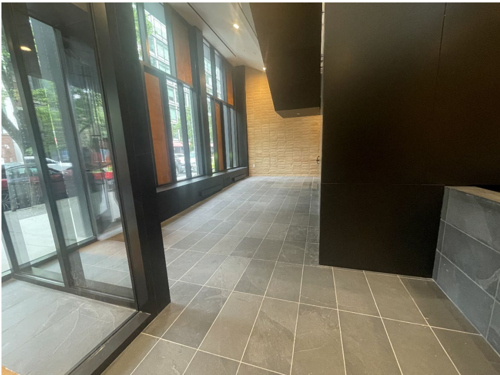
Photograph 8: View of Site Cover System intact above the on-grade Track 4 area comprised of concrete building foundation, NYSDEC approved clean stone, and a demarcation layer.
