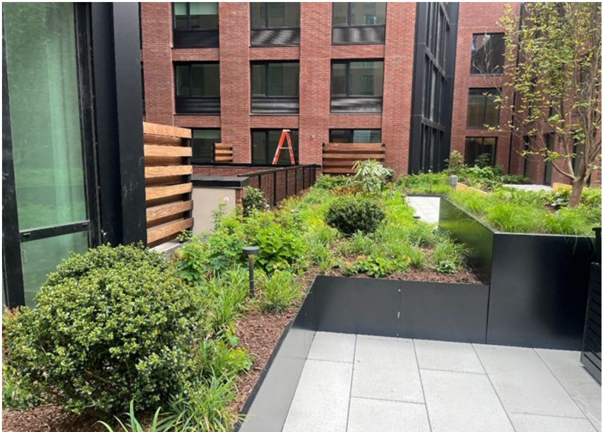
Photograph 10: View of raised planter on the green roof of the building.
