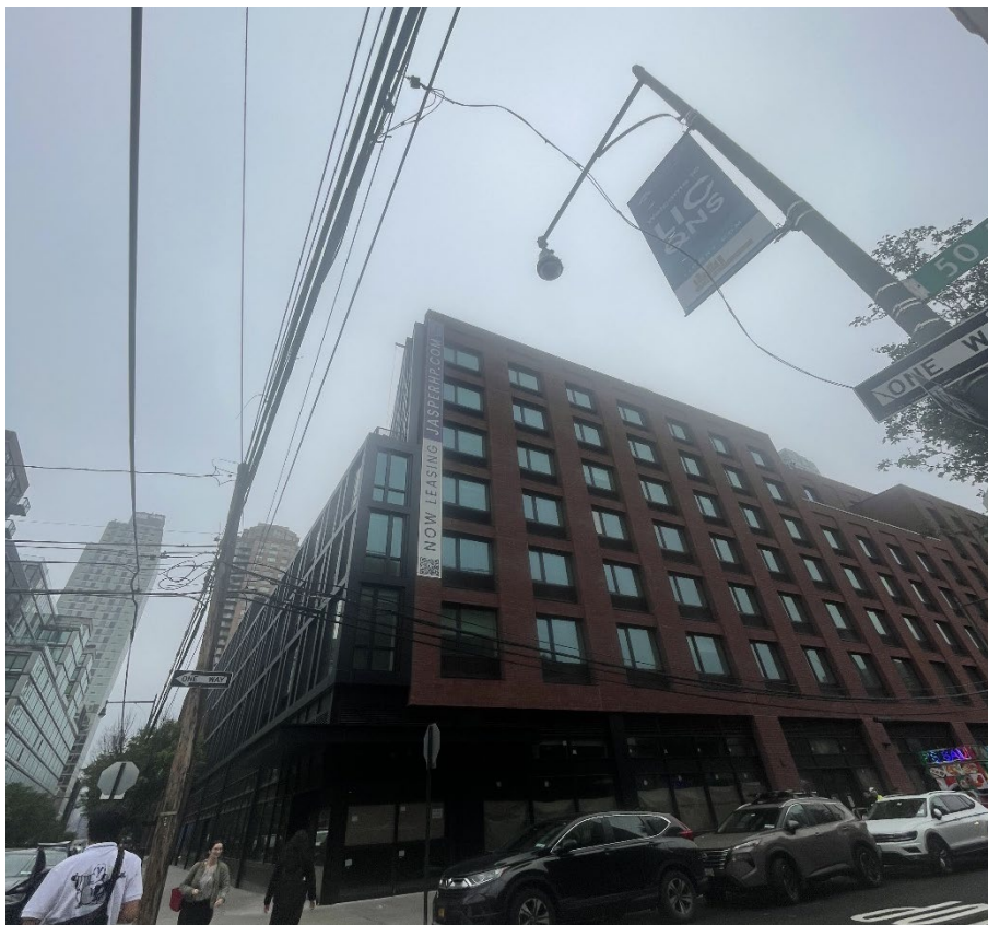
Photograph 1: Facing northwest, view of newly constructed Site building.
