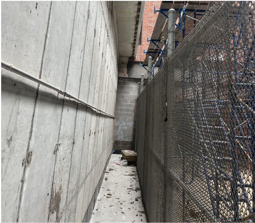
Photograph 9: Facing northeast, view of exposed building footing above Track 4 area to be waterproofed, insulated, and topped with a concrete slab.
