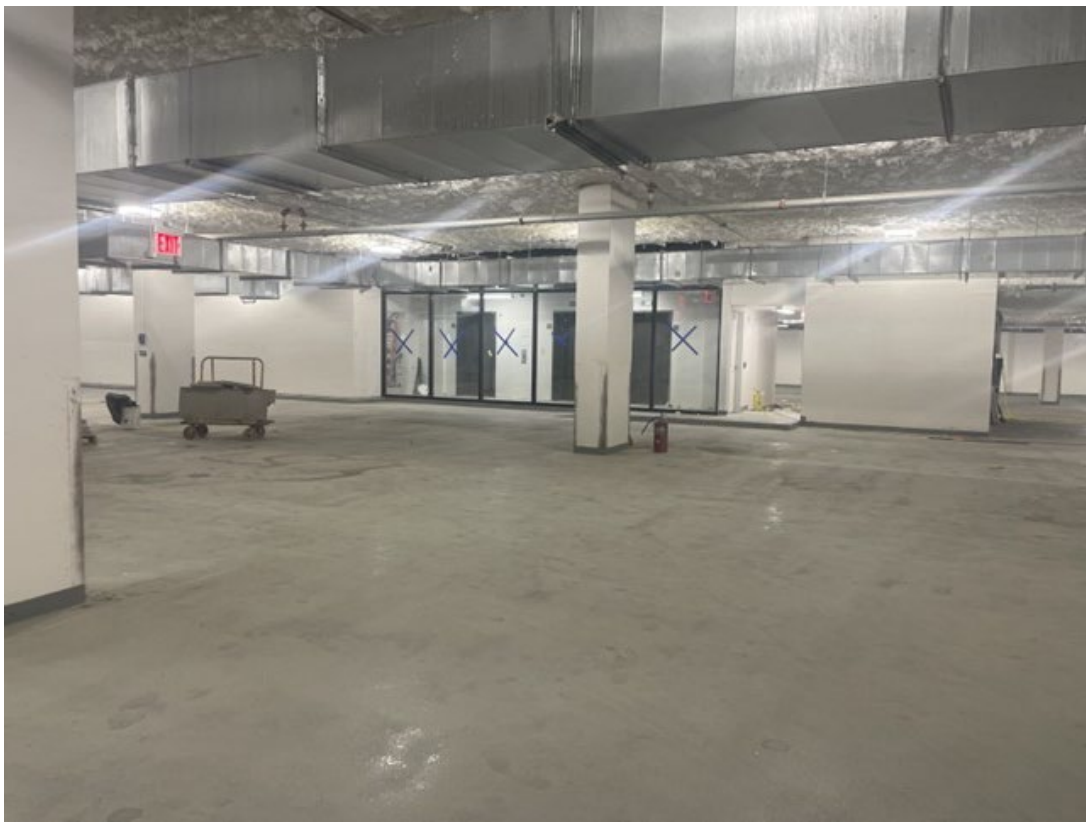
Photograph 5: Facing north, view of Site Cover System intact above the subgrade Track 1 area comprised of concrete building foundation, NYSDEC approved clean stone, and a demarcation layer.
