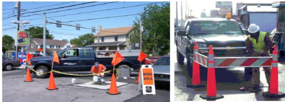
Figures A1.2.2(a)(b)(c) - Examples of Level 2 Traffic Control
