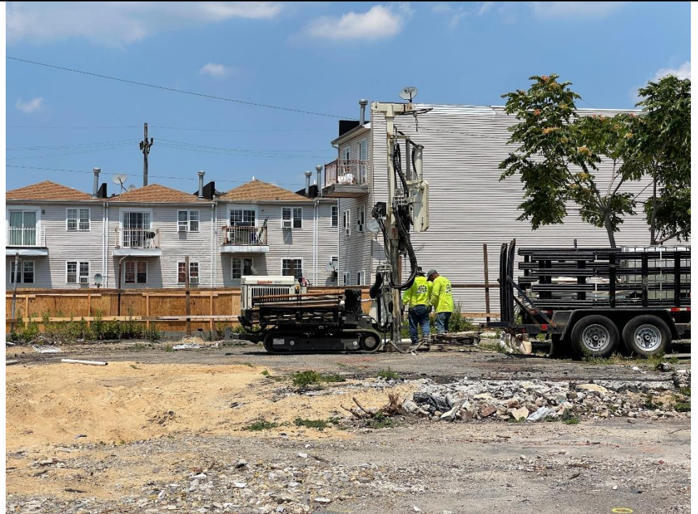
Photo 1 – Photo of typical well abandonment activities
