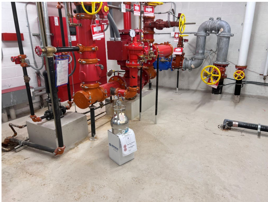
Photograph No. 6: View of IA-5 located in the southeastern portion of the building.
