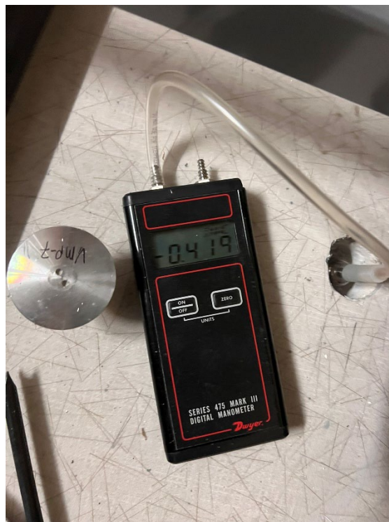
Photograph No. 11: Representative view of differential pressure readings at existing VMPs (e.g. VMP-7).
