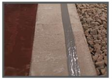
At a Location Designated by the Design Team: Seal Drago Wrap to concrete with DragoTack Tape.
