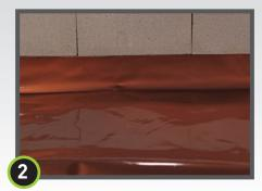
Press Drago Wrap firmly against the applied Drago Mastic on the foundation wall.
