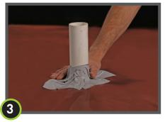
If Drago Wrap is close to pipe and void space is minimized then seal around pipe penetration with either DragoSeal Tape (as shown), Drago Tape, Drago Mastic or Drago Sealant and Drago Sealant Form.
