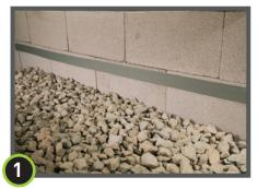
Remove the release liner on one side of DragoTack Tape and adhere to foundation wall at the height of the slab or at impediments.
