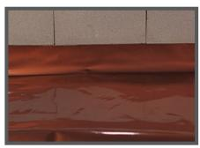
Note: Turn Drago Wrap up foundation walls or forms. Ensure Drago Wrap is flush against the corner to avoid tenting.
