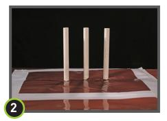
Place a detail patch over and around the base of the pipe penetrations as closely as possible, ensuring that it is flush with the base of the penetrations. Seal all sides of the detail patch with DragoSeal Tape.
