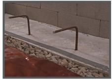
Onto a Perimeter Footing at Impediments: Seal Drago Wrap to concrete with DragoTack Tape.
