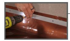
**MECHANICAL SEAL OPTION:** If a mechanical seal is needed, fasten a termination bar over the top of the Drago Wrap inline with the DragoTack Tape.
