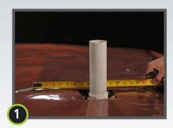
Cut a detail patch to a size and shape that creates a 6" overlap on all edges around the void space at the base of the pipe.
