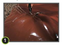
Install Drago Wrap around pipe penetrations by slitting/cutting material as needed. Try to minimize the void space created.
