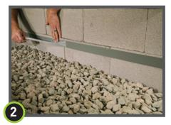
When ready to apply Drago Wrap, remove the exposed release liner from DragoTack Tape.
