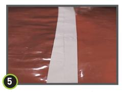
Seal the seams with DragoSeal Tape. Note: Remove the release liner on one side of DragoSeal Tape prior to application. Apply pressure to DragoSeal Tape after application.
