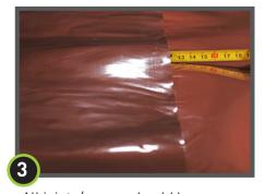
All joints/seams should be overlapped a minimum of 12 inches.
