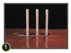
Cut a slit the size to accommodate the width of the multiple pipes. Try to minimize the void space created.
