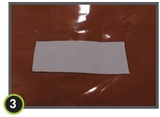
Center DragoSeal Tape over small hole or slice in Drago Wrap. Apply pressure to DragoSeal Tape after application.
