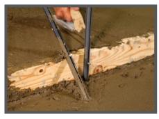
Beast Form Stake is strong enough to withstand a beating during concrete placement while holding its shape. It is easy to remove and reusable for the next job.
