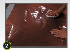
Measure and cut a piece of Drago Wrap to cover damaged area 6" in all directions. Clean area of adhesion.
