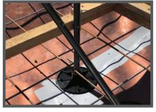
This concrete form stake takes the place of traditional nail stakes for interior forming applications, utilizing SpeedTrack™ Fastening Grooves for unlimited fastener placement.
