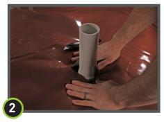
Pull material over and flatten. Clean area of adhesion where Drago accessory will be applied.
