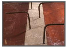
Onto Interior Grade Beams at Impediments: Seal Drago Wrap to concrete with DragoTack Tape.
