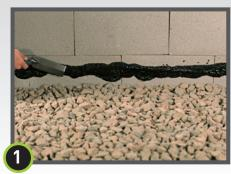
Apply Drago Mastic to the foundation wall at the anticipated edge of the subsequently applied Drago Wrap at the height of the slab or impediments.
