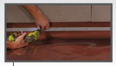
**MECHANICAL SEAL OPTION:** If a mechanical seal is needed, fasten a termination bar over the top of the Drago Wrap inline with the DragoTack Tape.
