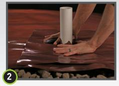
Cut an "X" the size of the pipe diameter in the center of the detail patch and slide tightly over pipe.
