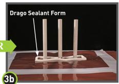
Install Drago Sealant Form continuously to Drago Wrap and around the entire perimeter of the group of penetrations and at least 1 inch beyond the terminating edge of Drago Wrap.
