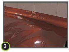
Press Drago Wrap firmly against DragoTack Tape to secure.
