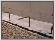
Onto a Perimeter Footing at Impediments: Seal Drago Wrap to concrete with Drago Mastic.
