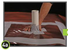
Seal around the base of the pipe using DragoSeal Tape (as shown) or Drago Tape.
