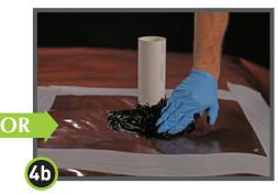
Seal around the base of the pipe with Drago Mastic. Note: apply using disposable glove, paint brush, or similar.
