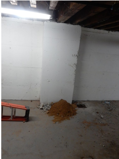
13. Typical suction pit construction at cellar
