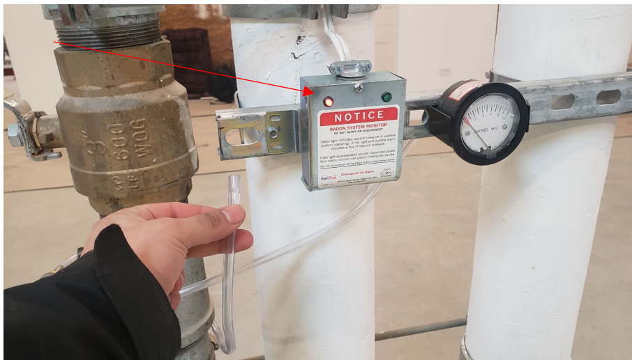
17. Typical visual gauge and audible alarm installation at RP-1 and RP-2 (note green light indication normal operation)
