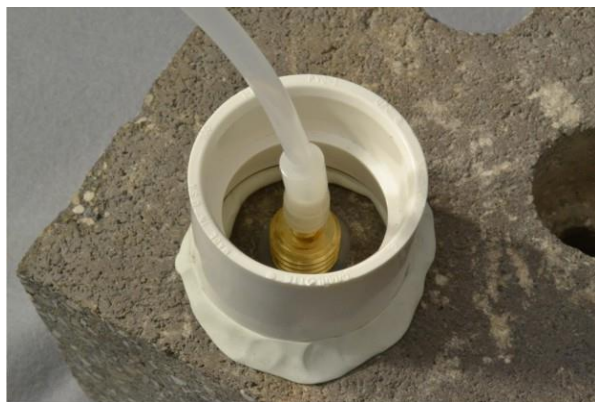
Figure 6. Water dam used for leak detection
