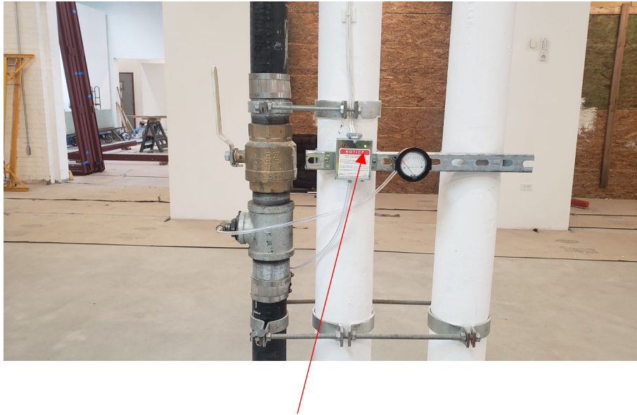
17. Typical visual gauge and audible alarm installation at RP-1 and RP-2 (note green light indication normal operation)
